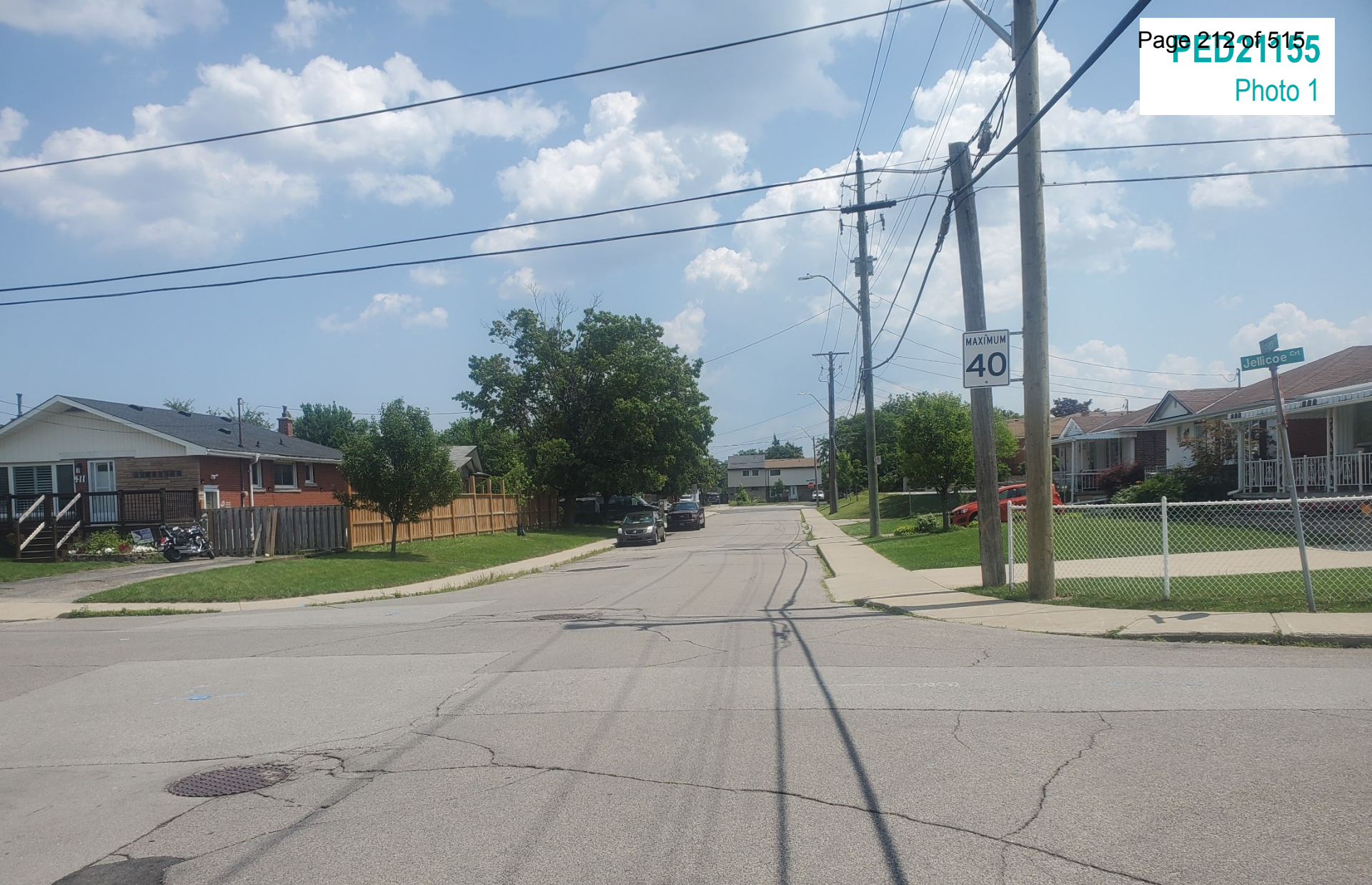
Subject Property looking east towards Upper Wentworth Street at Jellicoe Court
