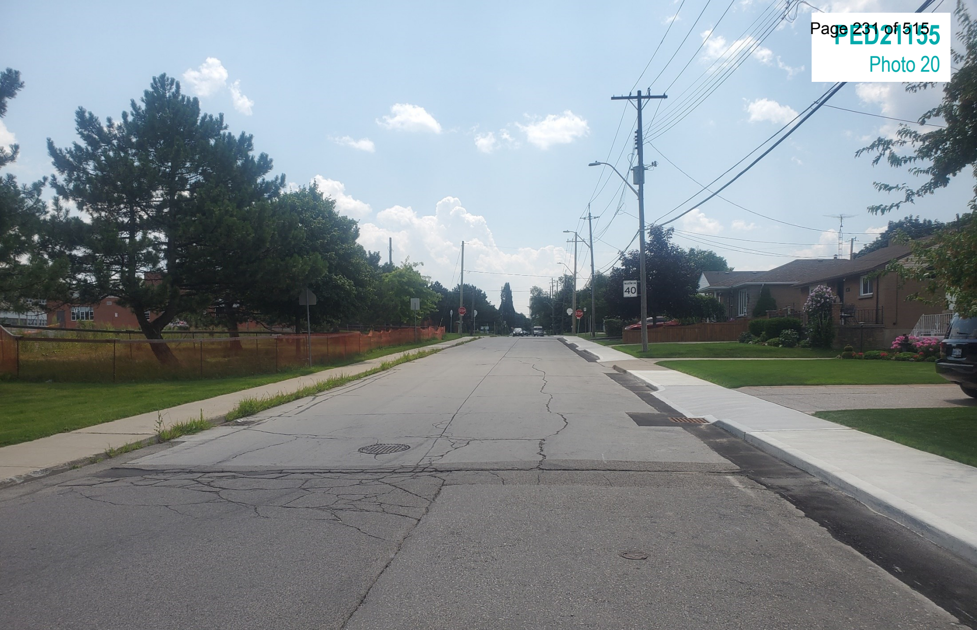
East 16th Street looking south
