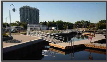
Pier 7 Shorewall, Boardwalk & Boat Slips
