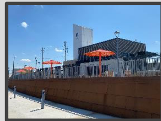
Pier 8 Sanitary Pumping Station Infrastructure
