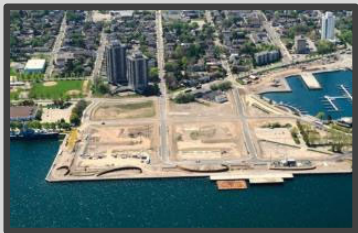
Pier 8 Servicing (Underground & Road) Infrastructure
