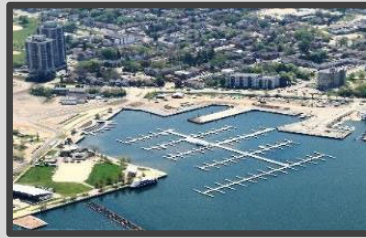
Main Basin Marina & Breakwater Infrastructure Renewal
