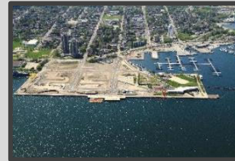
Pier 8 Shorewall Infrastructure Rehabilitation & Renewal
