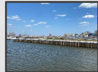
Pier 6&7 Shorewall Rehabilitation, Fish Habitat & Public Boardwalk
