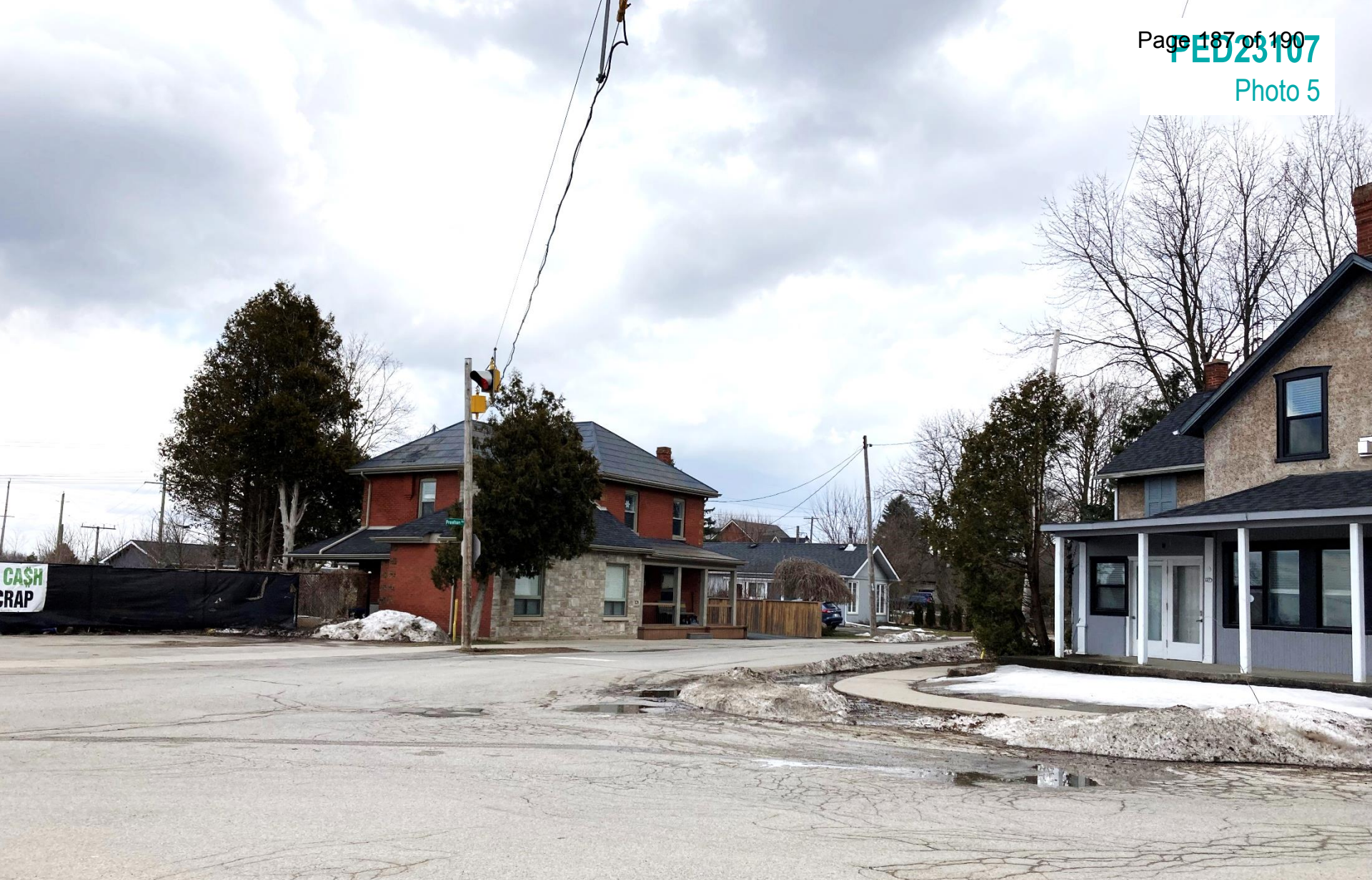
Looking south-east from the intersection of Freilton Road and Brock Road
