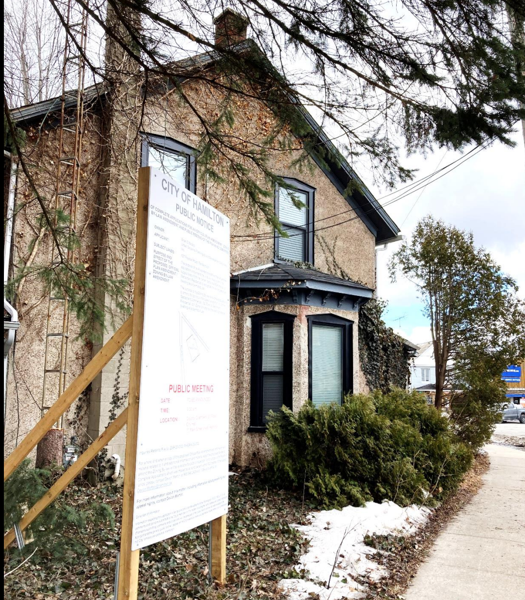
East facade of the subject property looking north on Freelon Road
