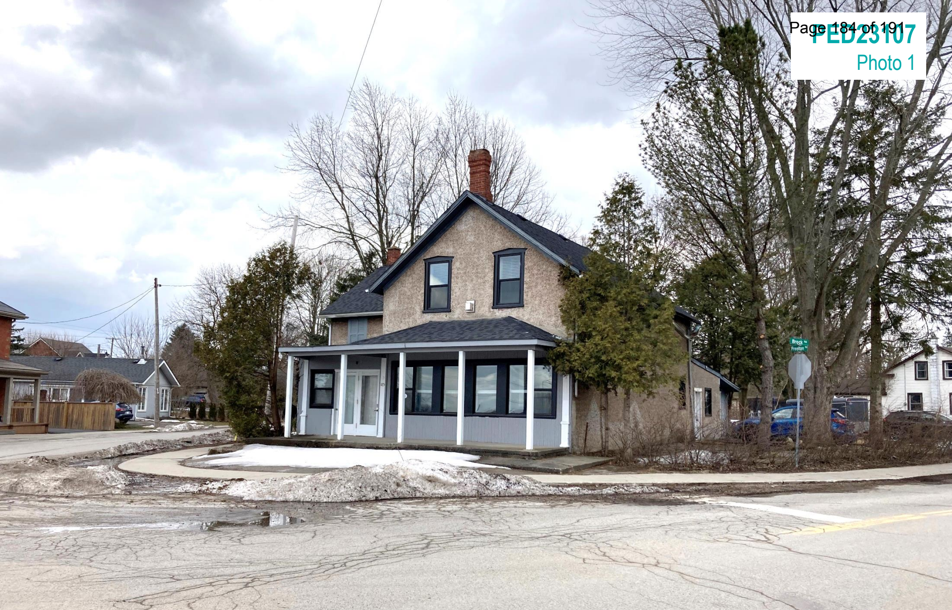
Subject lands looking south from the intersection of Freelon Road and Brock Road
