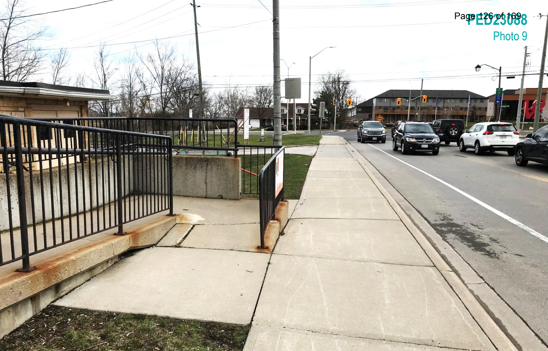
Sidewalk connection along Trinity Church Road between the two properties
