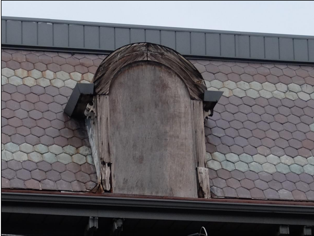
Image 7: Dormer window within Mansard roof (November 2022)
