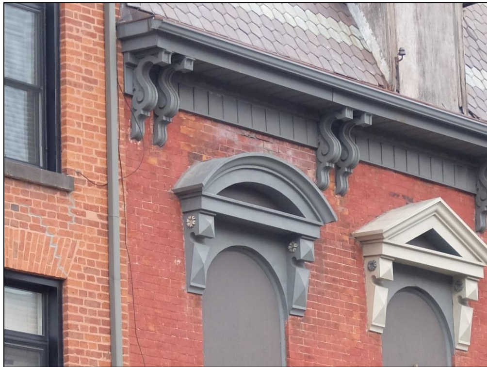
Image 10: Paired brackets on second storey (November 2022)
