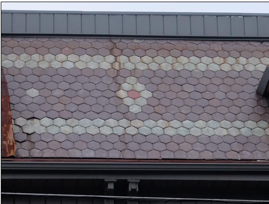
Image 6: Details of polychromatic hexagonal slate tiles (November 2022)
