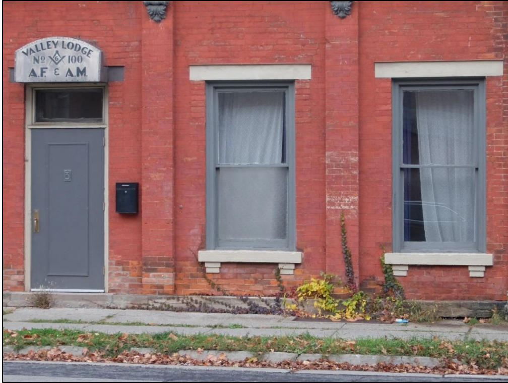
Image 13: First-storey windows with stone sills (November 2022)
