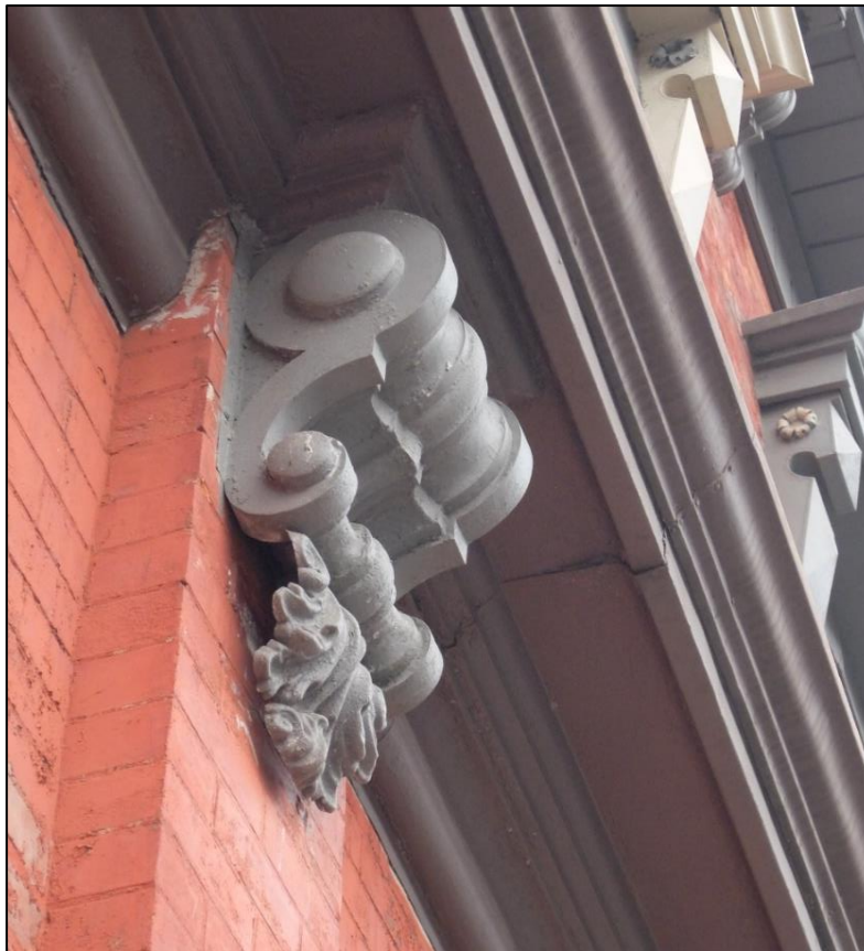
Image 12: Close-up of first-storey bracketed eaves (November 2022)
