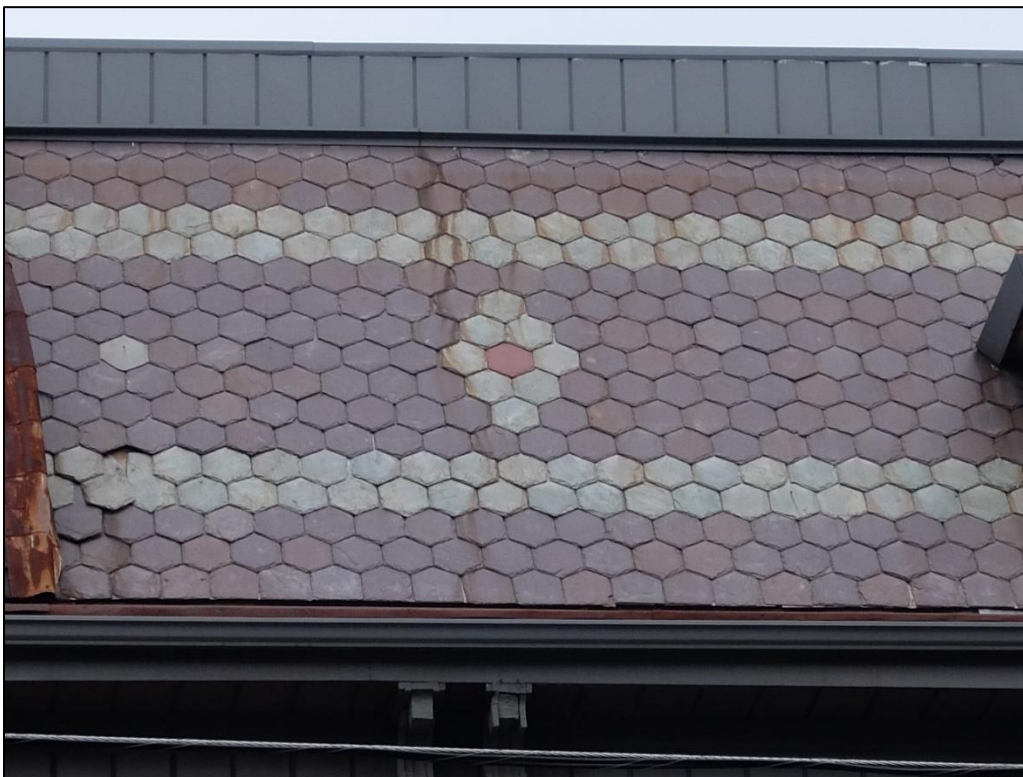
Image 6: Details of polychromatic hexagonal slate tiles (November 2022)
