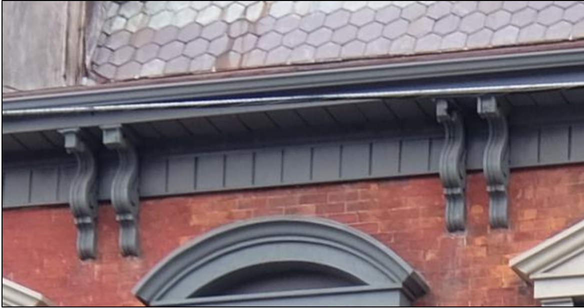
Image 11: Close-up of paired brackets (November 2022)
