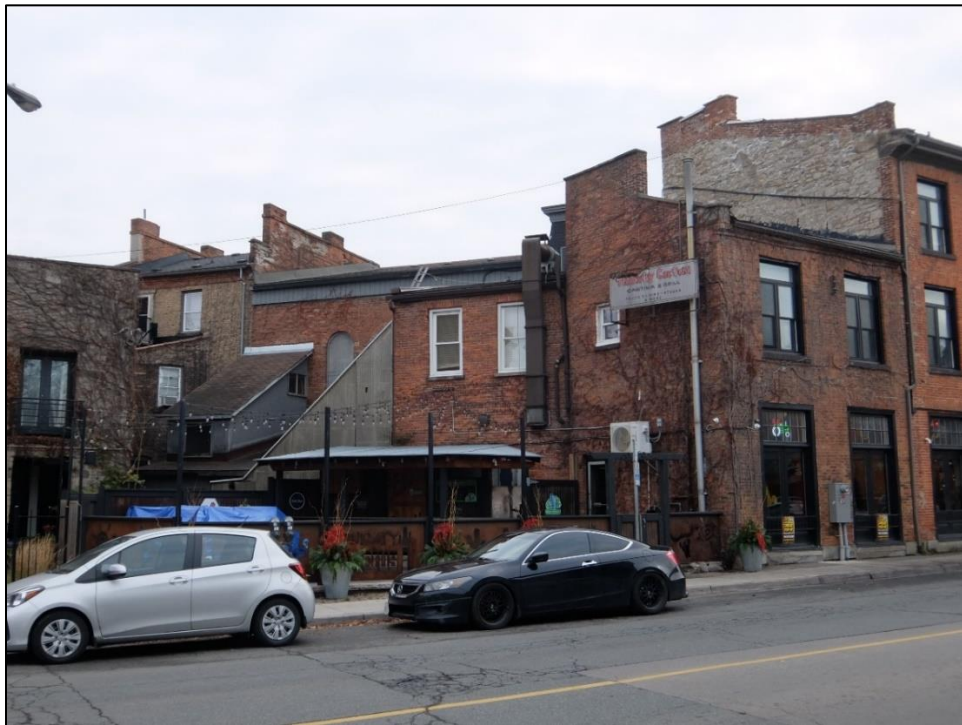
Image 4: Eastern elevation (November 2022)
