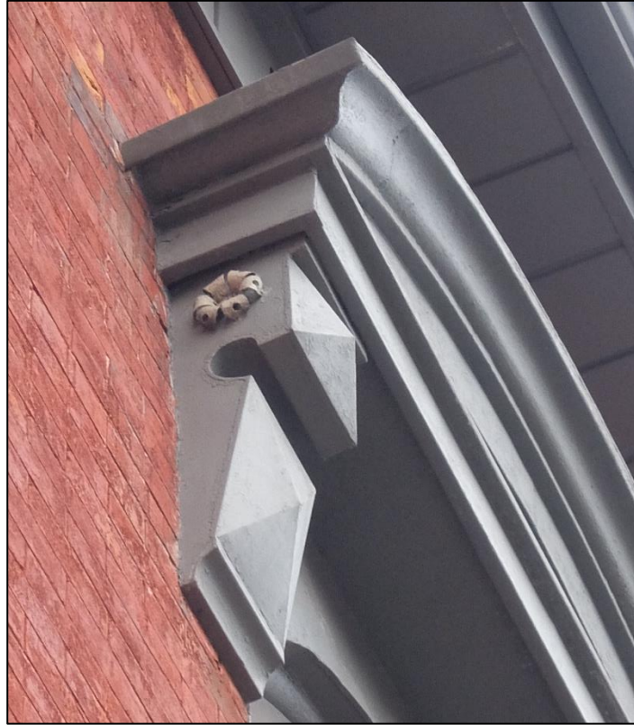
Image 9: Close-up of second-storey window detailing (November 2022)
