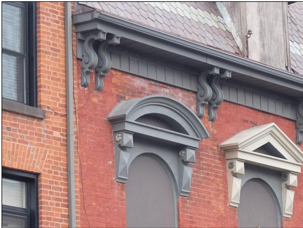
Image 10: Paired brackets on second storey (November 2022)
