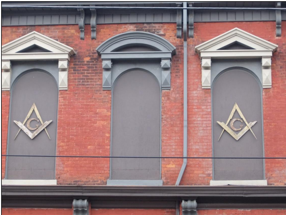
Image 8: Second-storey windows with galvanized iron window hoods (November 2022)
