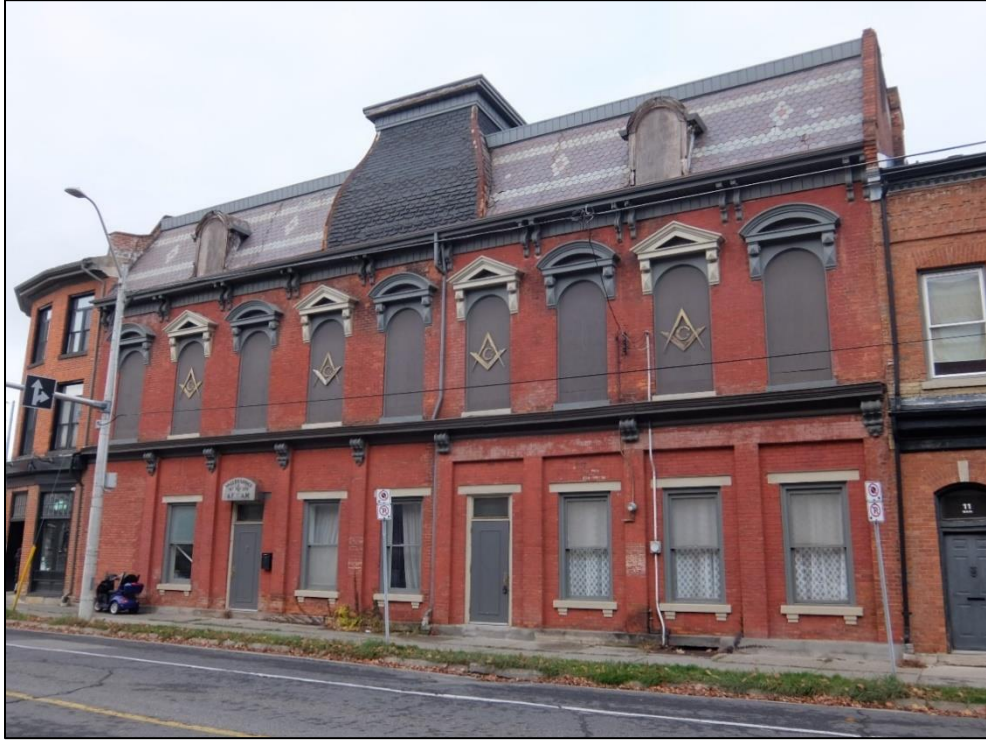
Image 3: Western elevation (November 2022)
