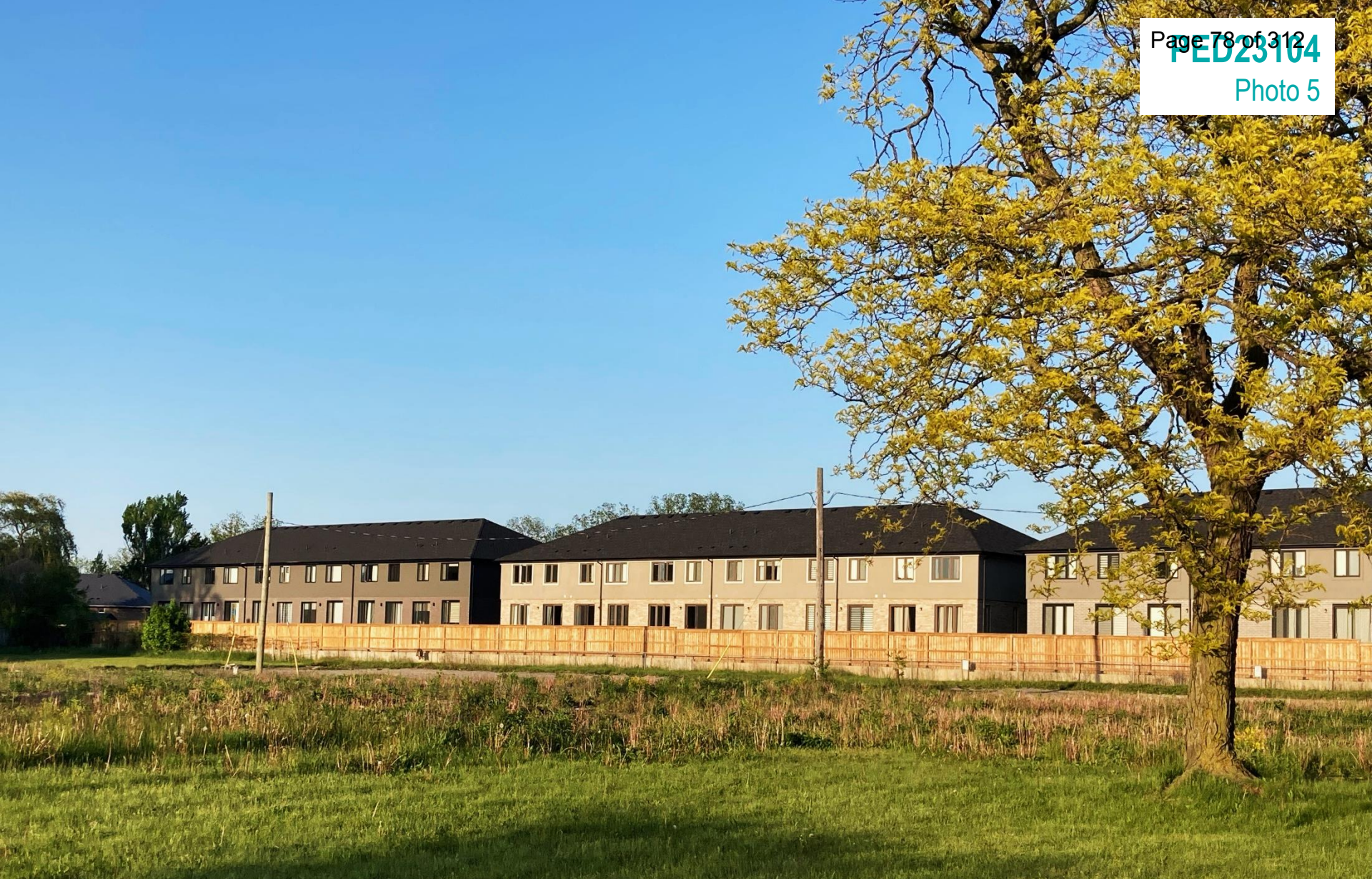
East side of the Subject Lands
