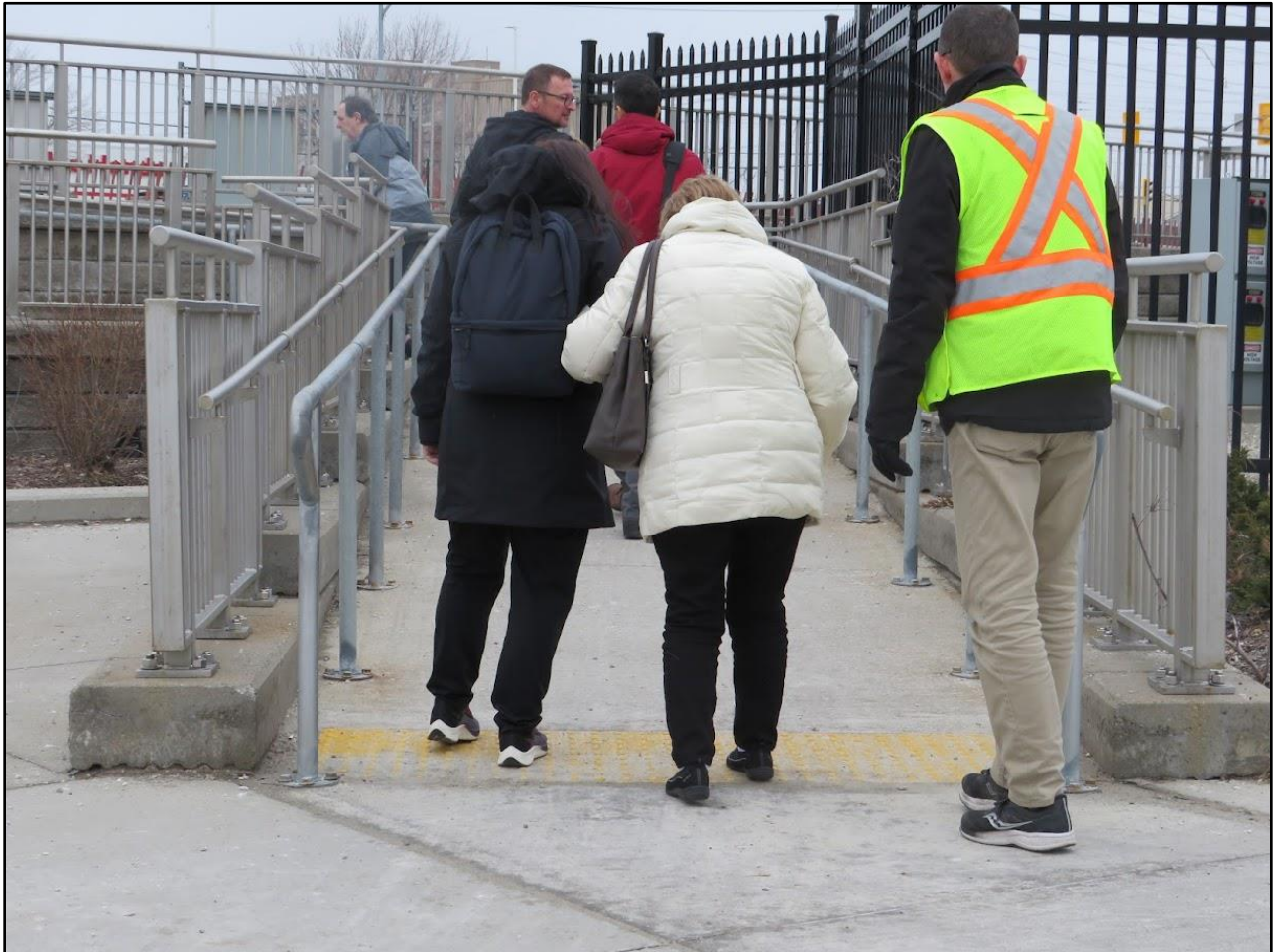
Figure 32: Access ramp up to platform. Numerous landings and lots of button plates to cross.
