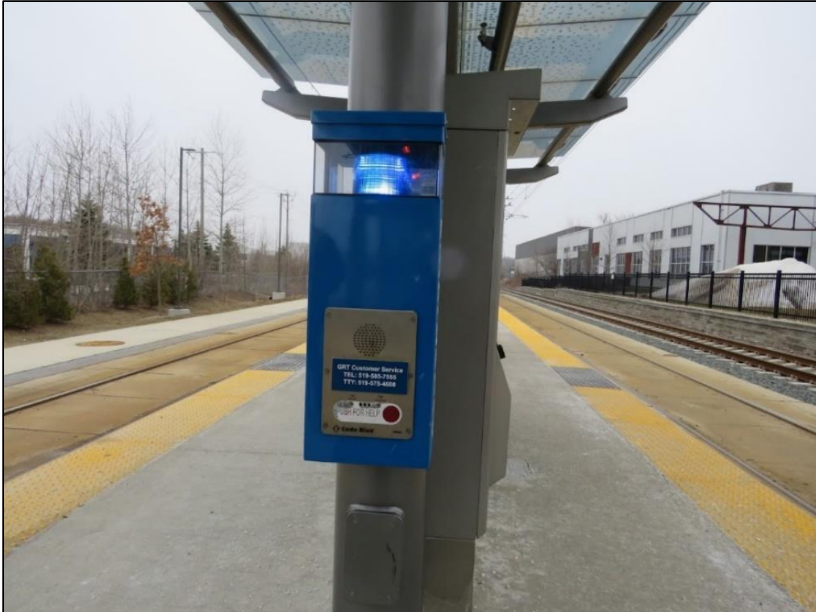
Figure 4: Image of Emergency Beacon at the station. When the button is pressed, all cameras are focused on the platform and emergency services are put on alert. *This is a good example of colour being used as contrast.
