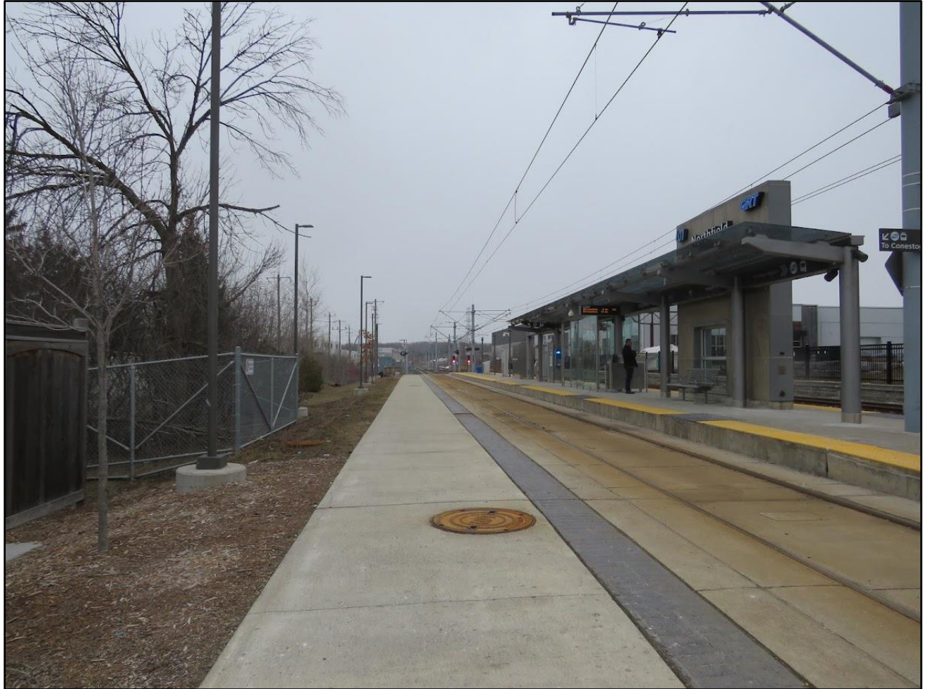
Figure 6: Image of area across from the LRT station platform emergency pedestrian pathway opposite station
