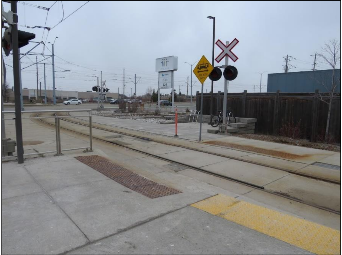
Figure 14: Rail crossing to platform
