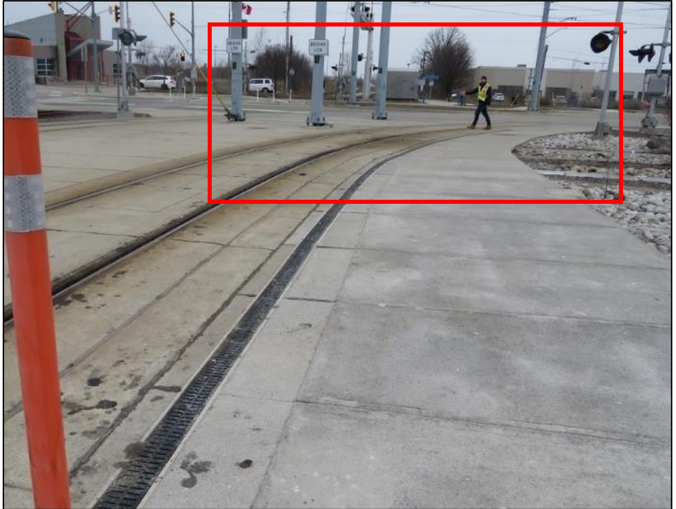
Figure 12: Host demonstrating the difficulty of crossing the intersection in this configuration.
