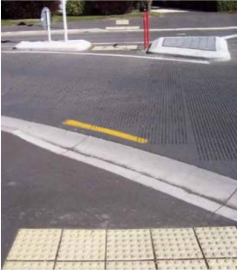
Figure 3: Tactile Ground Surface indicator alignment with crosswalk (Image credit: New Zealand Transportation Authority)
