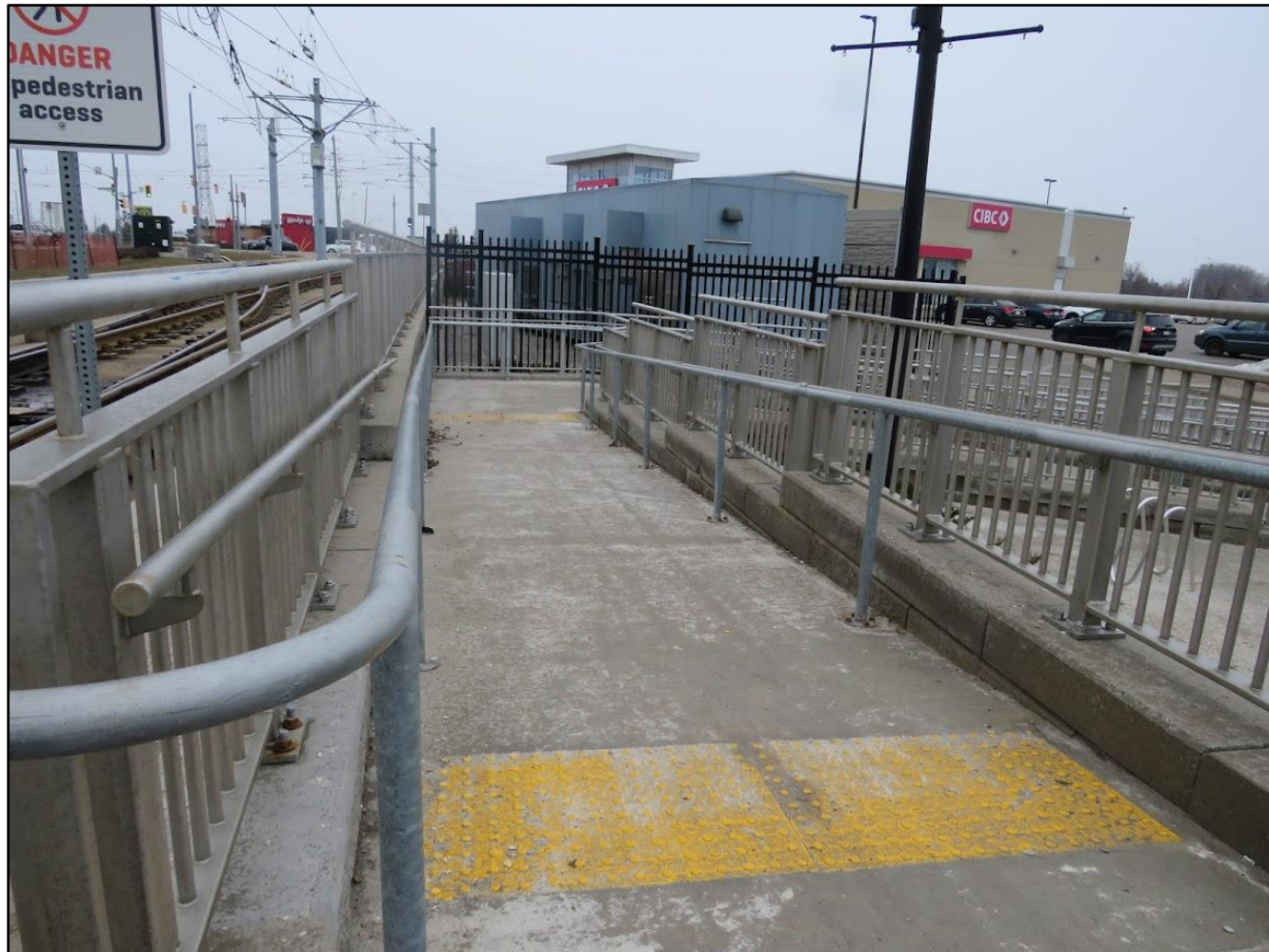
Figure 37: Top of the ramp leaving Conestoga LRT Station
