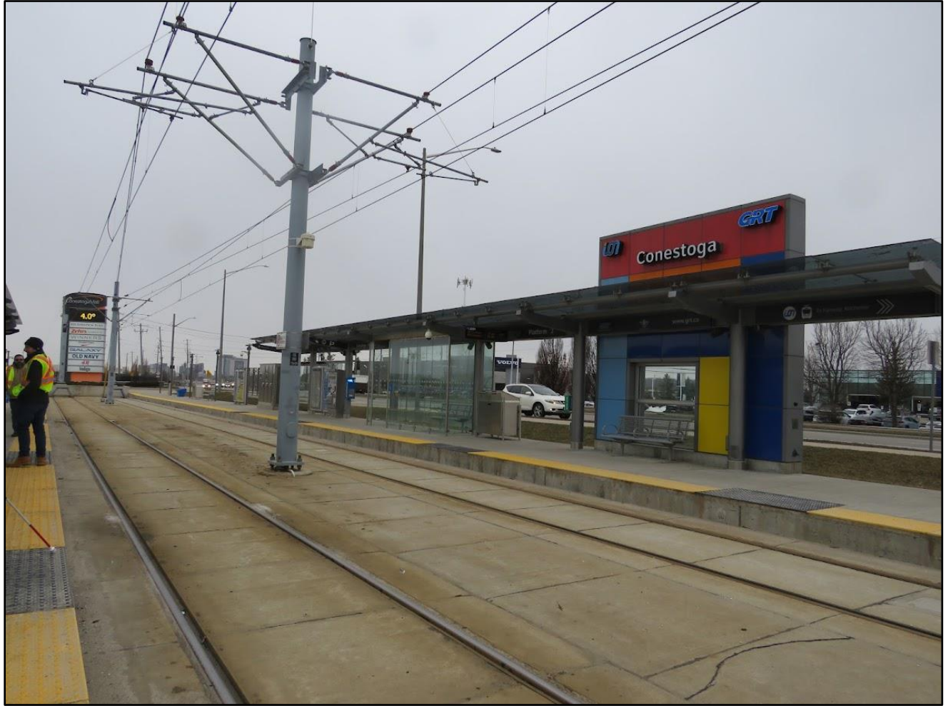
Figure 28: View of the opposite platform.
