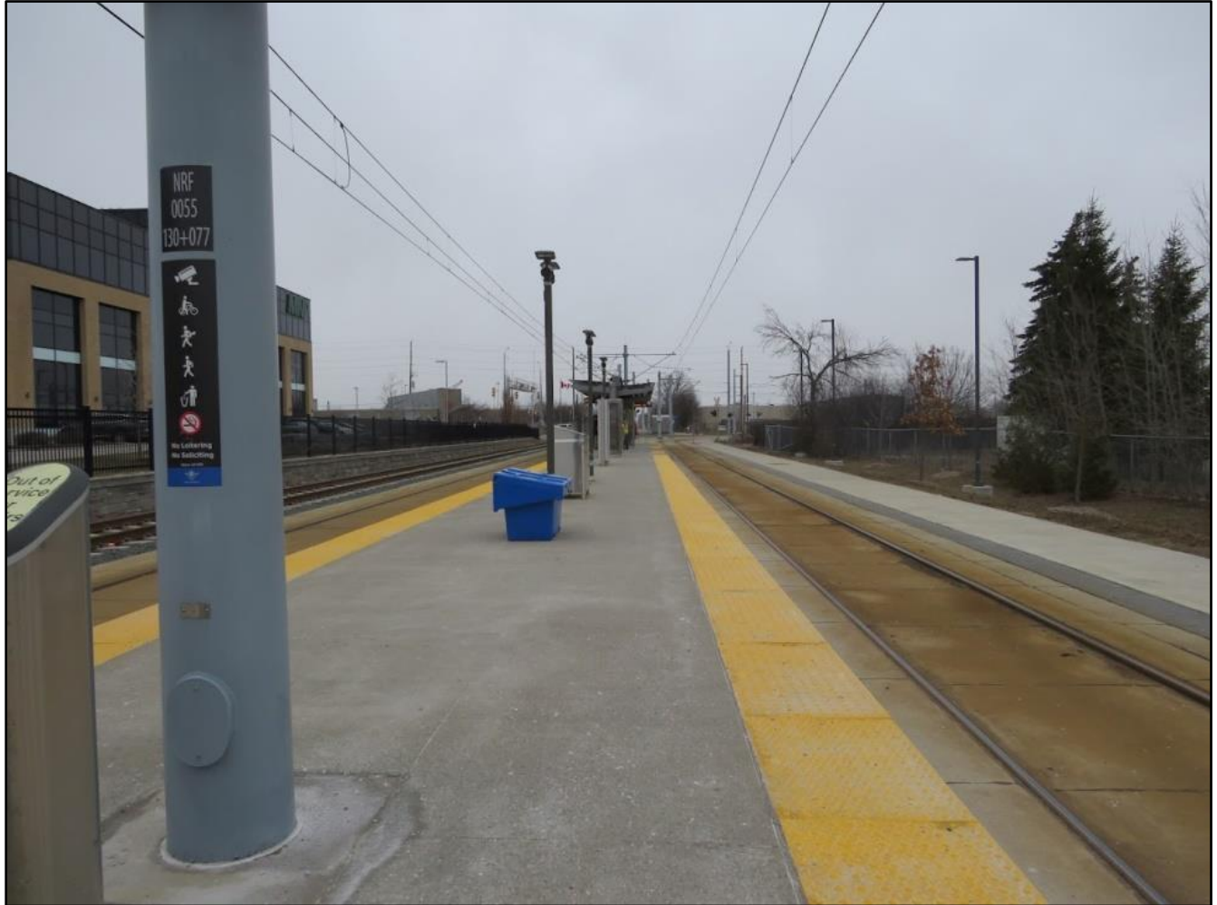
Figure 20: Platform view from the emergency exit
