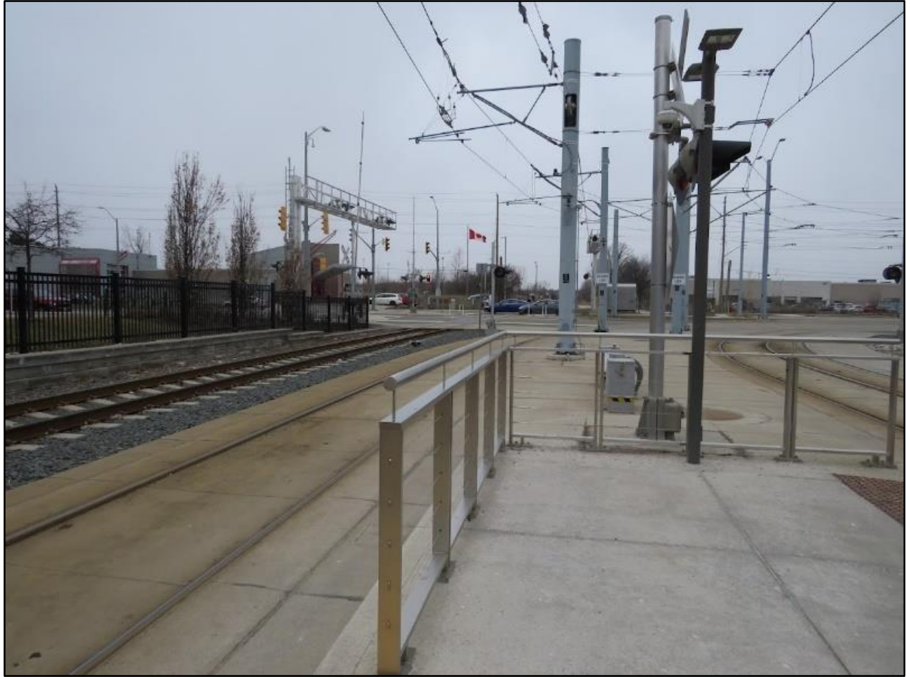
Figure 13: Opposite direction rail line, platform barrier and intersection behind
