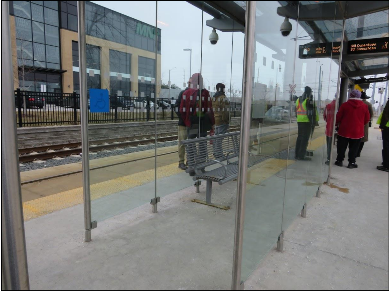
Figure 15: LRT Station Shelter (glass and polished metal) * **No high contrast or tactile markings to indicate entry point into the shelter
