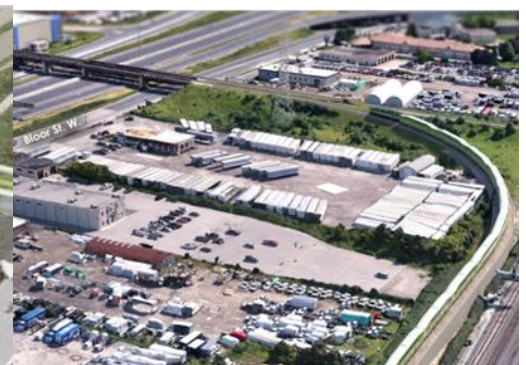
GO Rail Extension to Bowmanville
