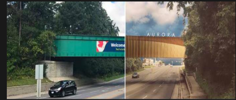
EXAMPLE: THE YONGE STREET RAIL BRIDGES, AURORA The bridge cladding and/or protective bridge barriers shall be treated as an additive feature
