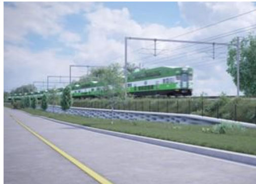
GO Expansion On-Corridor Works
