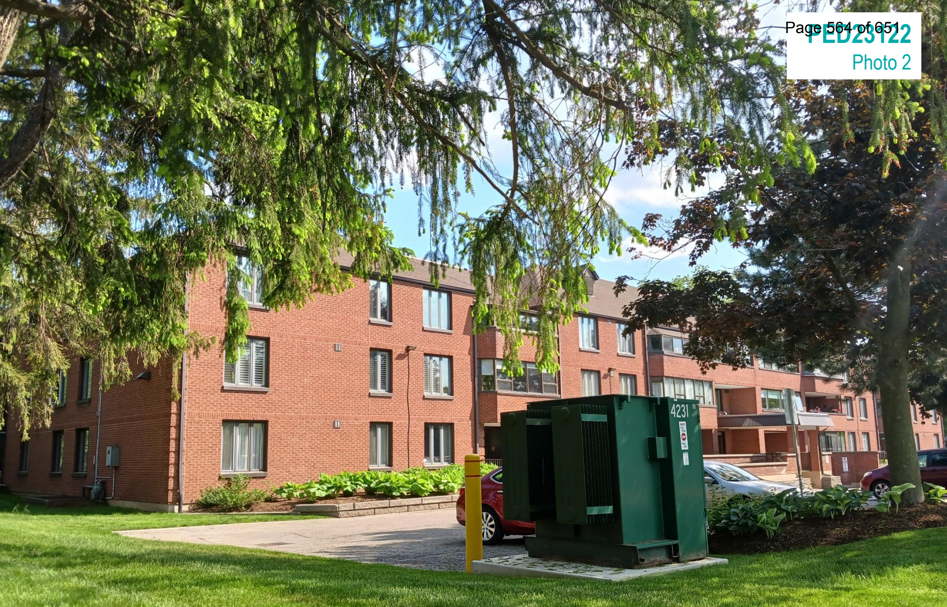
Adjacent multiple dwelling to west
