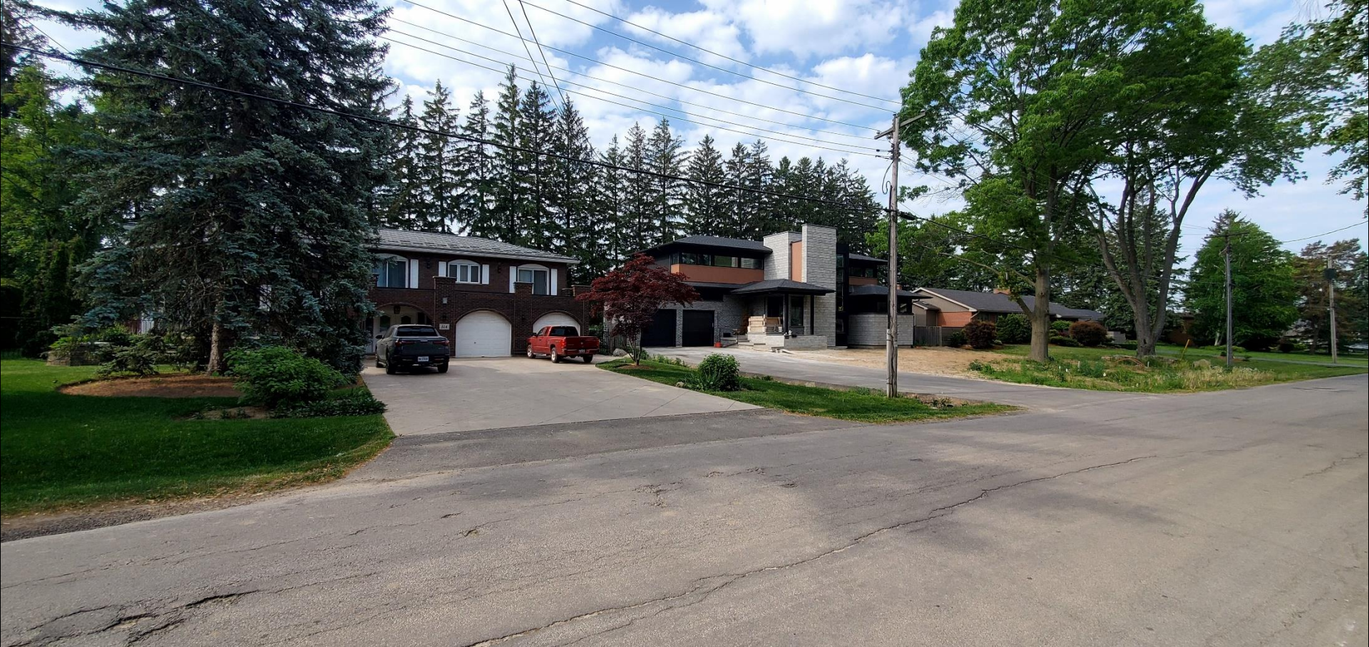
View looking southeast from Southcote Road
