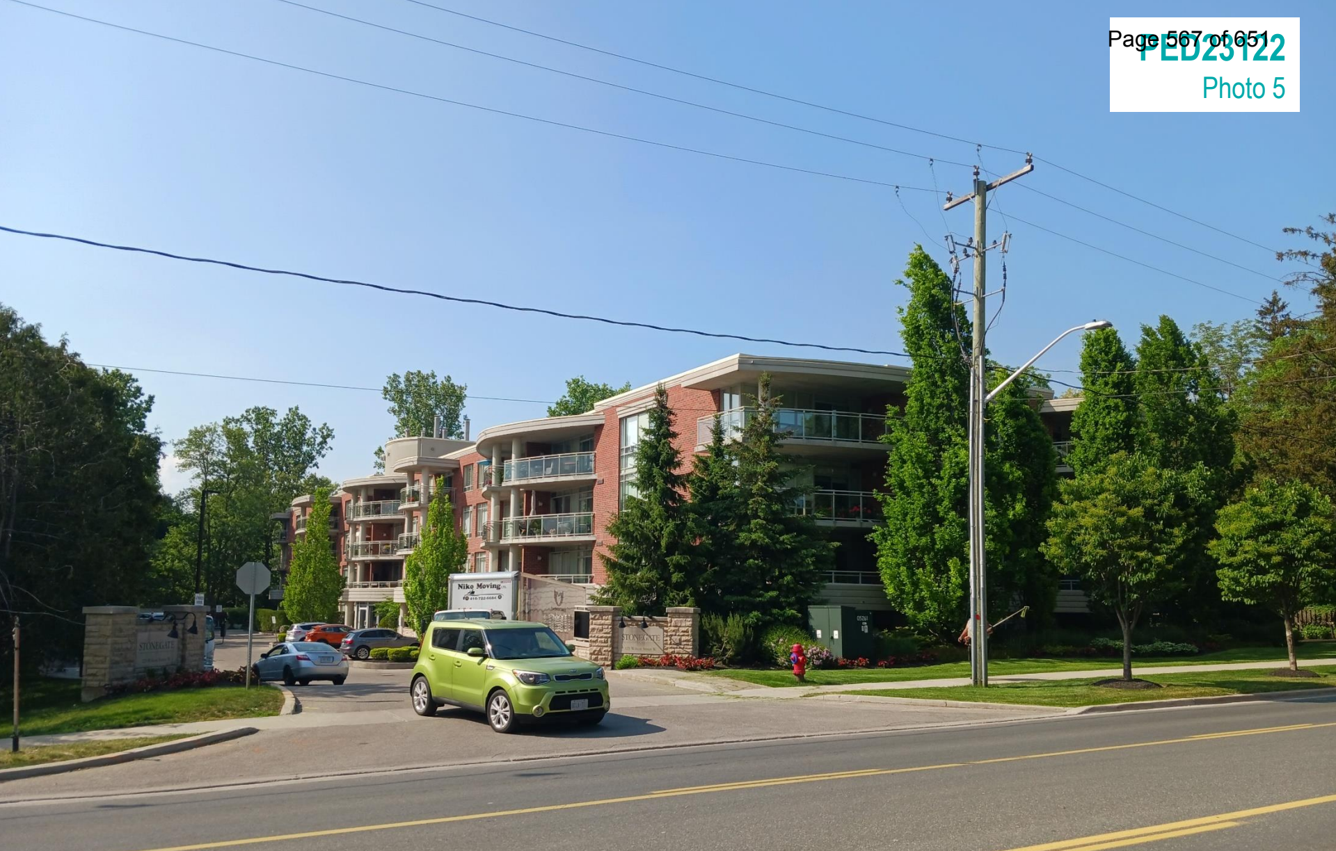
Multiple dwelling across Wilson Street West
