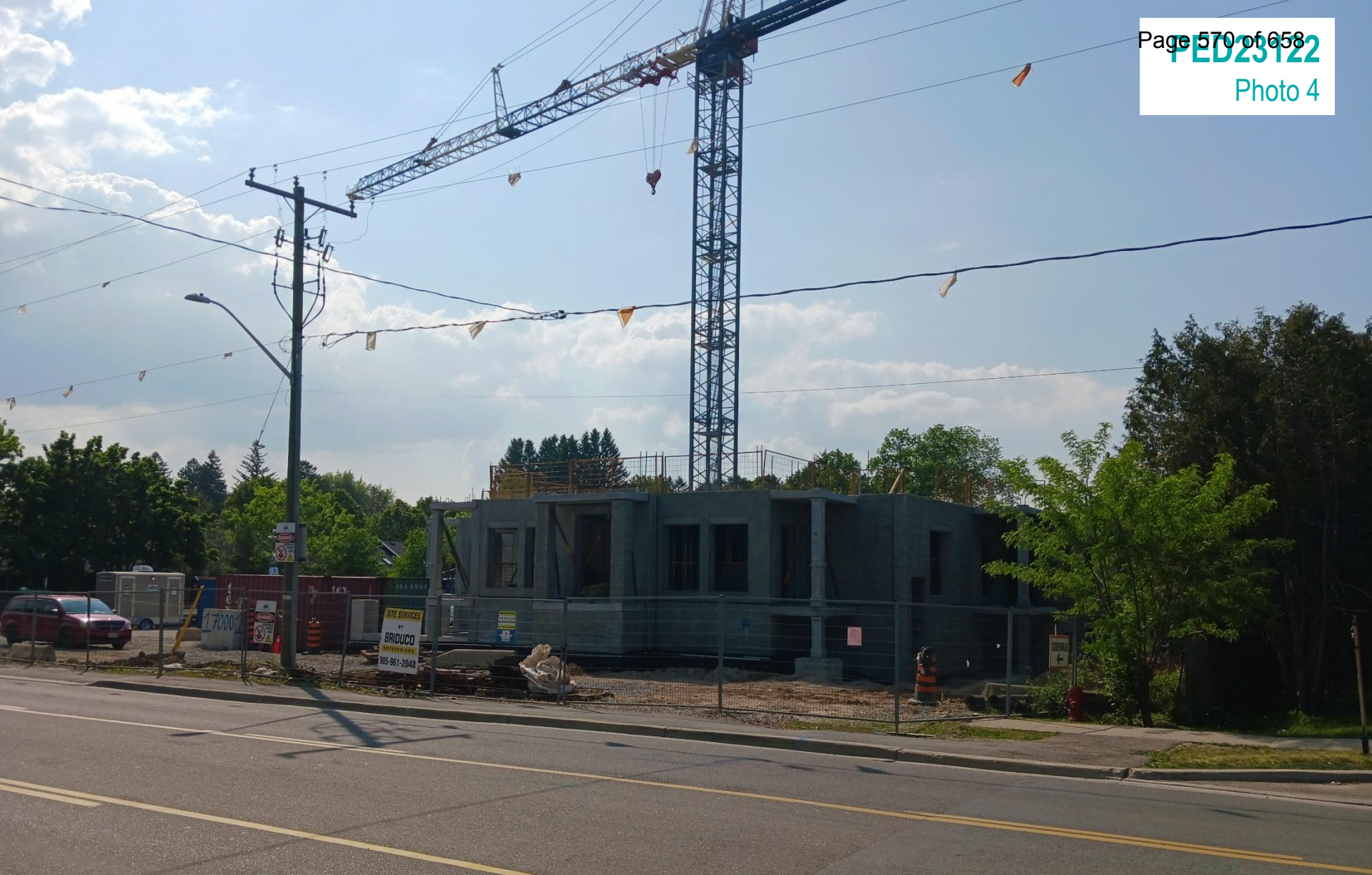
Multiple dwelling (under construction) across Wilson Street West
