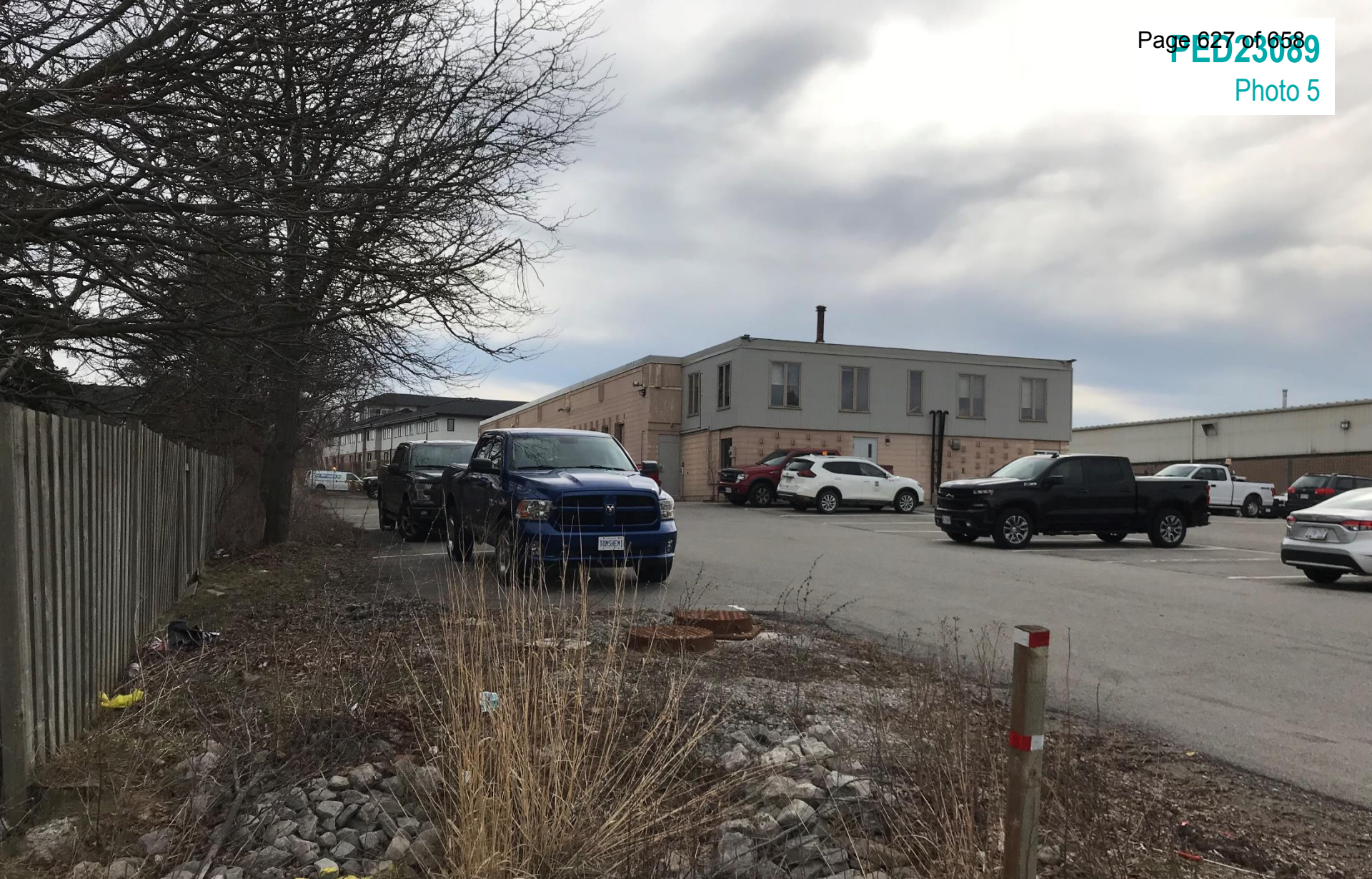
Public Works building located directly south of the Subject Property
