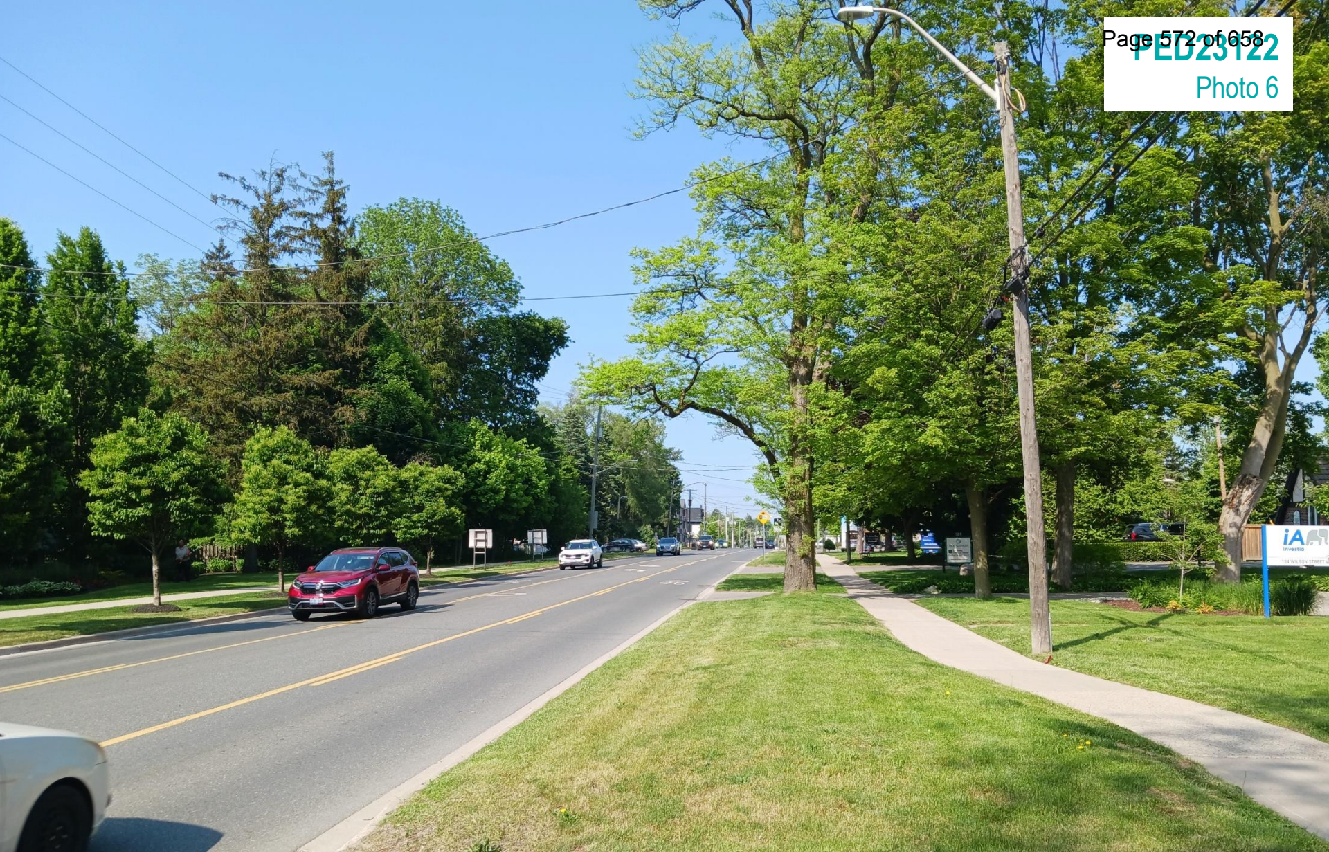
View to east along Wilson Street West
