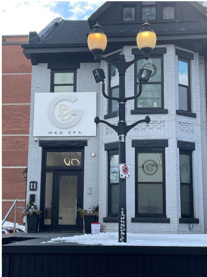
11 Hess Street South, Hamilton (Source: CDSB staff)
