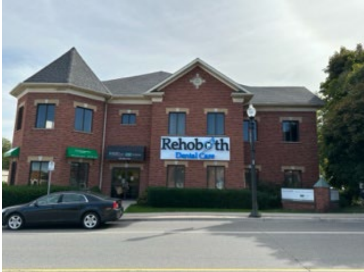
66 King Street East, Stoney Creek (Source: Applicant)
