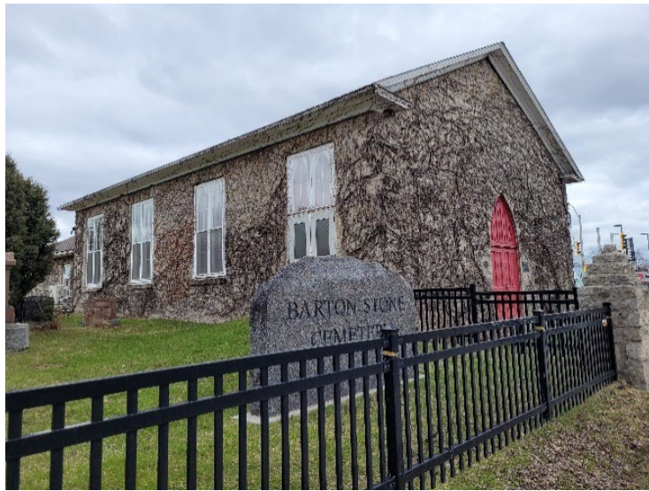
21 Stone Church Road West, Hamilton (Source: CDSB Staff)
