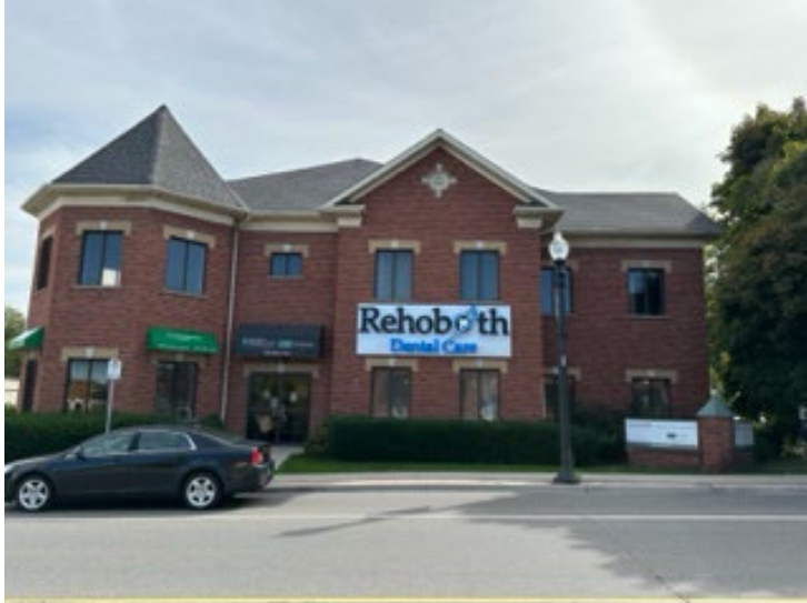
66 King Street East, Stoney Creek (Source: Applicant)
