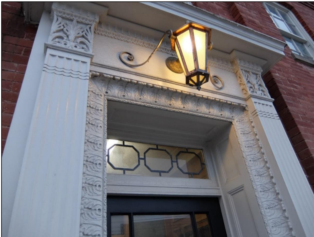
Image 6: Close-up on details of entrance to Building No. 7 (December 2022)
