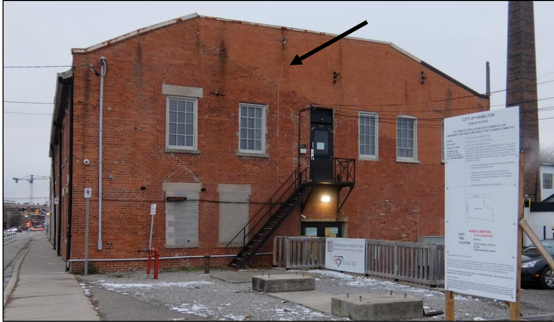
Figure 17: West wall of Building Nos. 2 and 5. Notice the difference in the colour of the brick, marking the former roofline of Building No. 2 (December 2022)
