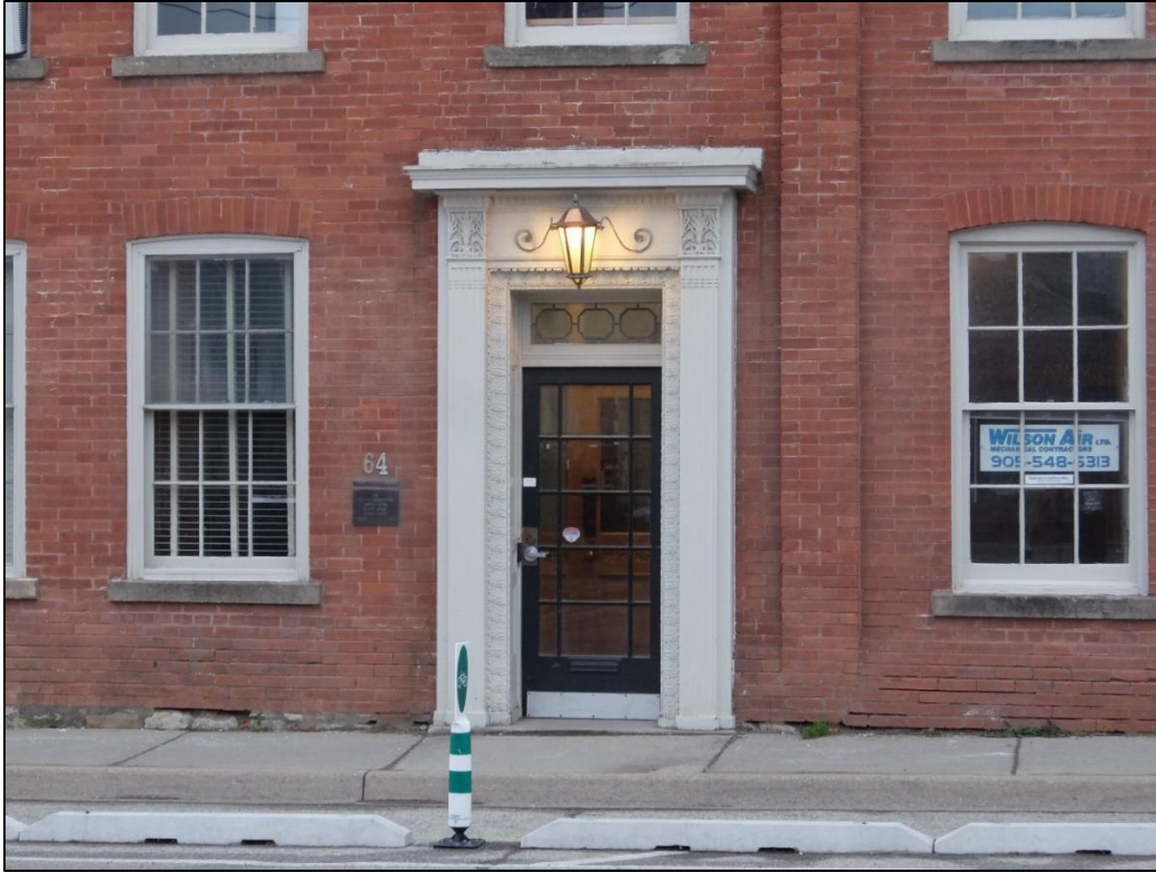
Image 5: Entrance to Building No. 7 (December 2022)
