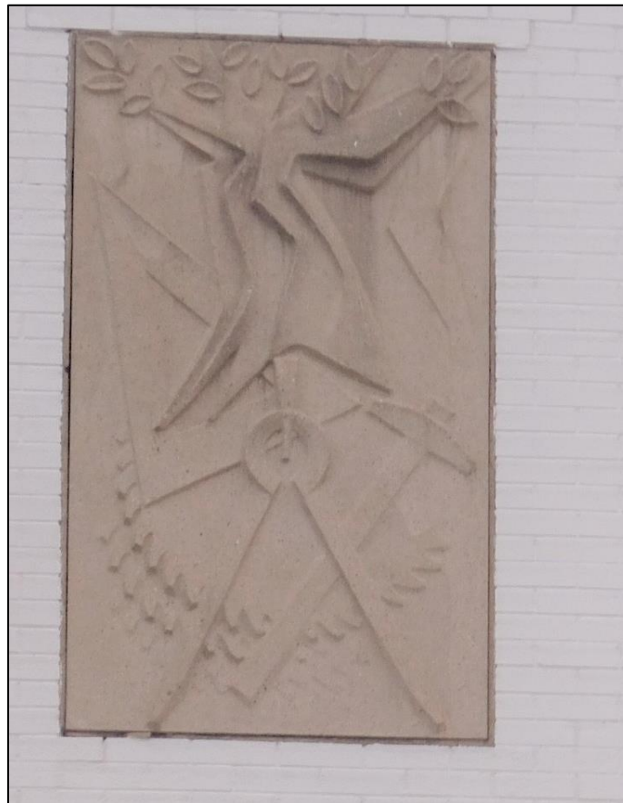
Figure 18: Details of decorative concrete panel on Building No. 11 (January 2023)
