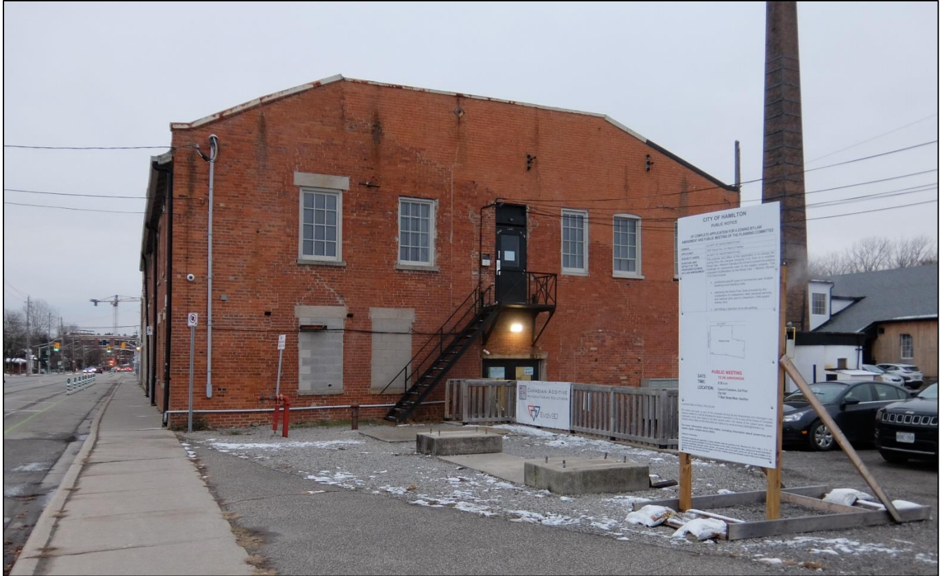
Image 11: Western elevation, Building Nos. 2, 5, and 3 (December 2022)
