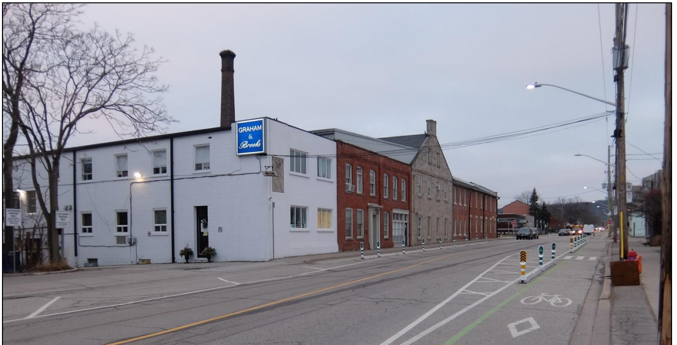
Image 14: 64 Hatt Street looking west (January 2023)
