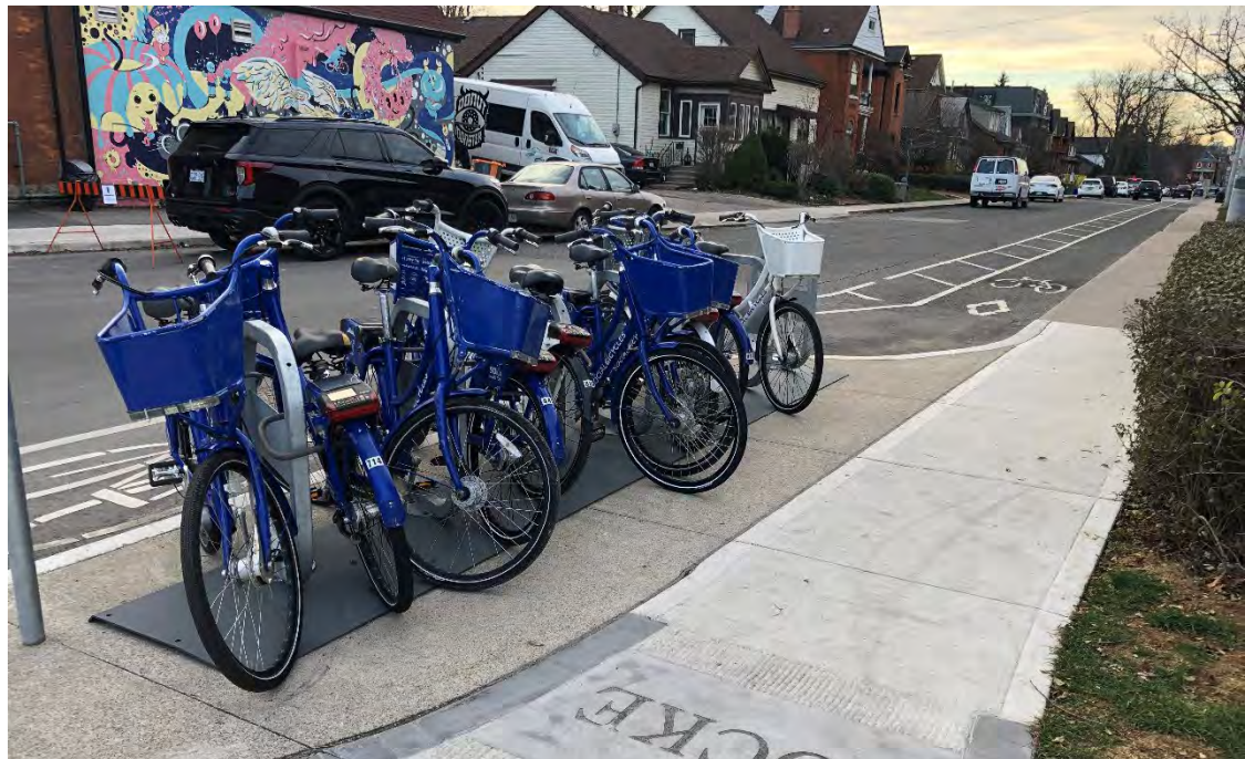
Exhibit 4-10: Curb Extension Retrofitted with Bike Share Station
