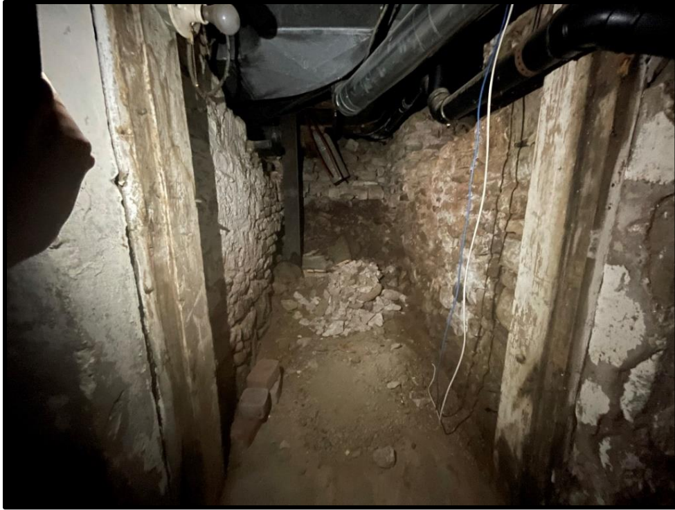
Image 73: Basement – Dirt Floor and Fieldstone Foundation (Photo taken on August 6, 2021)
