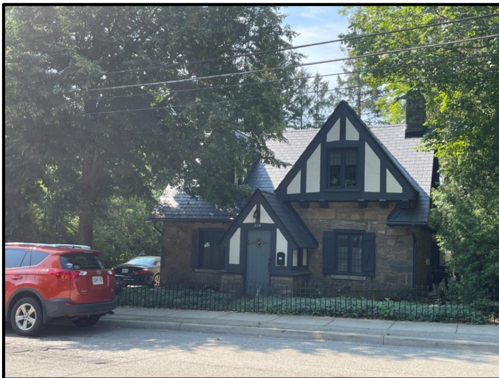
Image 42: 214 Park Street West (Photo taken on August 6, 2021; Facing South)
