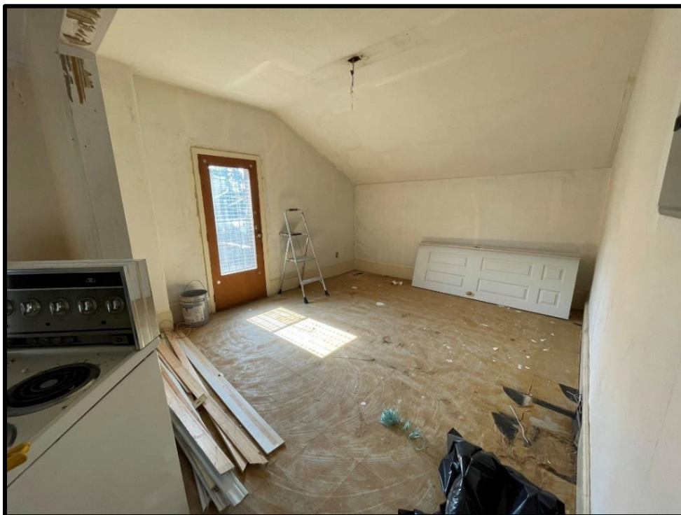
Image 62: Second Floor Open Area (Photo taken on August 6, 2021)
