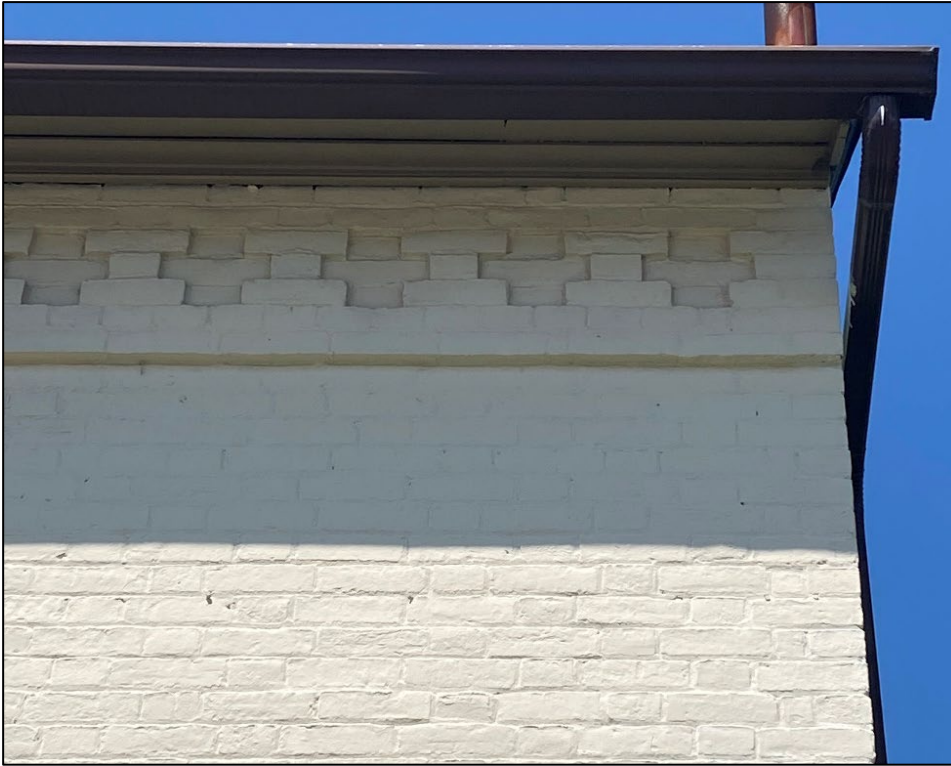
Figure 5 – 215 King St. W, Dundas, front elevation, close up of decorative cross brickwork under the eaves, Flemish bond and English corner detailing, July 2023
