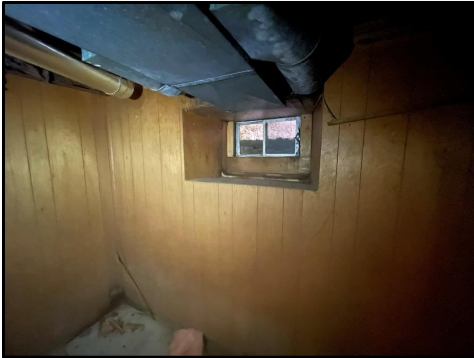
Image 79: Basement Window Well Showing Depth of Foundation (Photo taken on August 6, 2021)
