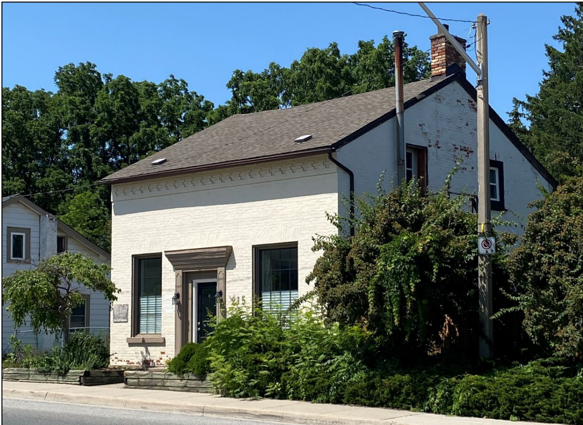
Figure 4 – 215 King St. W, Dundas, side elevation, July 2023
