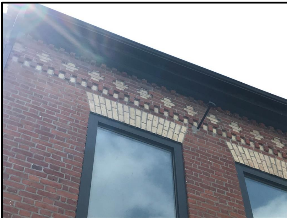
Image 82: 28 King Street West – Decorative Brick Detail (Photo taken on August 6, 2021; Facing Southeast)
