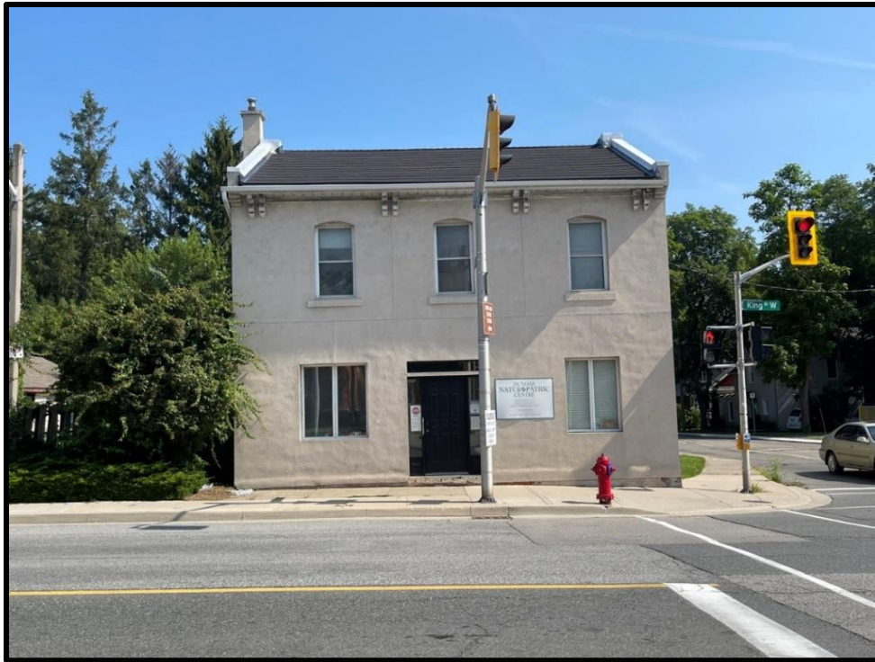
Image 41: 211 King Street West (Photo taken on August 6, 2021; Facing North)
