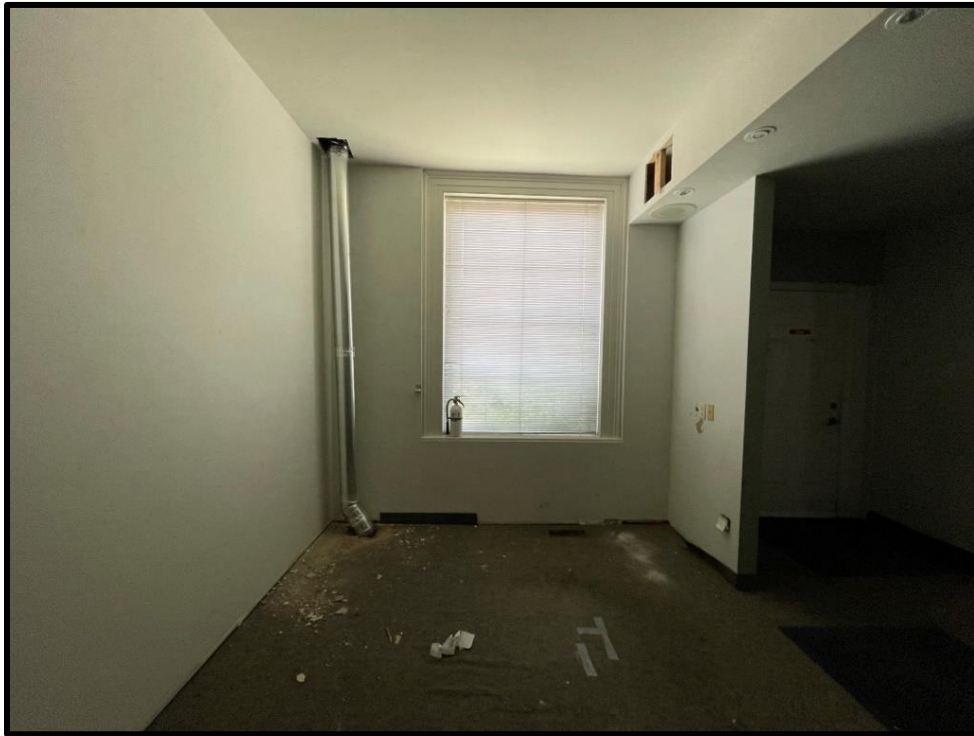
Image 47: East Window Opening on Façade (Photo taken on August 6, 2021)
