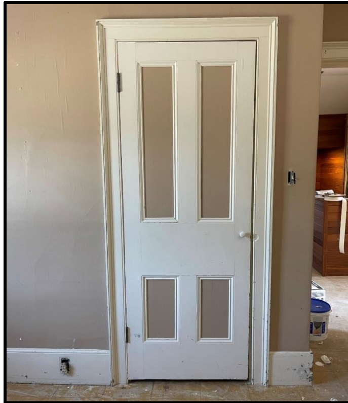
Image 69: Bedroom Closet with 4-Panel Door (Photo taken on August 6, 2021)
