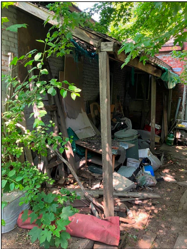
Figure 4: View of exterior of the dwelling.
