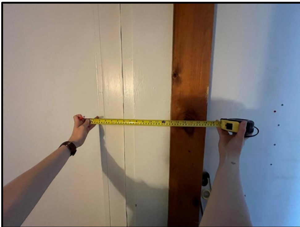
Image 54: Interior – Wall Thickness Between Brick Building and Rear Addition (Photo taken on August 6, 2021)
