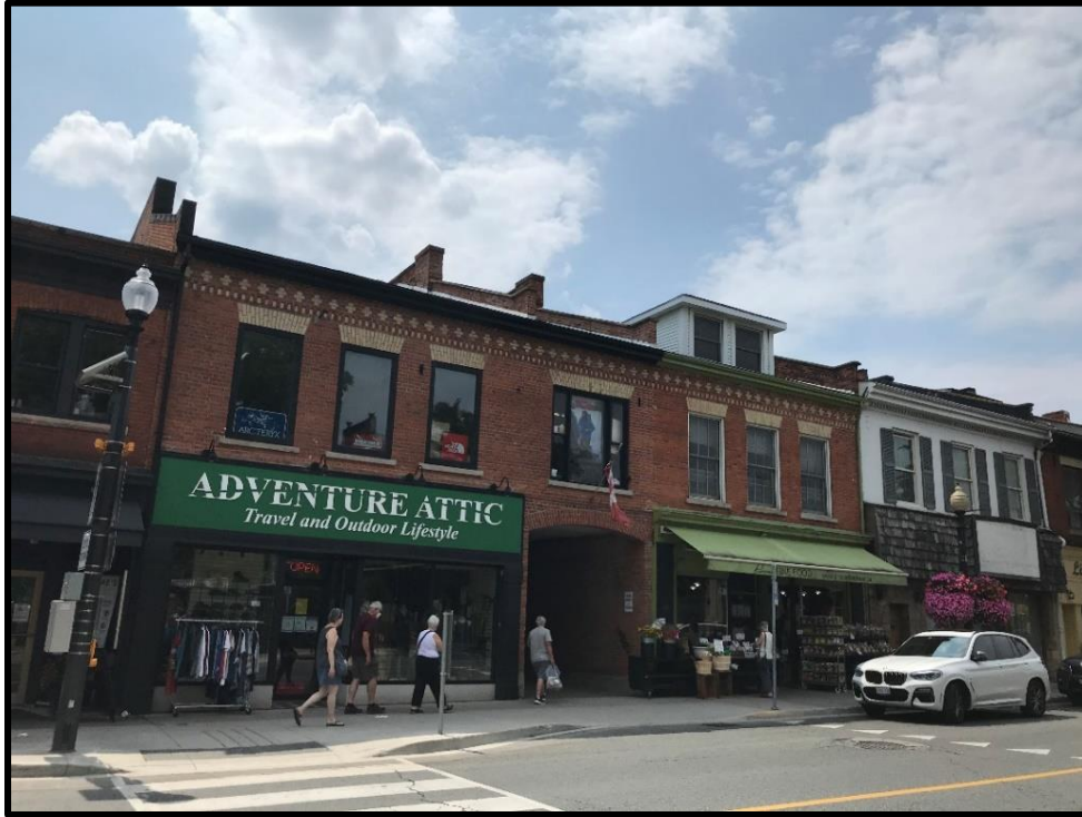
Image 81: 28 King Street West – Decorative Brick Similar to 215 King Street West (Photo taken on August 6, 2021; Facing Southeast)
