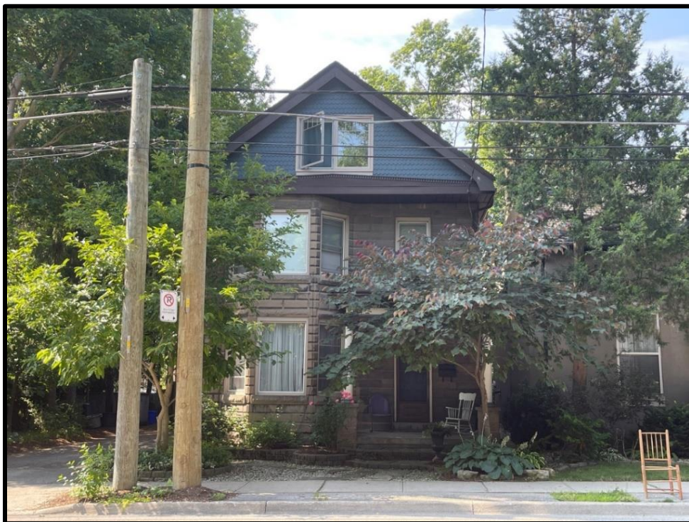
Image 44: 218 Park Street West (Photo taken on August 6, 2021; Facing South)
