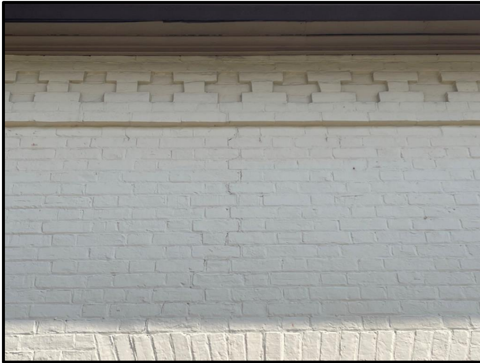
Image 5: Decorative Brickwork and Flemish Bond on 215 King Street West (Photo taken on August 6, 2021; Facing North)
