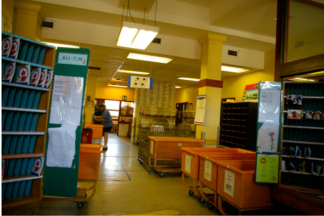
Photo 38: Ground floor looking directly south towards the back wall of the rear extension, with a partitioned office area not shown on the 1978 ground floor plan (A2: Figure 47 ). Nearest column, with the exposed cap, is one of the original four supporting the rear wall of the second storey.
