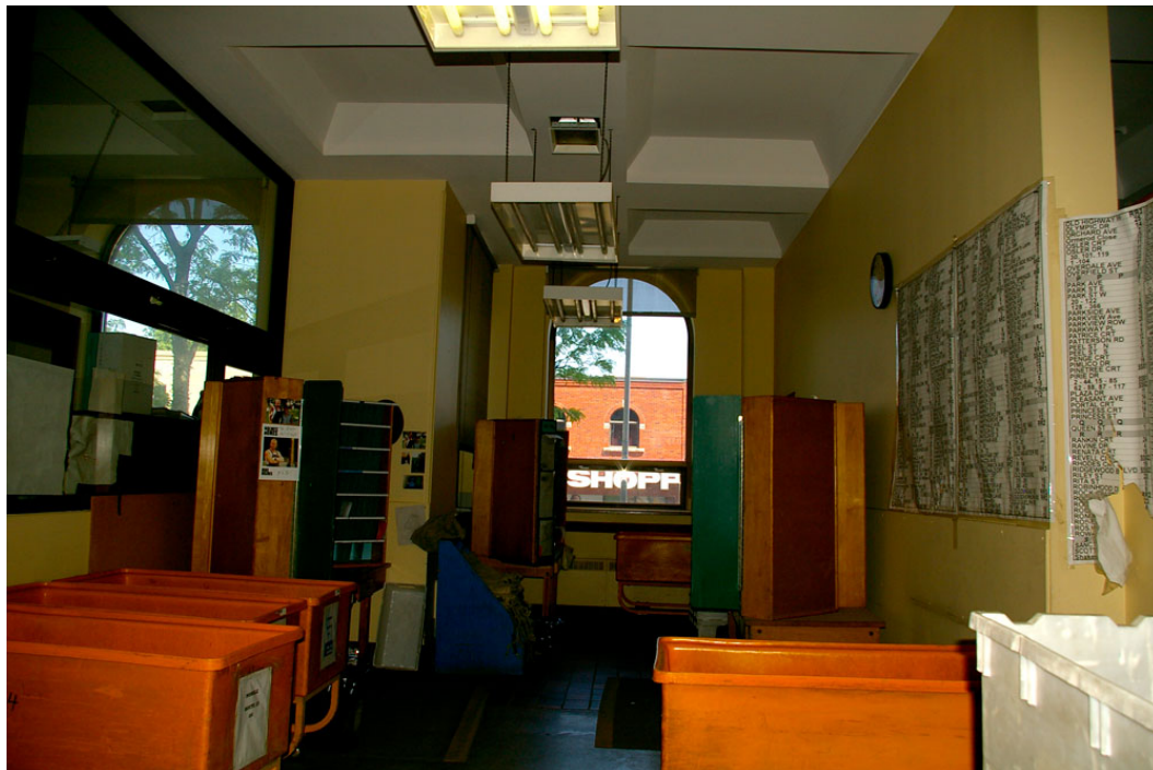
Photo 43: View looking north to the window on the west side of the front facade of the frontispiece, with the north-south glazed partition wall of the former Postmaster's Office as enlarged in 1979, visible to the left and shown on the 1978 ground floor plan (A2: Figure 47 ). The ceilings were not dropped in this area or the adjacent office.
