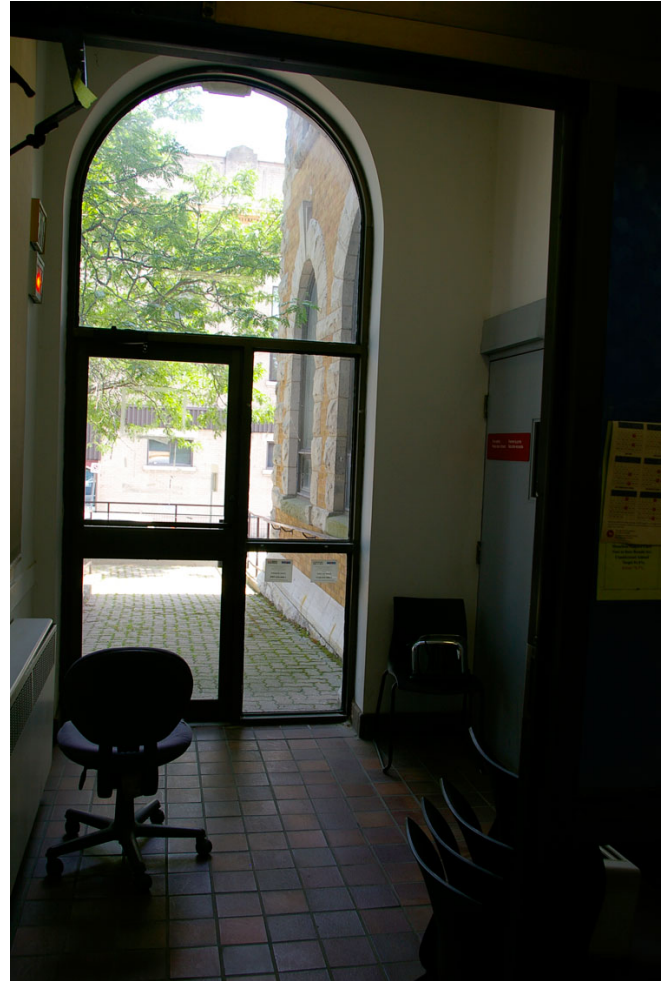
Photo 49 (left): Letter carrier's booth in the front entrance vestibule. The transom above marks the location of the inner set of vestibule doors installed in 1979.
