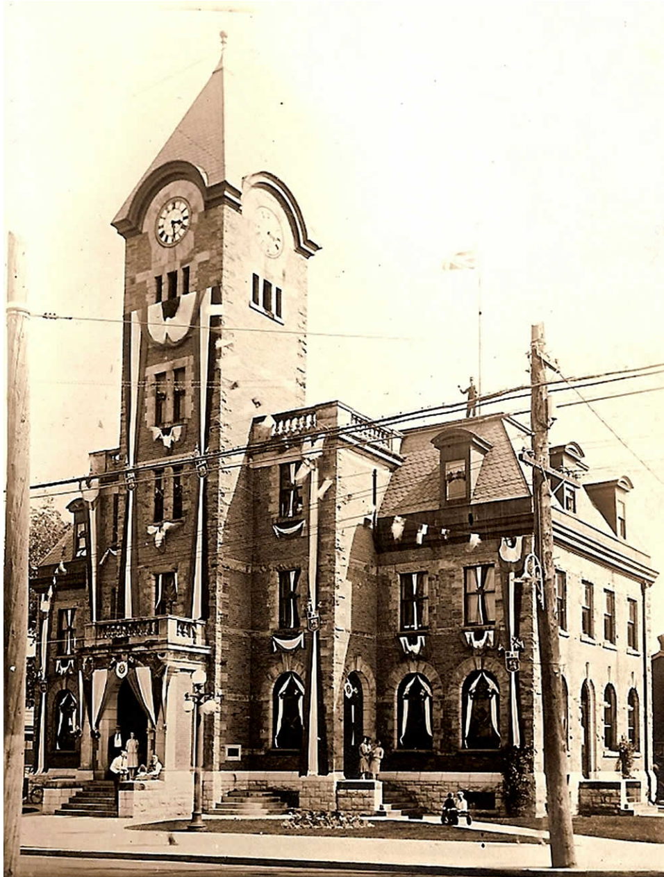
Figure 33: Postcard view of the Dundas Post Office decorated for the Confederation Jubilee celebrations held across the country on July 1 st , 1927, with people posing for this photograph. The building exterior is still in its original condition with no rear extension. Also shows the original landscaping, with grass-covered areas between the sidewalk, pathways and building and the circular flower bed in the grassy area at the north-west corner of the property.
