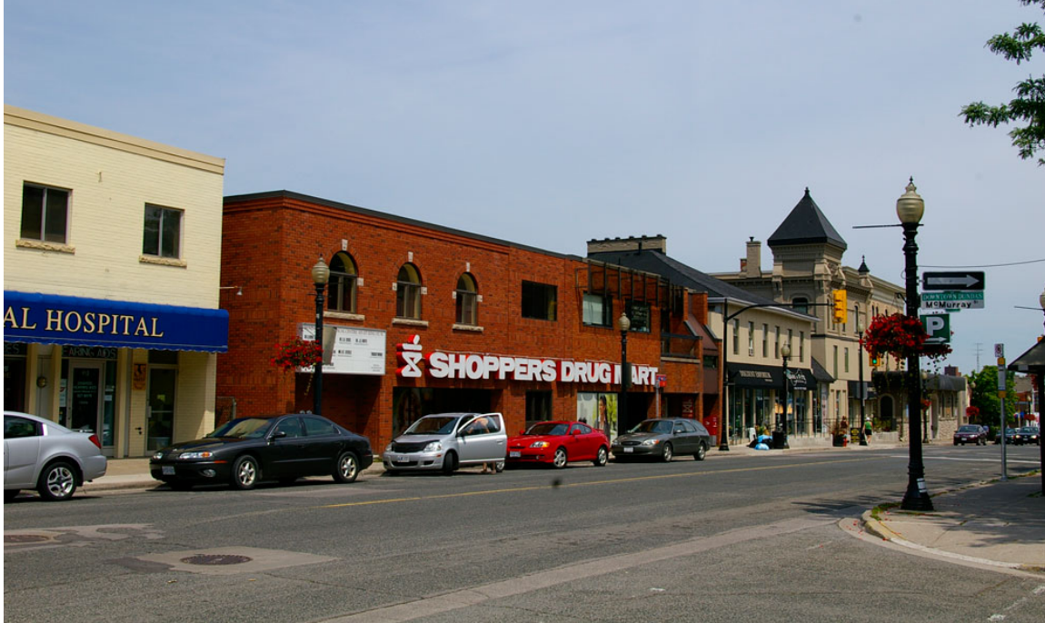
Photo 2: View of King Street looking north-east from the corner of McMurray Street. The building with the corner tower on the north side of King Street is the former Central Hotel. Directly across from the CPC property is a two-storey 1970s commercial block, largely occupied on the ground floor by a Shoppers Drug Mart, which housed the first Canada Post retail outlet in Dundas and continues to provide this service.
