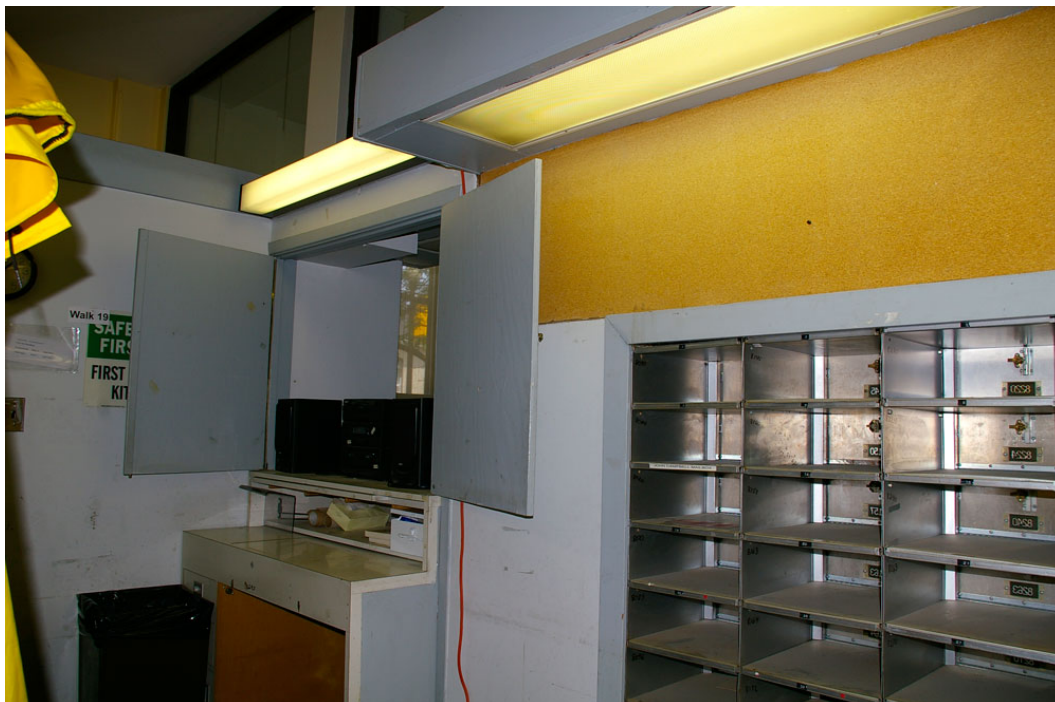
Photo 47: Staff side of the west wall of the former Lock Box Lobby looking north-east through the Dutch doors of the wicket towards the east entrance vestibule, as shown on the 1978 ground floor plan (A2: Figure 46).
