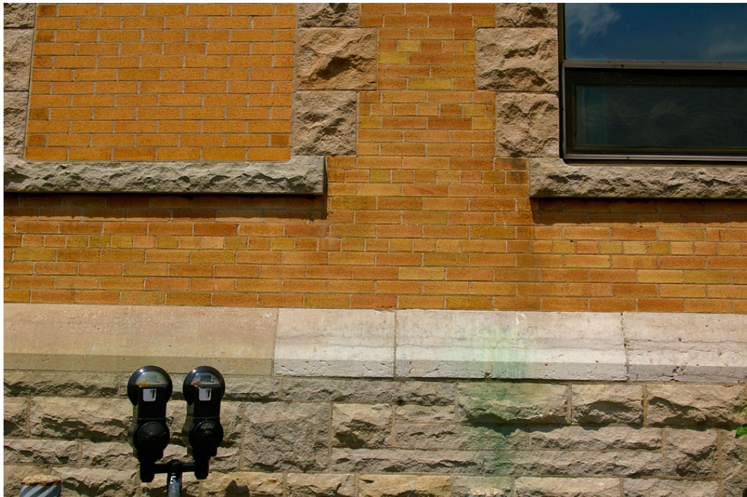
Photo 24: Detail of the foundation wall of the pre-1949 rear extension, showing some of the original stone caps salvaged from the original rear wall and a longer poured concrete capstone to the left. Also shows the double brick masonry construction of the extension with one header course for every four stringer courses (same as the original building).
