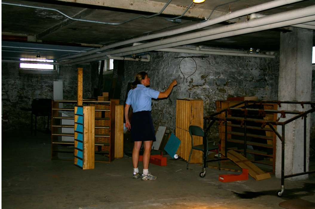
Photo 30: Inspection of the basement with Office Supervisor Kim Thomas. View looking towards the north-west corner with the west and north facing windows on the left and the north window of the frontispiece on the far right partially obscured by one of the two reinforced concrete columns supporting the back half of the clock tower.
