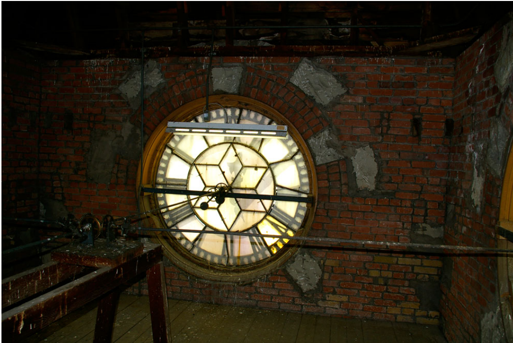
Photo 81: One of the clock dials showing the interior construction of the metal and glass dial set in a circular wood frame. Visible through the opaque glass are the Roman numerals on the outer face. In recent history the clock dials have been illuminated by fluorescent lighting tubes.
