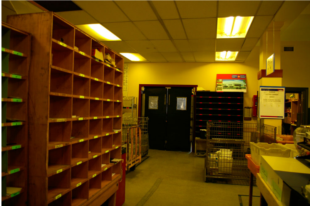
Photo 40: Ground floor looking directly west to the one set of double swinging doors opening onto the Mail Lobby, with the doorway to the former Vault visible to the right of the column.
