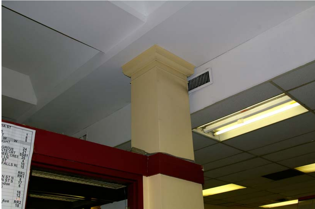
Photo 46: Detail of one of the original column caps left exposed by the higher ceiling in this area. The column, located at the south-west corner of the Registration Room, is one of four supporting the rear wall of the second storey.
