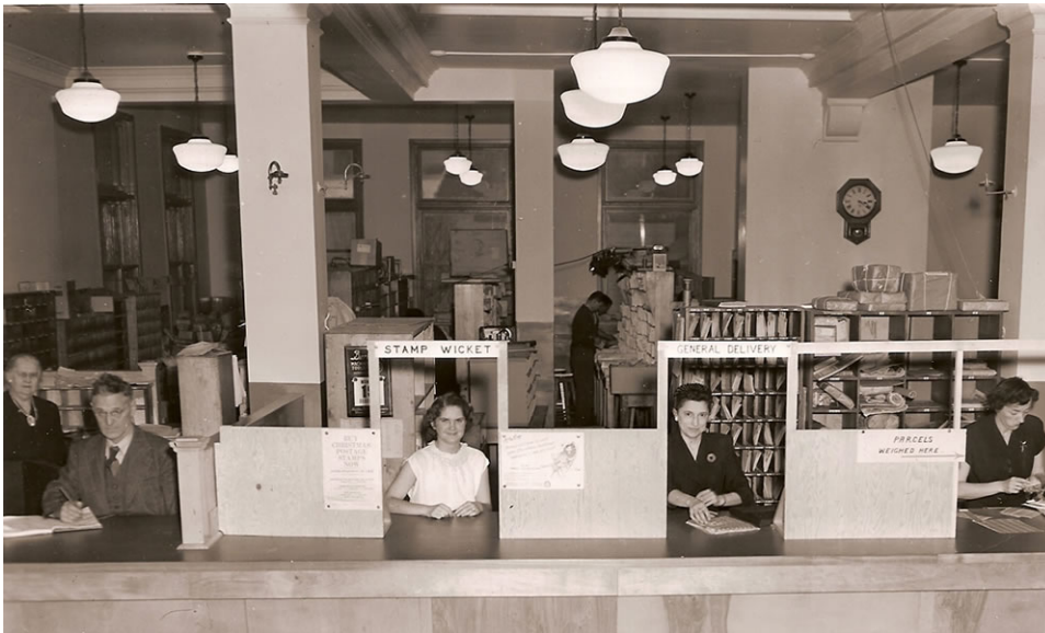
Figure 39: View of the new front counter faced with marble (wickets still under construction) and counter staff in December 1949, looking towards the rear extension. Also visible are the supporting piers marking the location of the original back wall and three of the five south-facing windows and the two east-facing ones. By this date, the original suspended lighting fixtures had been replaced by more contemporary ones (compare with fixtures shown in Figure 37 ).
