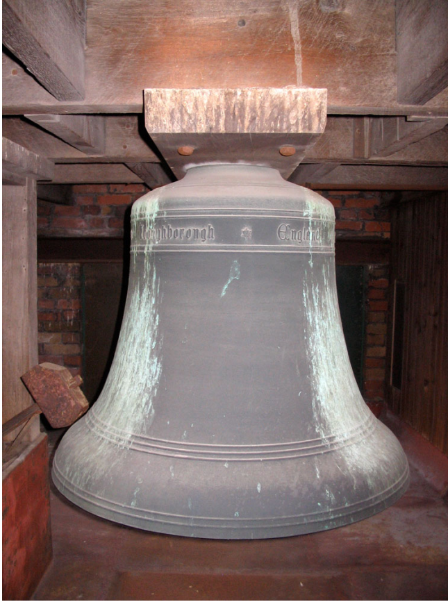
Photo 78 (left): Bell showing method of suspension from a thick plank bolted to two ceiling joists.
