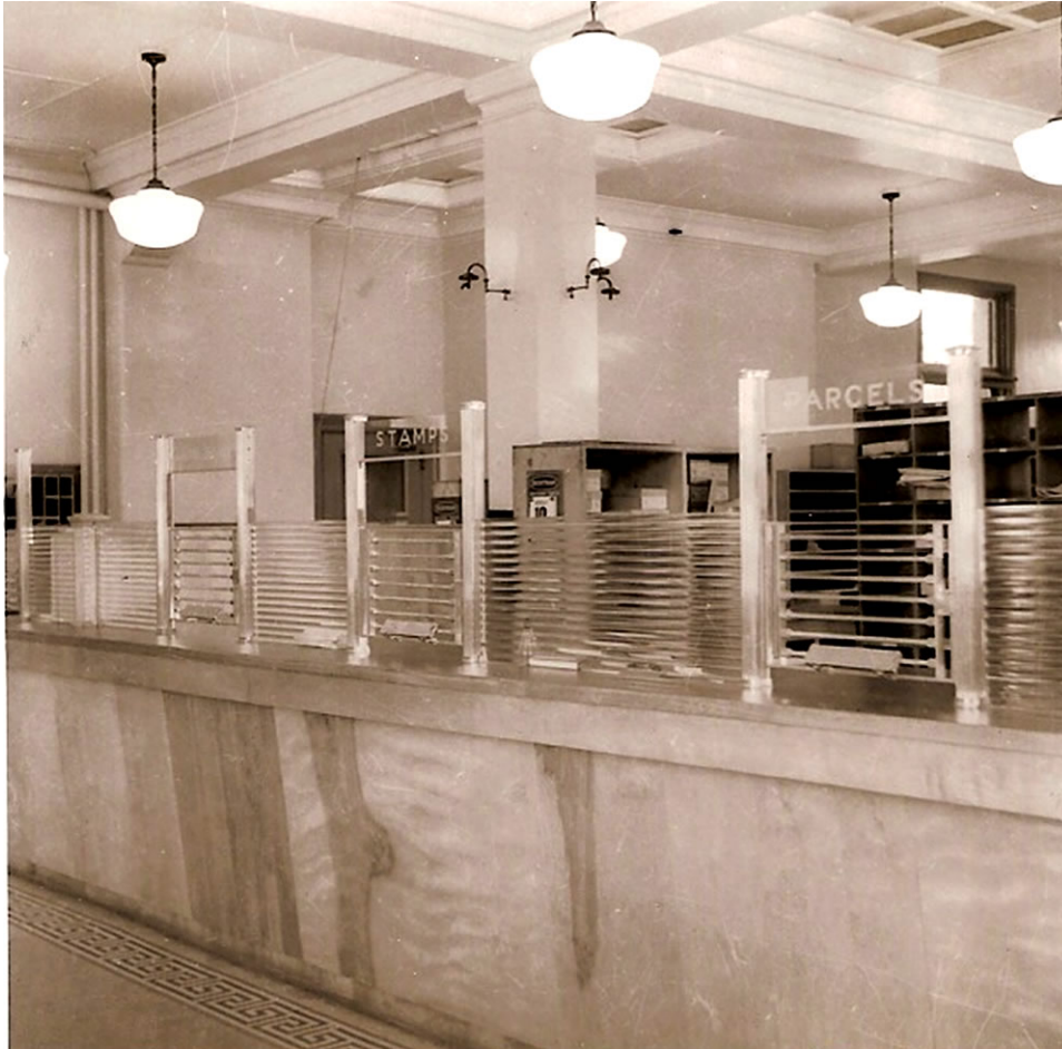
Figure 40: Counter as completed with the new wickets in place in 1950. Visible beyond is the transom of one of the east-facing windows and in front of the counter the terrazzo floor with its decorative tile border.
