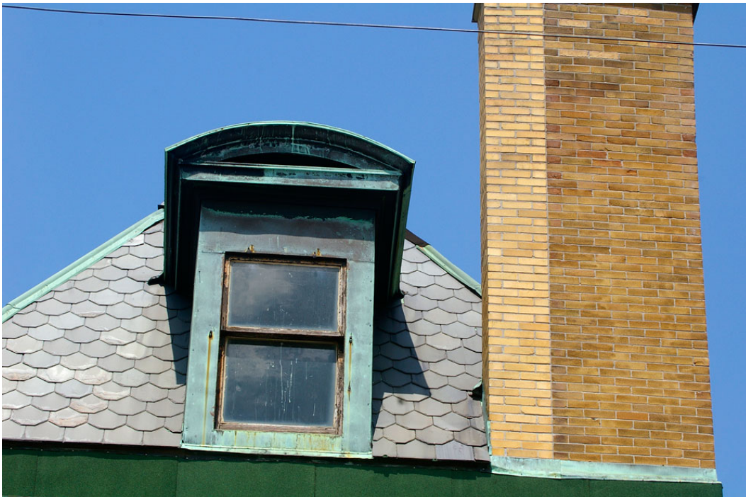
Photo 20: Close-up view of the south-facing slate mansard roof of the east wing, with its copper-clad dormer, and the original brick chimney with a third flue added to its west side (date unknown). All of the dormers are identical to this one, featuring a curved roof with a front-facing segmental arch and a one-over-one wood sash window.
