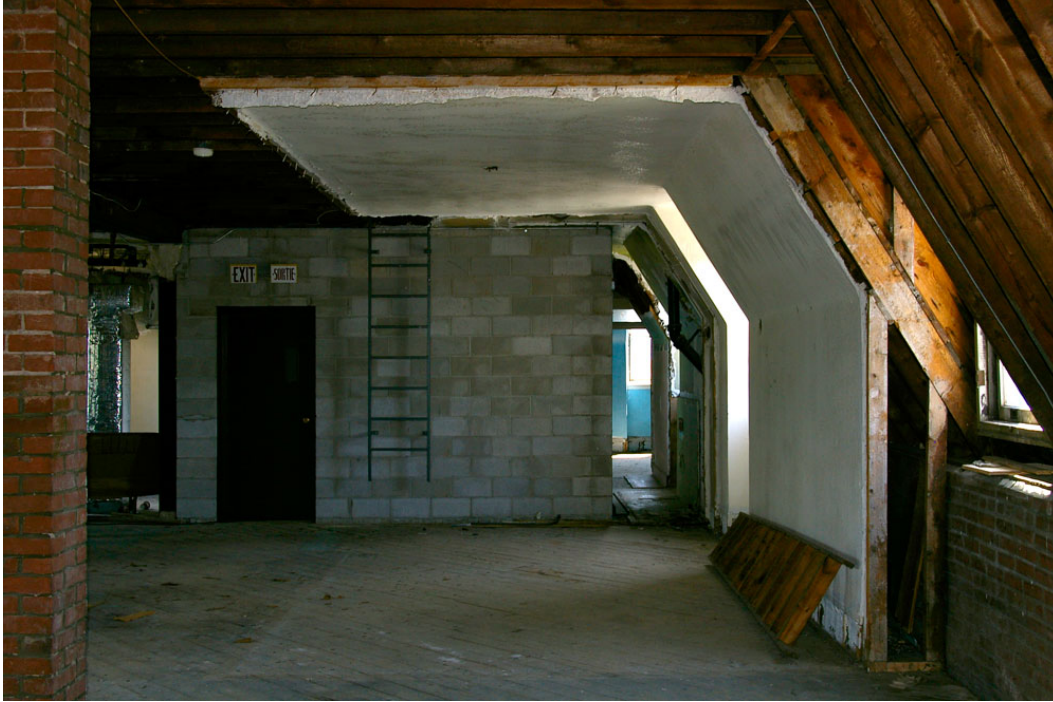
Photo 64: Third floor looking directly east towards the concrete block enclosure of the stairwell which replaced the original wood staircase in 1979 and left only a narrow passageway to the remaining rooms of the caretaker's apartment, which was then rendered unusable. The window directly ahead on the east facade was located in the second bedroom. The bathroom would have occupied part of the narrow passage, as shown on the Third Floor Plan, as revised in 1924 (No. 4: Figure 21 ).
