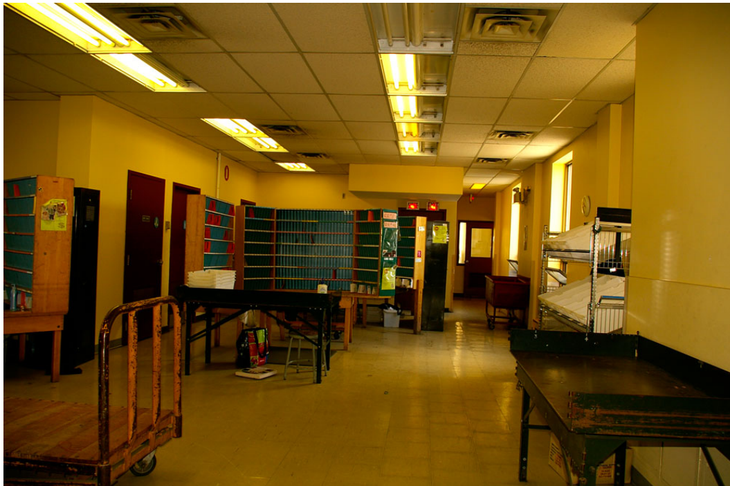
Photo 56: Second floor looking east towards the open doorway to the lunch room in the south-east wing, with three doors on the left (from west to east): the janitor's closet, the men's washroom and the women's washroom (barely visible in the corner above a sorting booth). Directly ahead but mostly obscured from view is the doorway (fire exit) to the enclosed concrete block stairwell constructed as part of the 1979 renovations.
