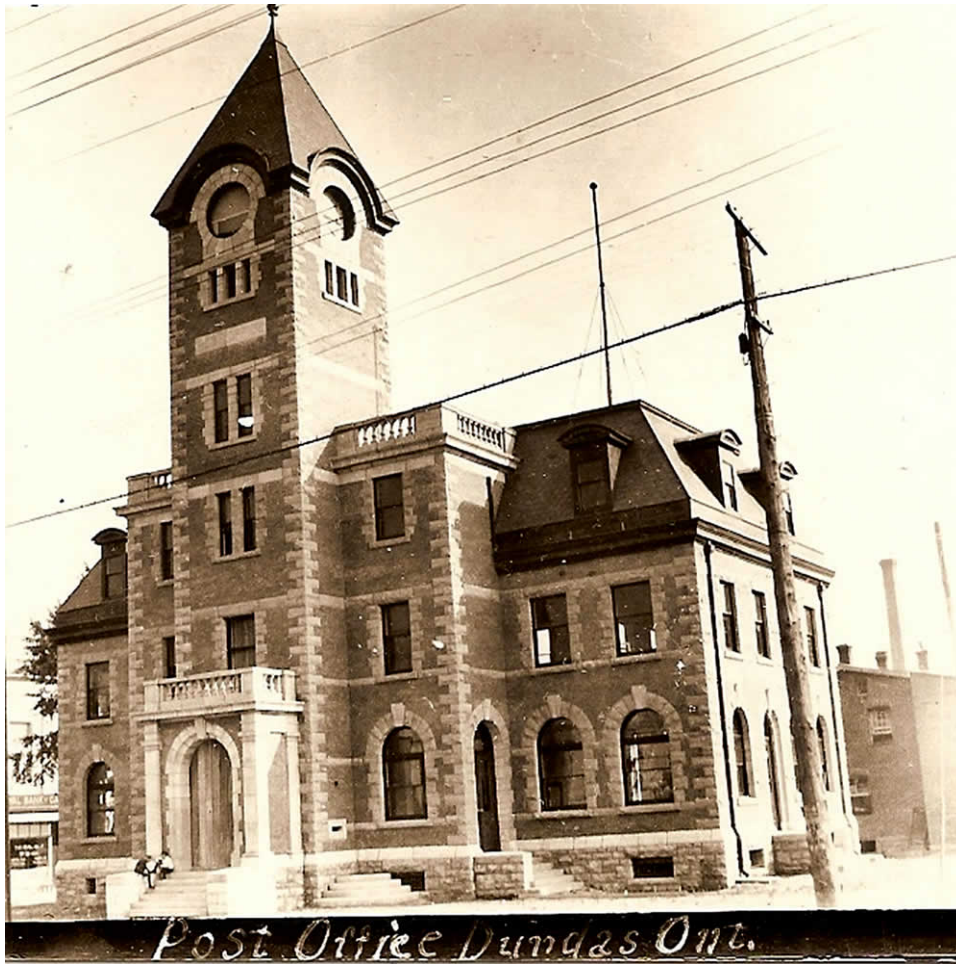
Figure 29: Postcard view of the Dundas Post Office looking south-east, which also shows part of the two-storey building directly behind on McMurray Street (since demolished). Photo taken in the summer or early fall of 1913 after the building exterior had been completed. The openings for the clock dials are shown covered from the interior with temporary wood sheathing.
