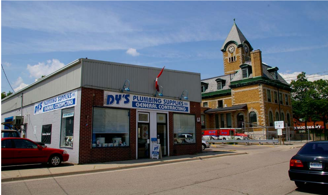
Photo 4: View looking north-west across Foundry Street to the CPC property with the front half of the one-storey concrete block building that originally housed the Brewers Warehouse visible on the west side of Foundry Street.
