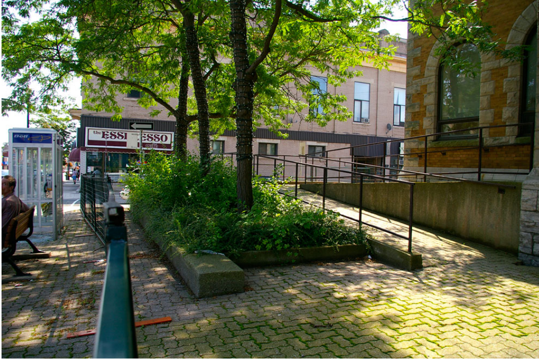
Photo 87: View of front landscaping looking east towards Foundry Street with the concrete planter and ramp installed in 1979. Similarly, to the west planter, the east planter contains low perennial shrubs, ground cover and three locust trees.
