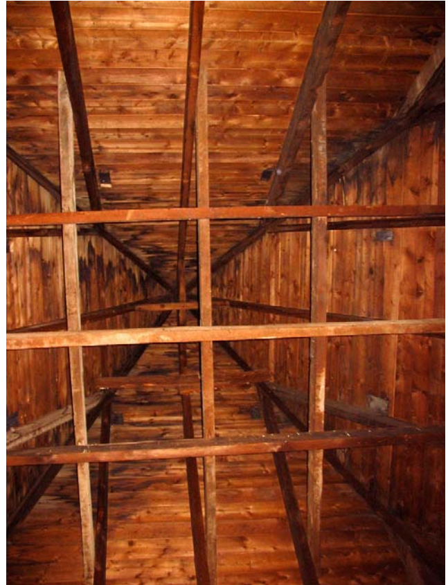
Photo 82 (left): Clock dial assembly showing the vertical drive shaft going through the floor to attach to the mechanism on the fourth floor.
