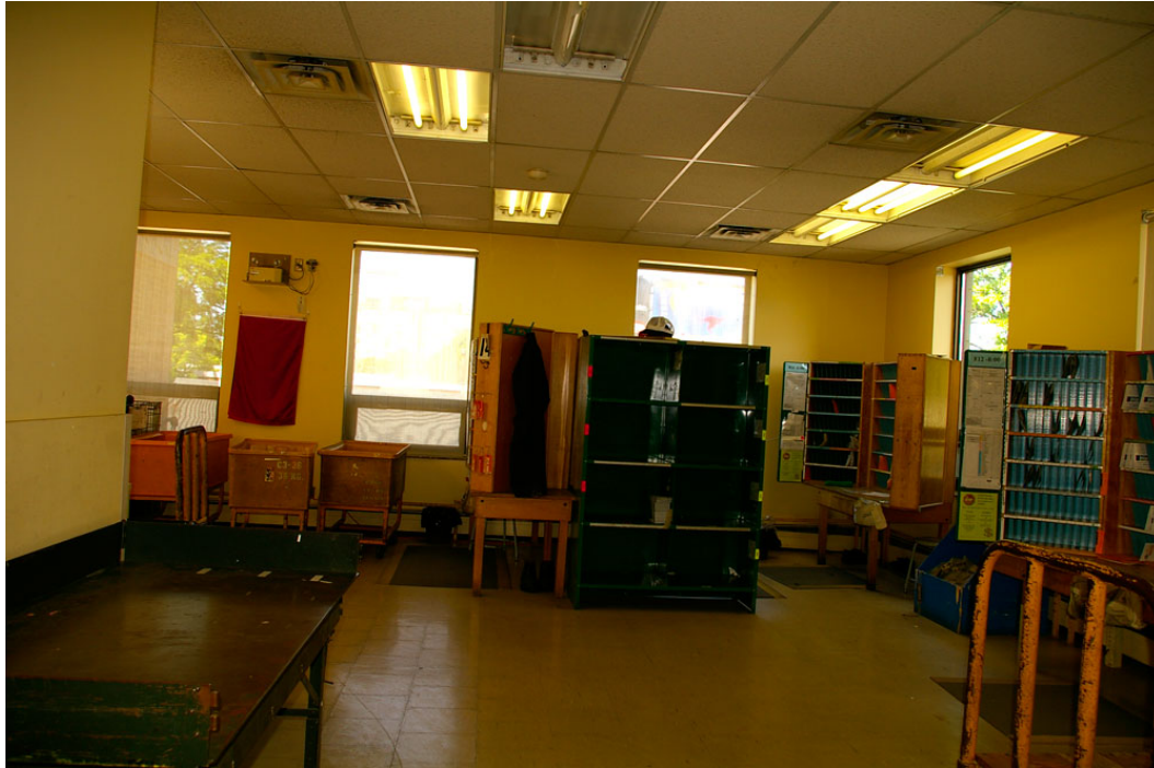
Photo 55: North-west corner of the second floor looking west. The linoleum tiles are identical to the ones on the ground floor, all laid as part of the 1979 renovations.
