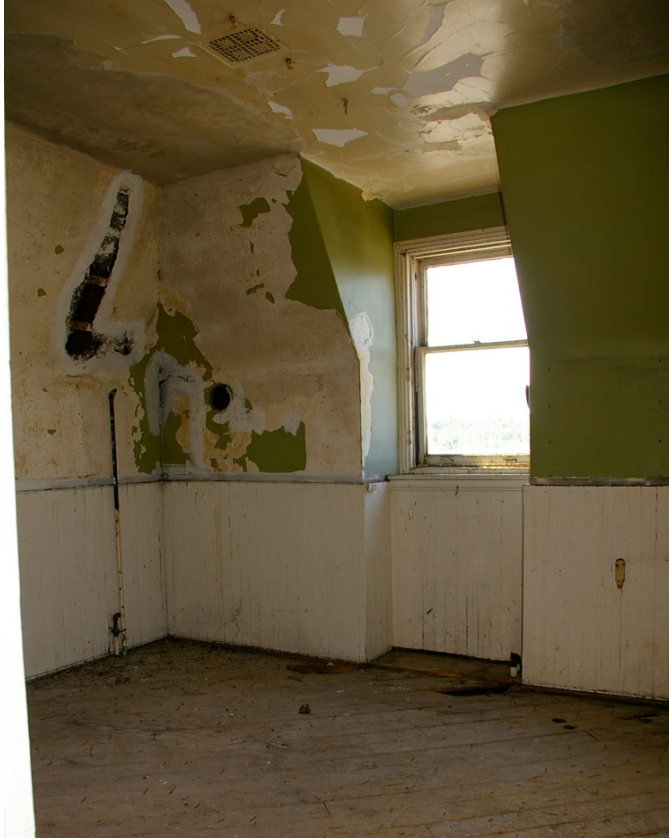
Photo 68 (left): Kitchen of the caretaker's apartment, stripped of radiators and plumbing fixtures. View looking towards the rear window in the south-east wing. Shows the slope created by the mansard roof and the vertical board wood wainscoting below the level of the window sill. The original flooring in the kitchen and bathroom was likely linoleum, all removed revealing the diagonal board sub-flooring.
