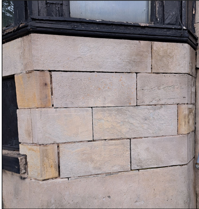
Closeup of cut-stone even course façade
