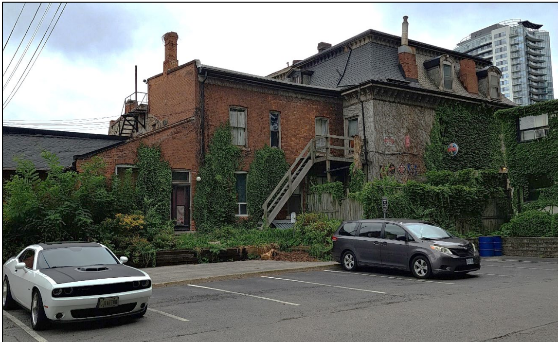
Side (south) elevation of 56 Hess Street South
