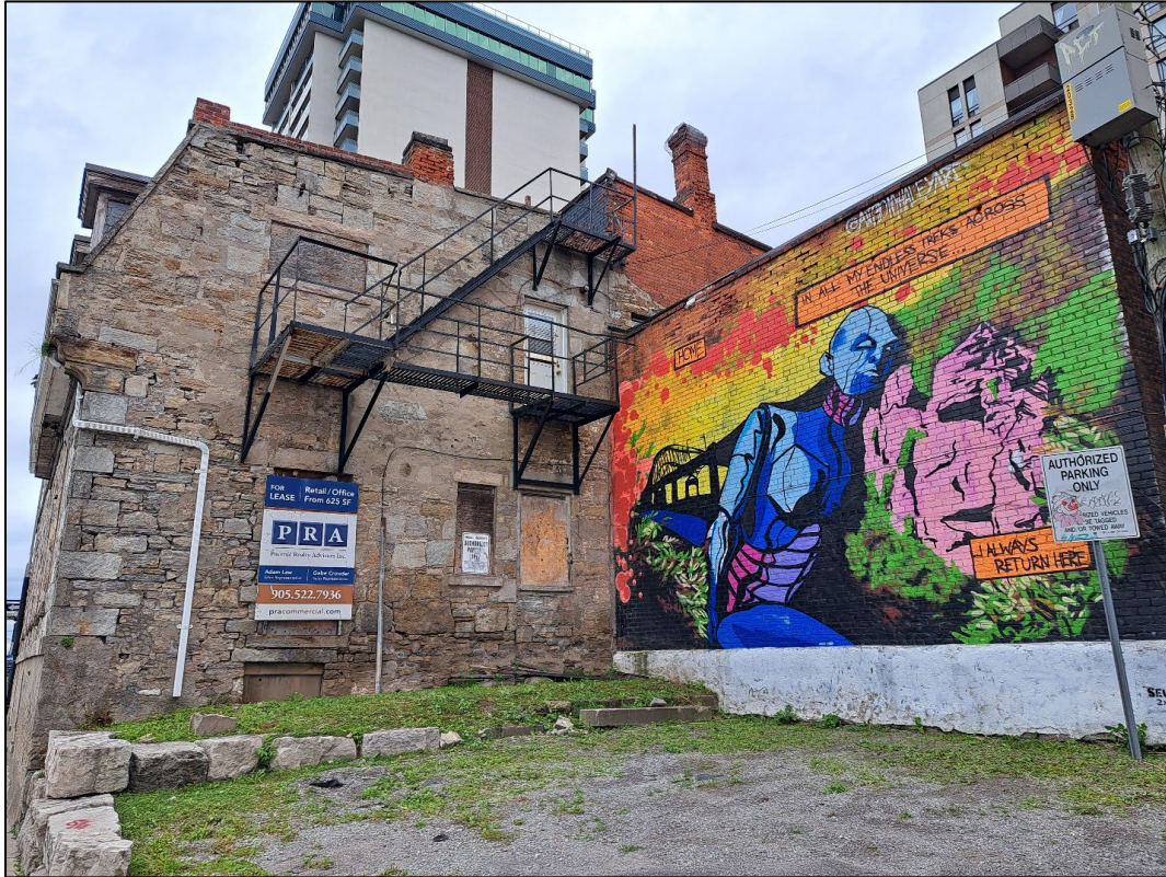
Rear (west) elevation of 54 Hess Street South (left) and north elevation of the painted rear brick wing of 56 Hess Street South (right)
