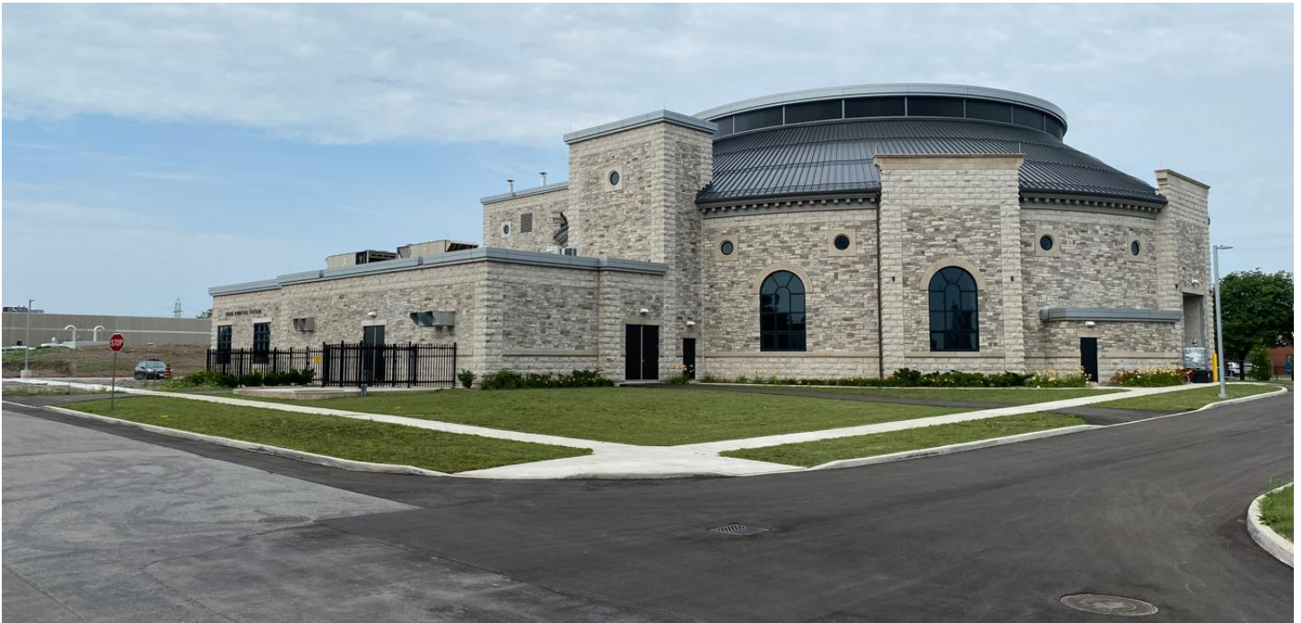
Figure 1: New Main Pumping Station
