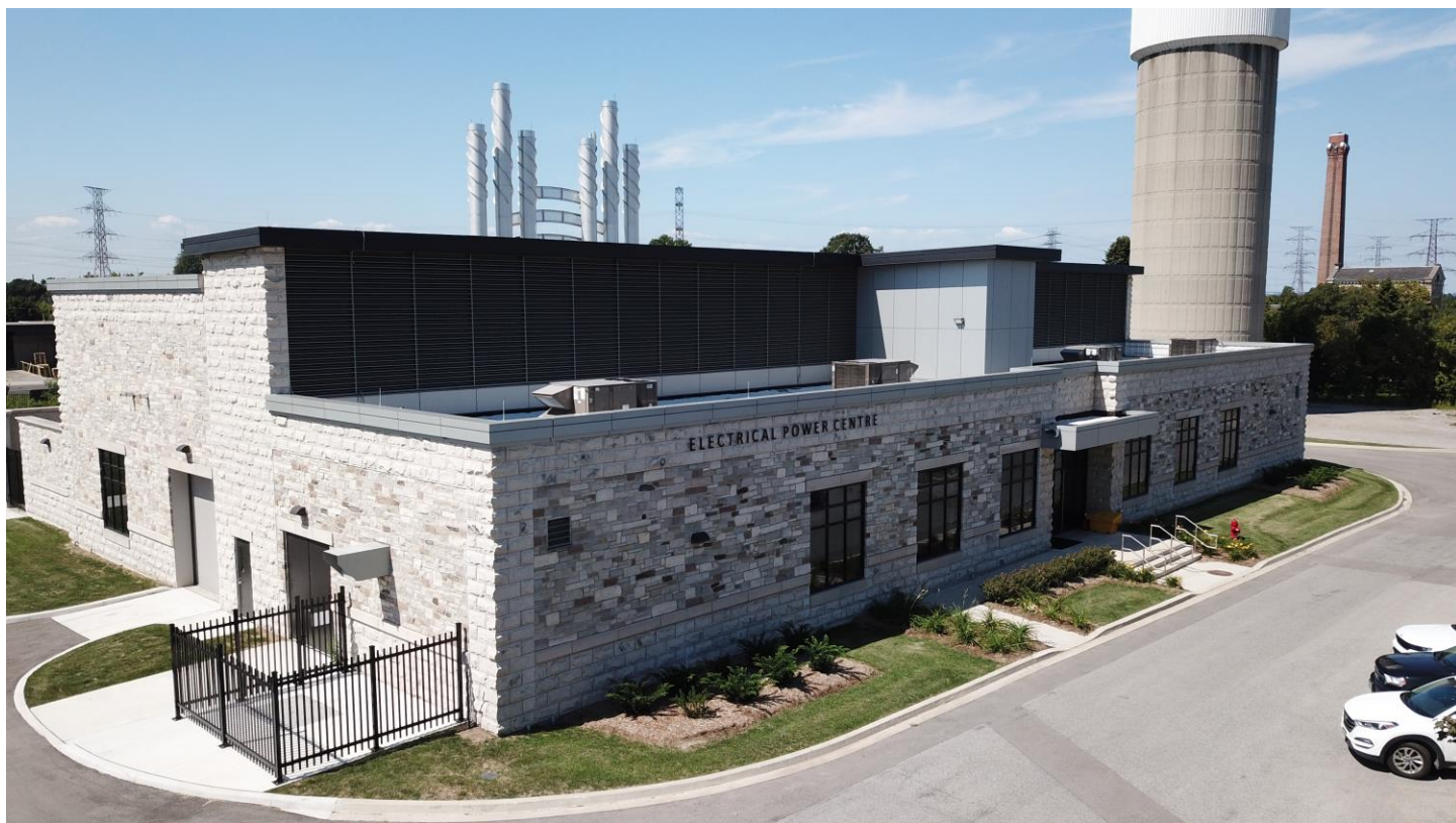
Figure 4: New Electrical Power Centre (Front)
