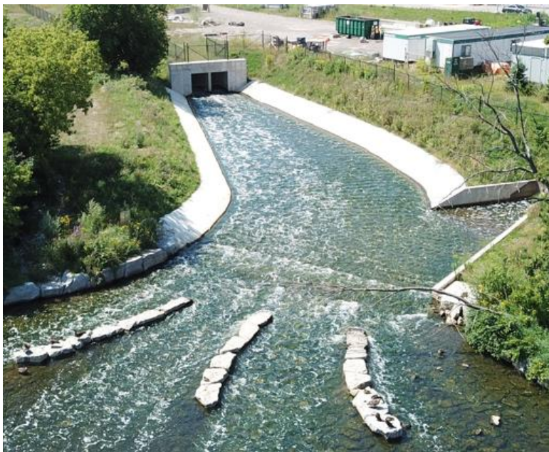
Figure 8: New Outfall & Dissipation Zone
