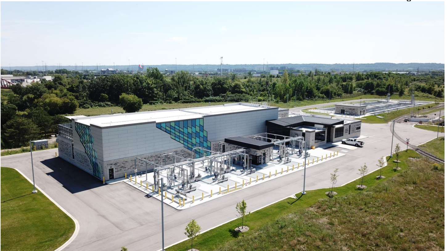
Figure 7: New Tertiary Treatment Facility and Chlorine Contact Tank
