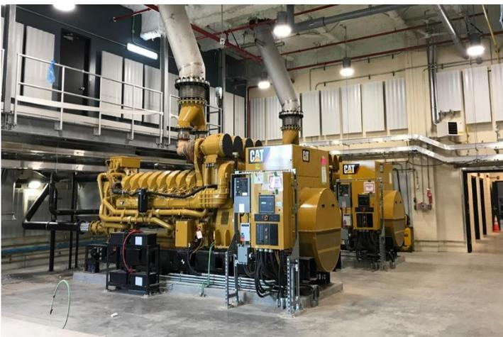
Figure 5: Diesel generators
