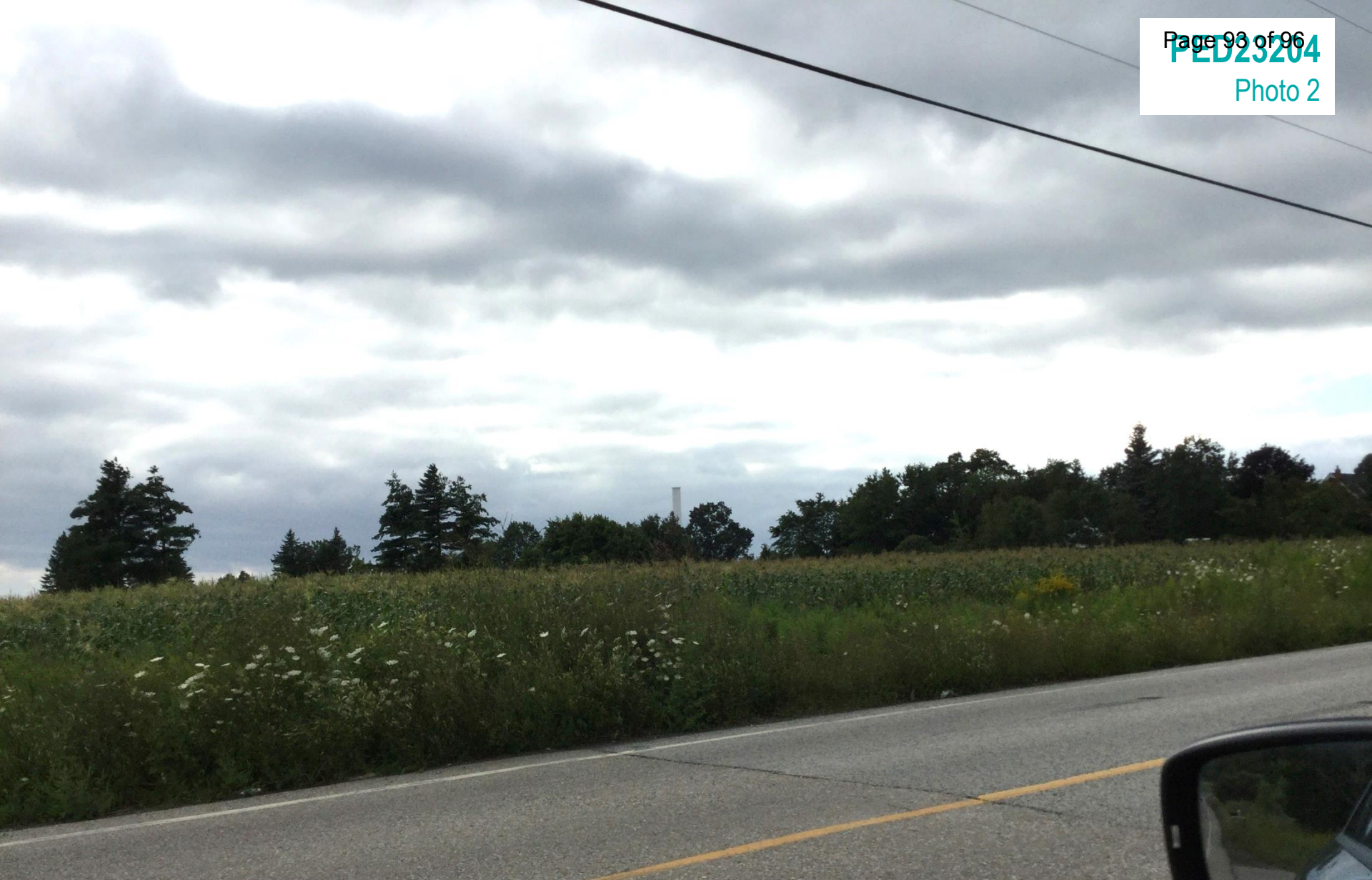
Existing telecommunications tower, as seen from Milborough Line looking north west
