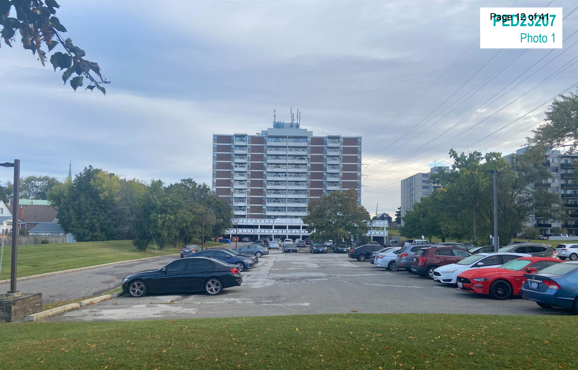
851 Lawrence Road facing north from Lawrence Road
