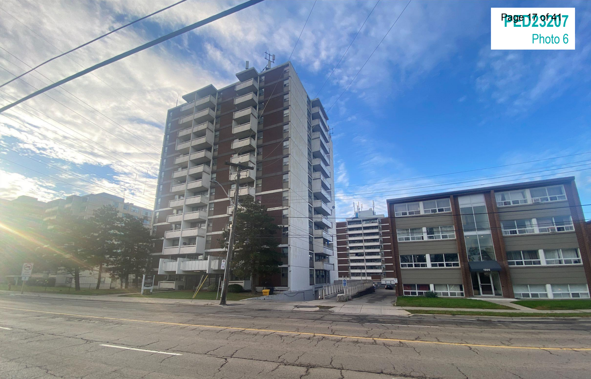
Existing building on Subject Lands at 2030 King Street East facing south
