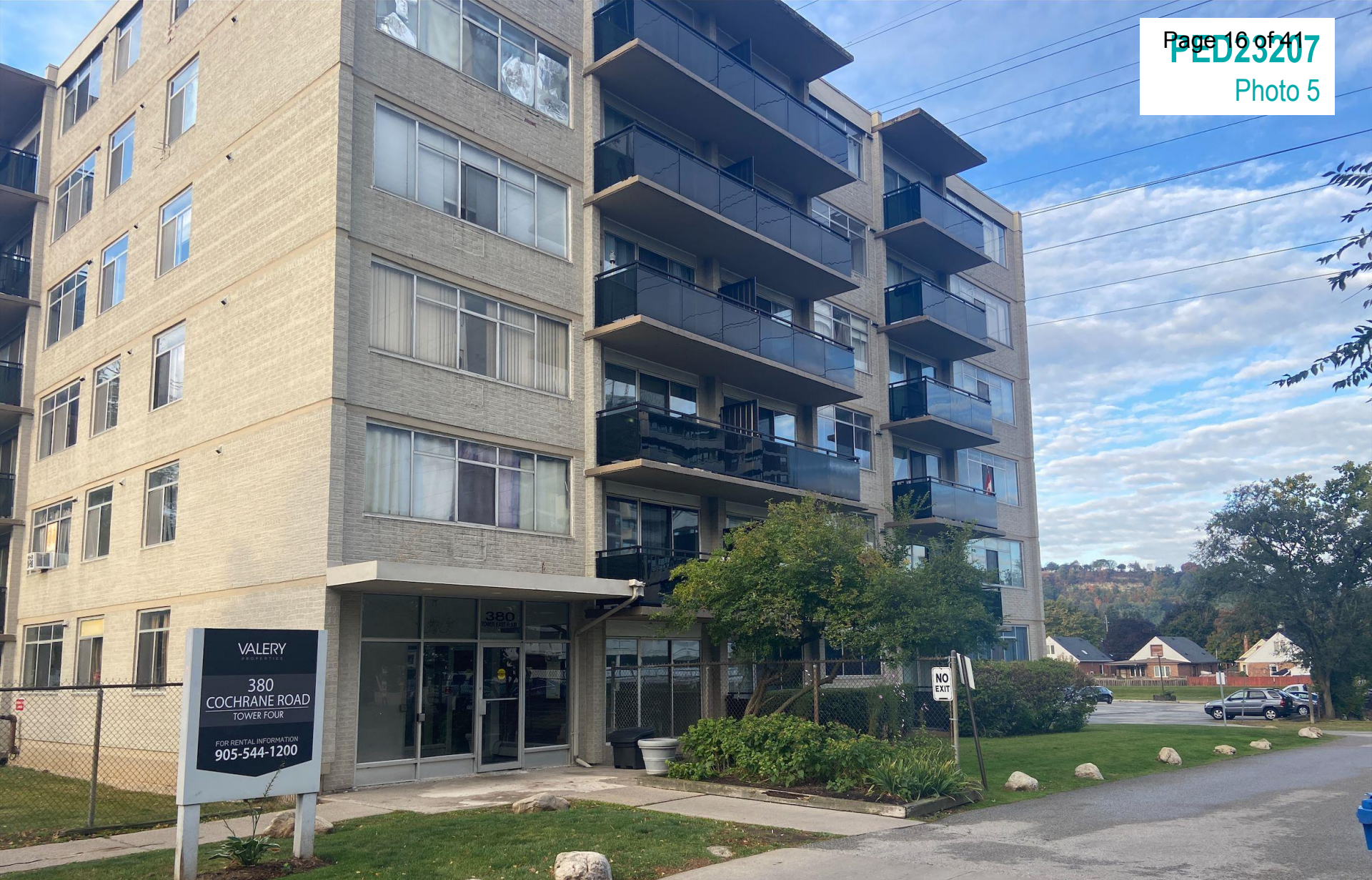
380 Cochrane Road to the east of the hydro corridor facing southwest
