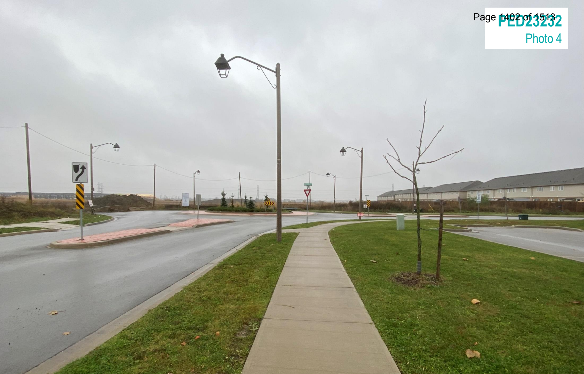
View of roundabout looking south
