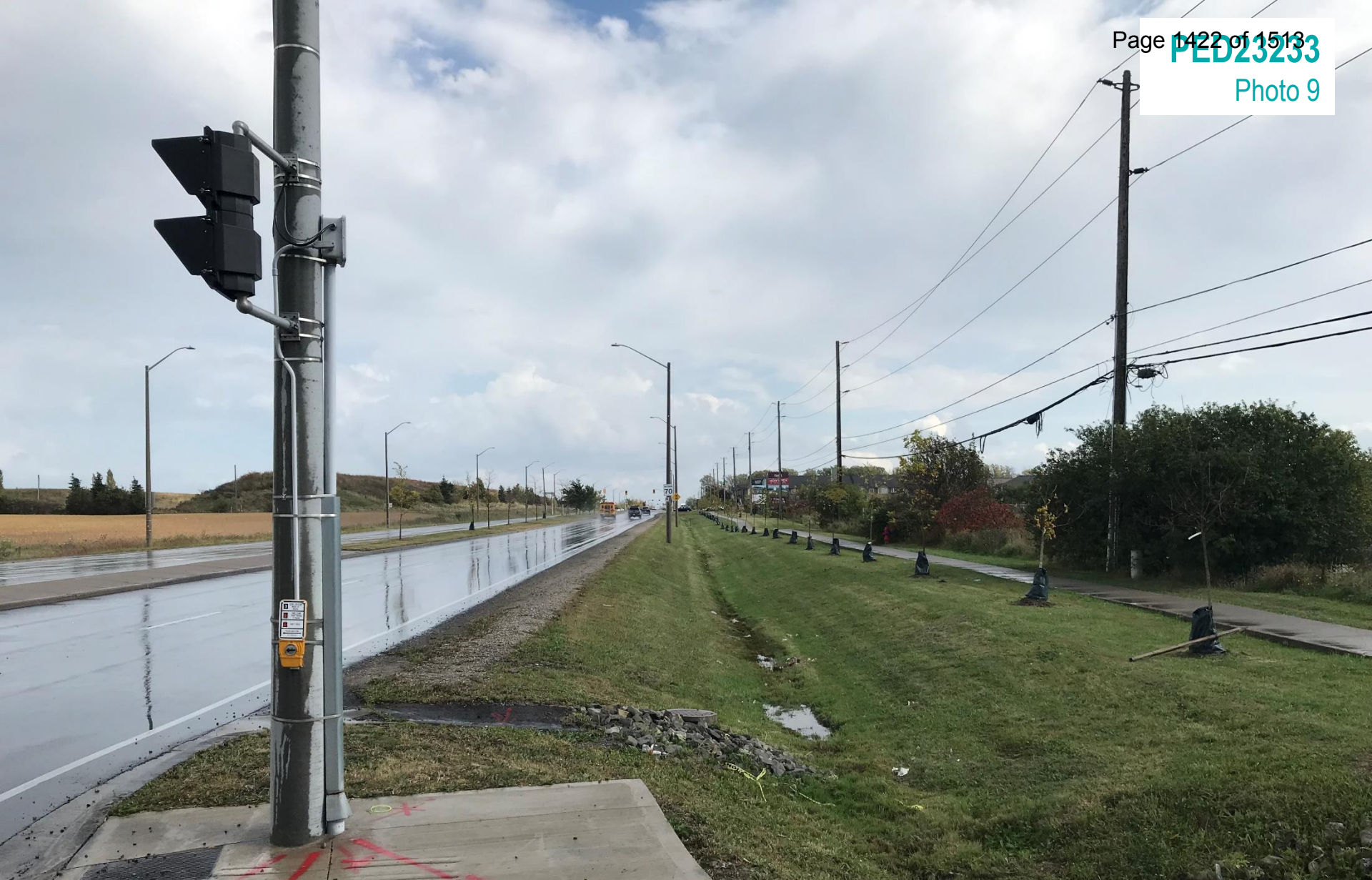
Mud Street West – Looking East
