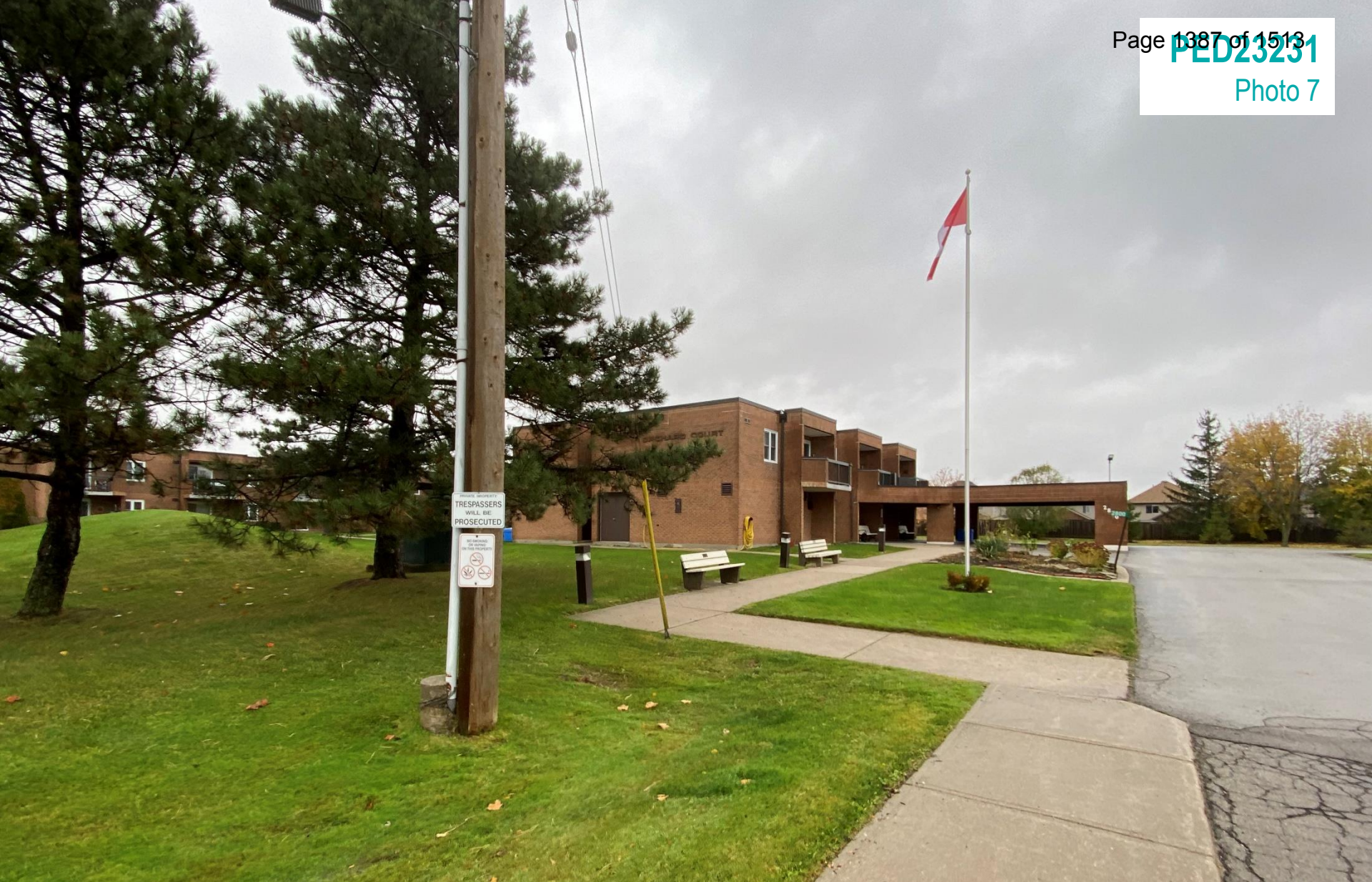
View of existing orchard court seniors residence
