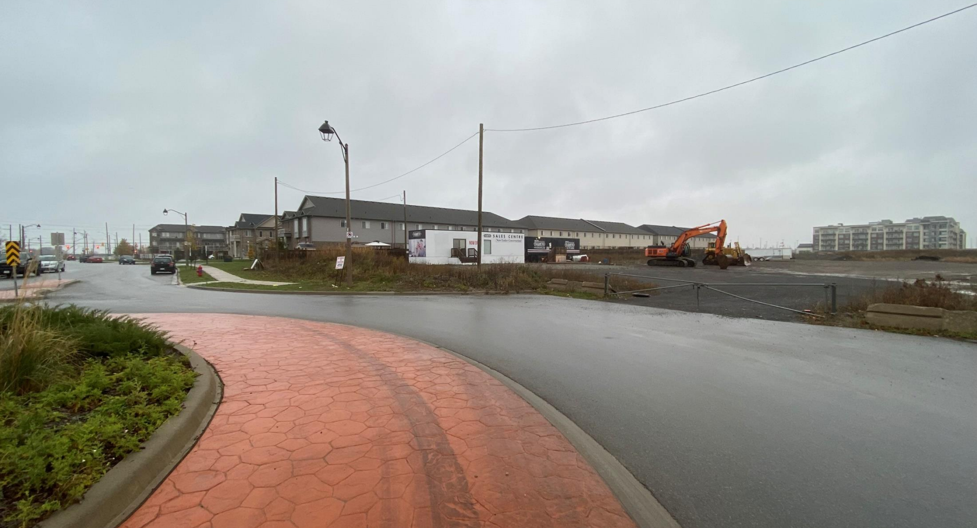
View of NE intersection of Kingsborough Drive and Bellagio Avenue roundabout
