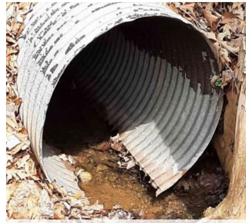
Damaged outfall
