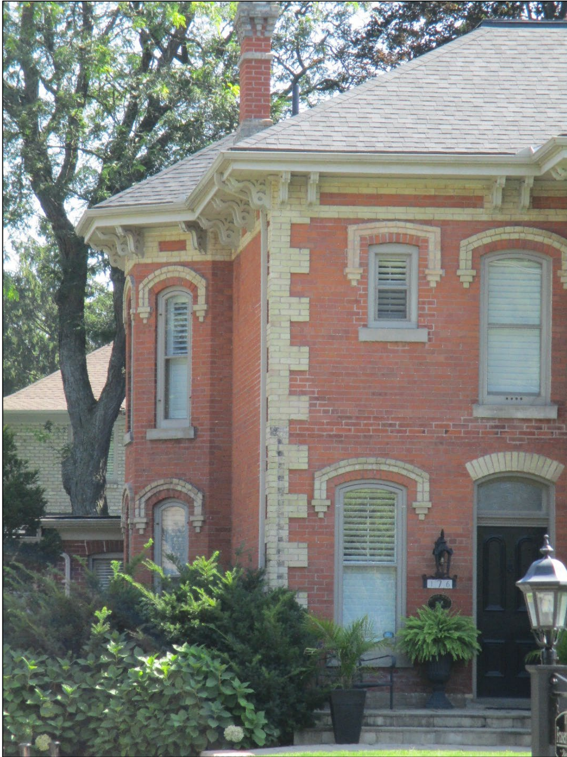
Image 9: Close up showing the projecting bay to the east, the paired brackets below the eave, dichromatic brickwork, wood windows with storms and front door with transom
