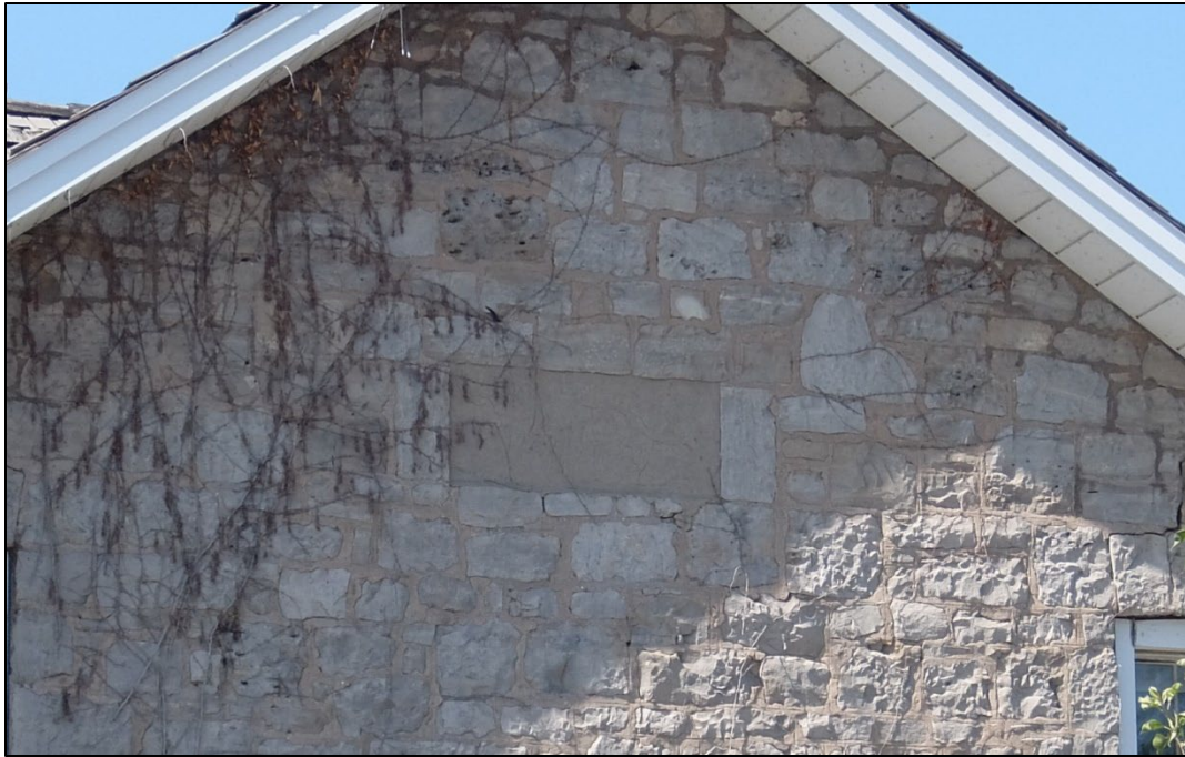
Image 13 and 14: Masonry details of the eastern gable of the south elevation
