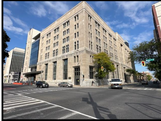
Image 1: View of Southeast Corner (October 18, 2023; Facing Northwest)
