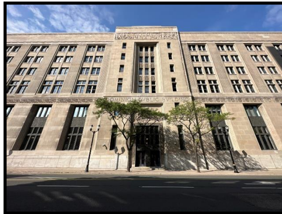
Image 2: View of East Elevation (October 18, 2023; Facing West)
