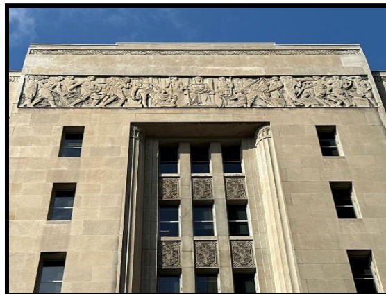
Image 3: Detailed View of East Elevation (October 18, 2023; Facing West)
