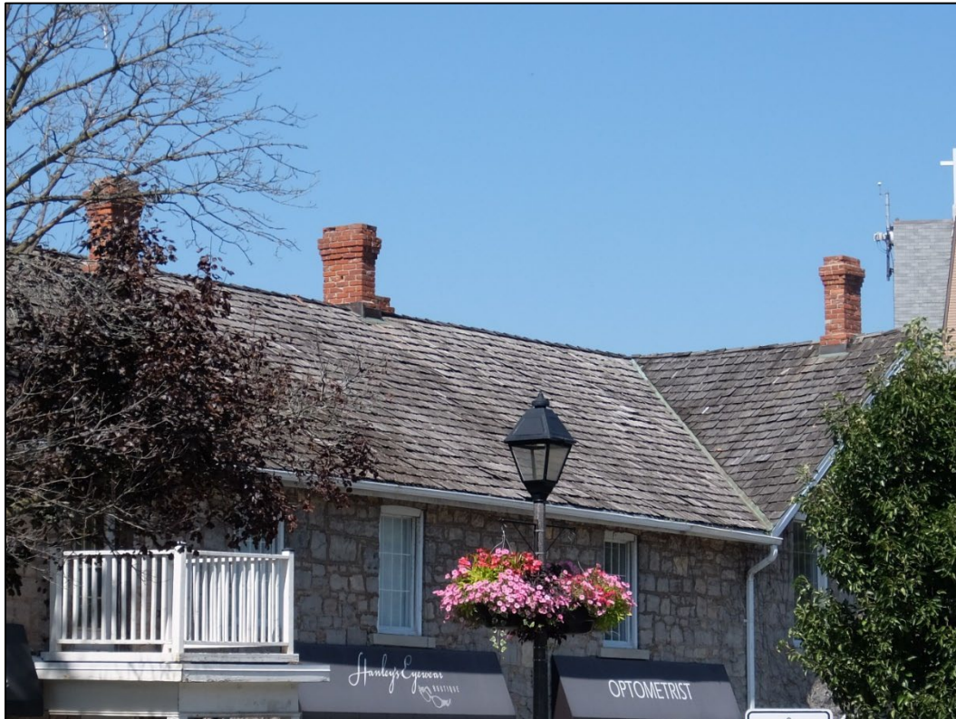
Image 12: Roofline detail on south elevation
