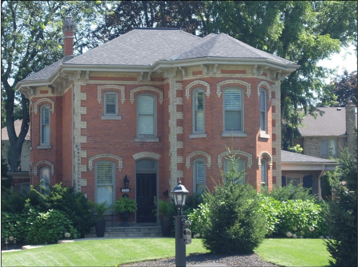
Image 2: Front (northern) elevation, from the east, showing the projecting bay in the side (east) elevation
