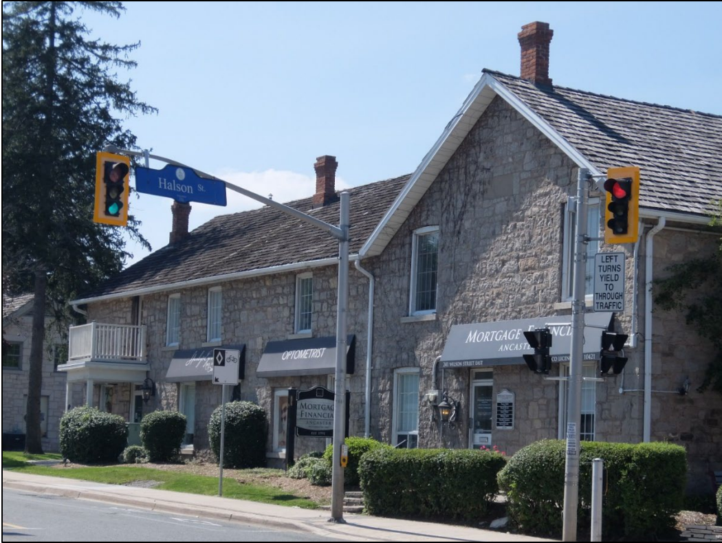
Image 5: South elevation of property
