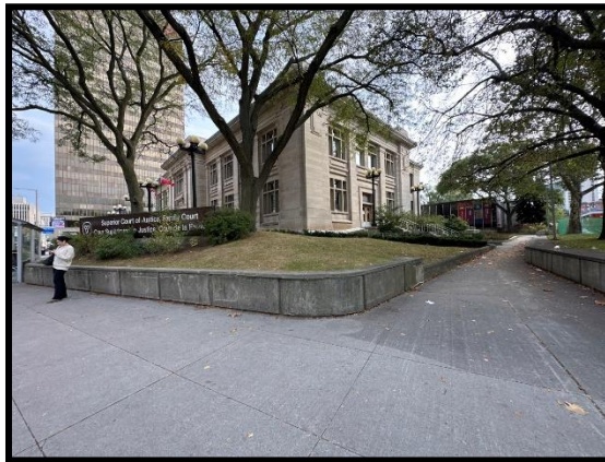
Image 2: View of Northwest Corner (October 18, 2023; Facing Southeast)
