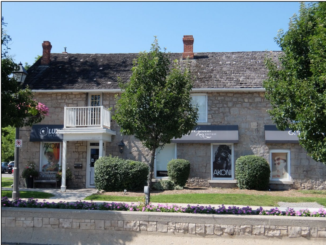
Image 6: West end of south elevation
