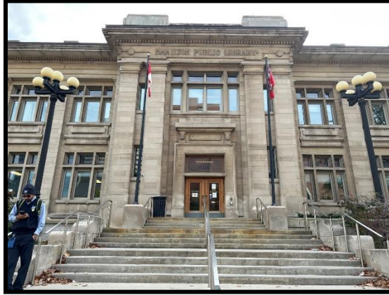
Image 1: View of Façade (October 18, 2023; Facing South)
