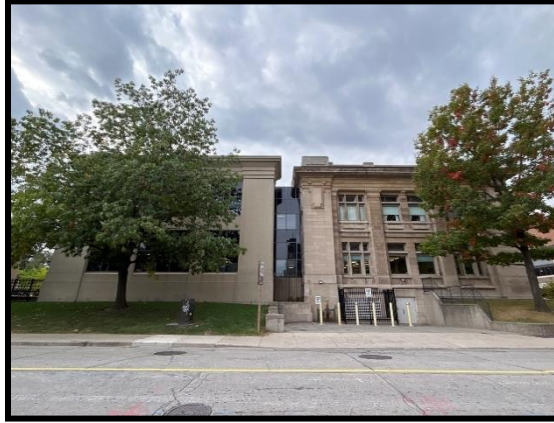
Image 4: View of East Elevation and Addition (October 18, 2023; Facing West)
