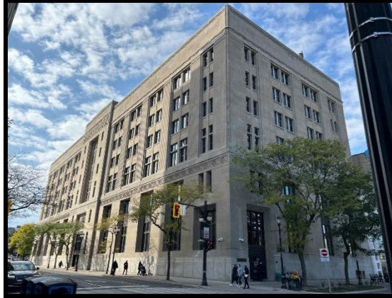
Image 4: Northeast Corner (October 18, 2023; Facing Southwest)
