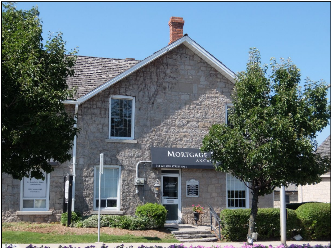
Image 8: Close up of east end of south elevation
