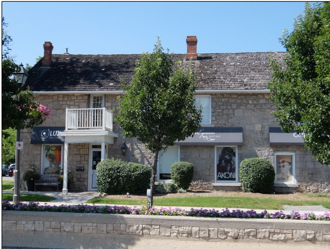
Image 6: West end of south elevation
