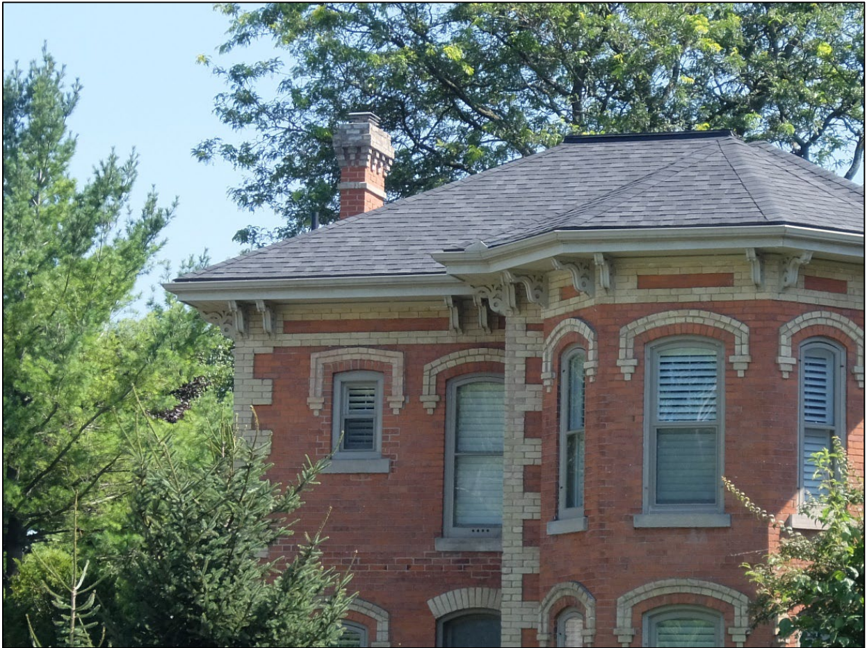
Image 6: Detail of chimney and truncated hip roof
