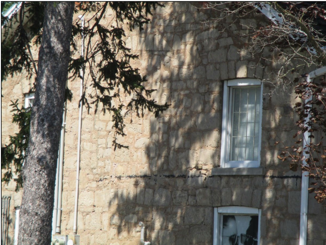
Image 10: Masonry detail on west elevation
