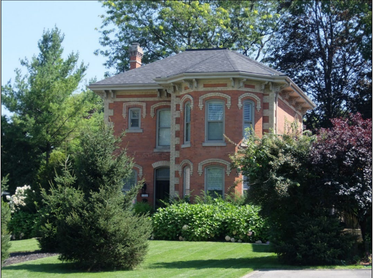
Image 1: Front (northern) elevation, from the west
