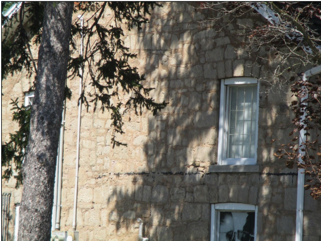
Image 10: Masonry detail on west elevation
