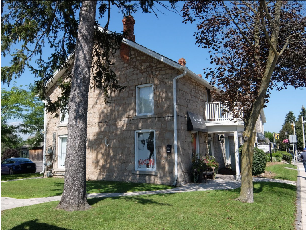
Image 4: Detail of west elevation and yard
