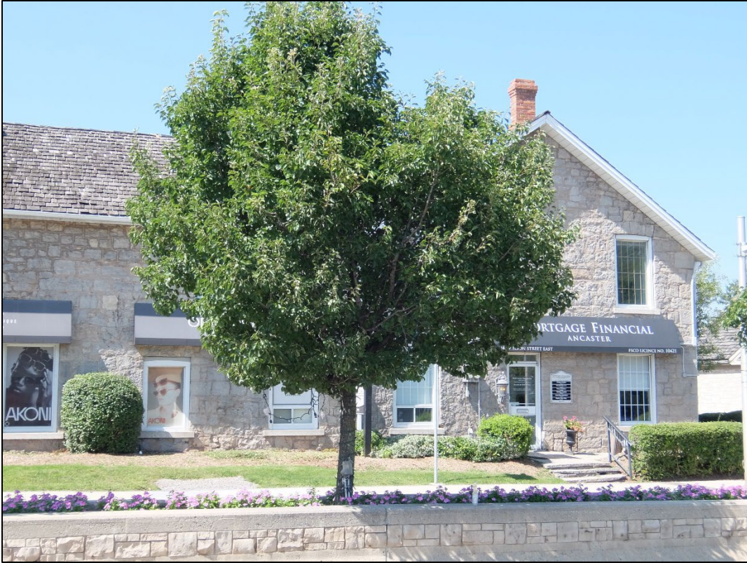
Image 7: East end of south elevation
