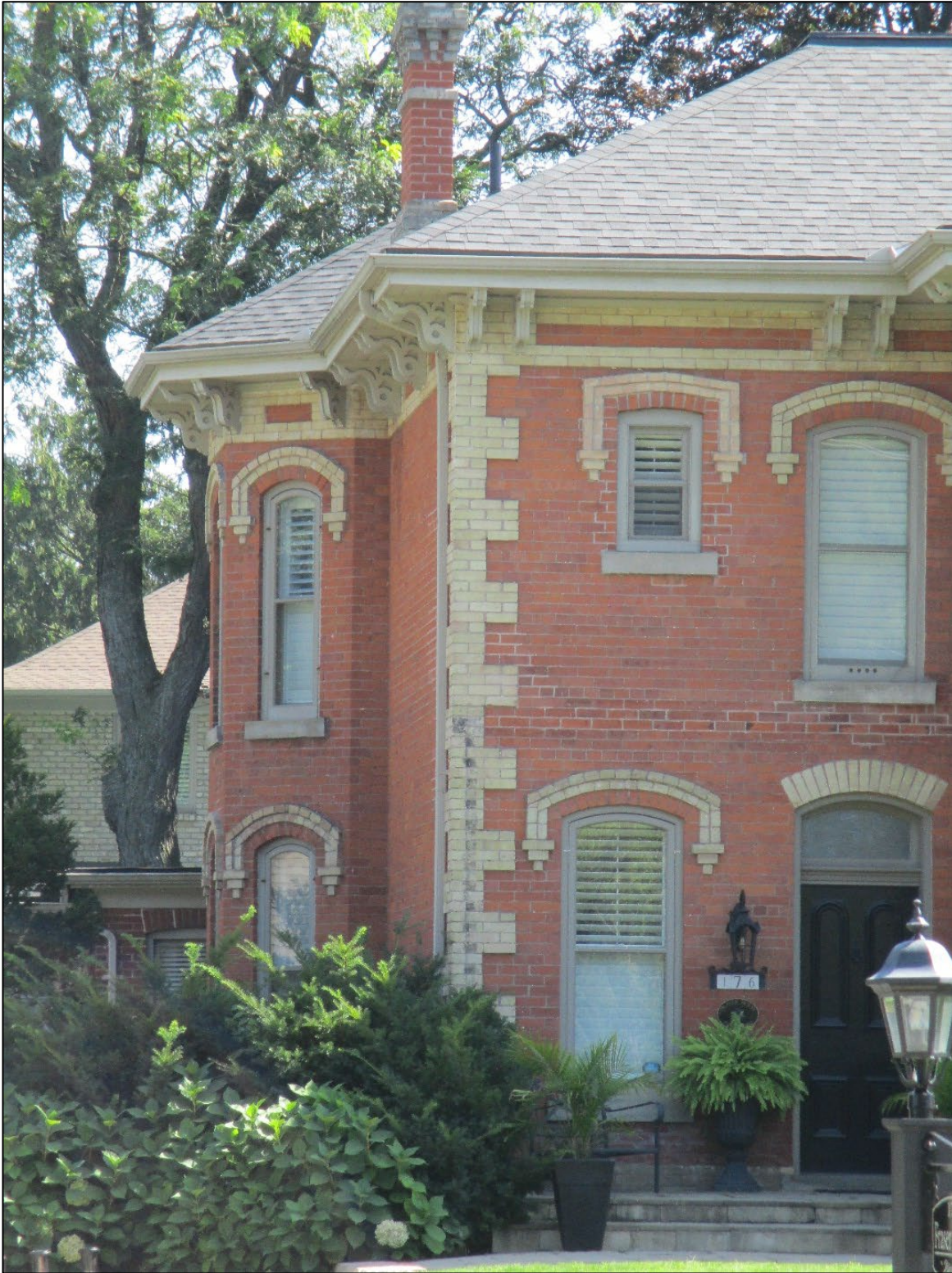
Image 9: Close up showing the projecting bay to the east, the paired brackets below the eave, dichromatic brickwork, wood windows with storms and front door with transom
