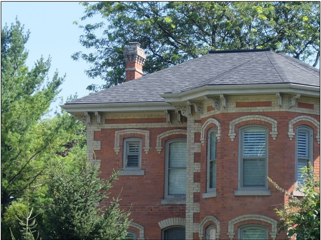
Image 6: Detail of chimney and truncated hip roof
