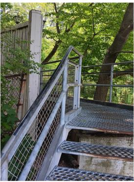
**Blind Corner:** At the bottom of the stairs, there is a blind corner. This is a safety hazard due to low lighting and restricted visibility by way of a wooden fence. **Street Crossing:** Access to the James Street Stairs requires users to jaywalk across James St. S.
