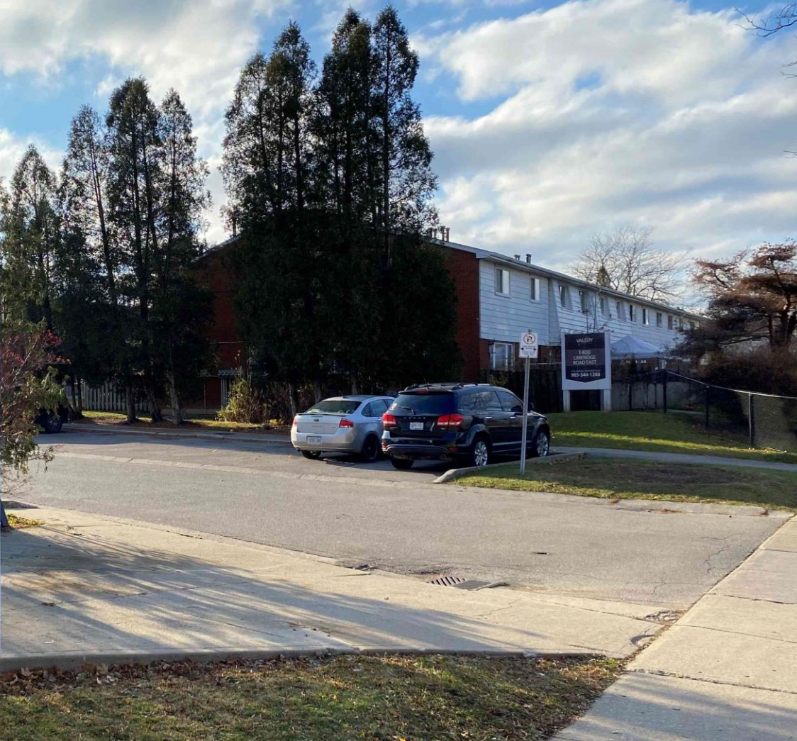
Subject lands from Limeridge Road East facing southwest
