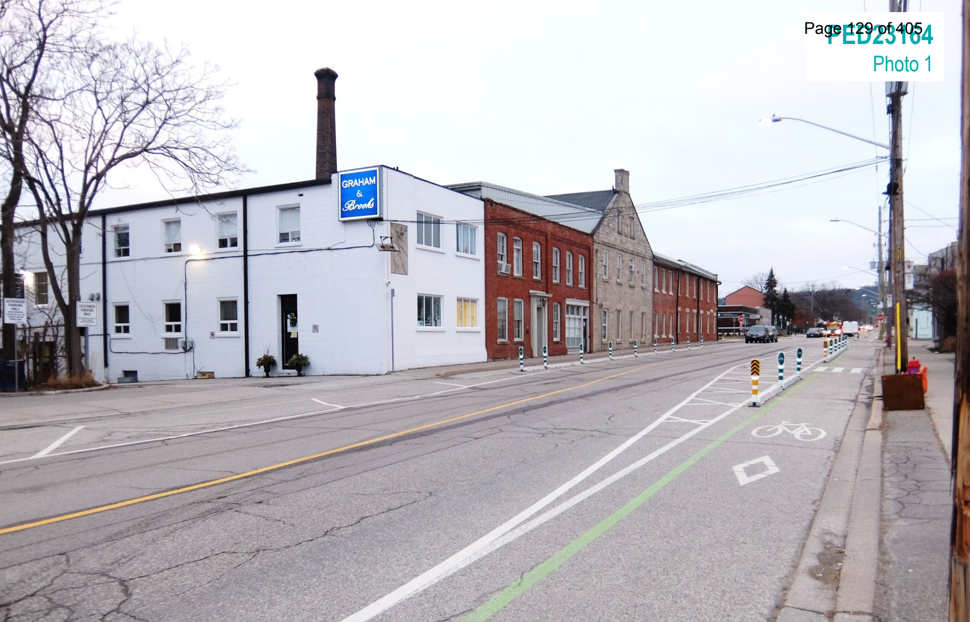
Looking south west at the subject property, from Hatt St
