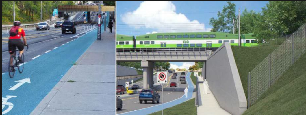
EXAMPLE: GO EXPANSION PROJECTS Accommodating planned municipal bike lanes as part of a grade separation project.
