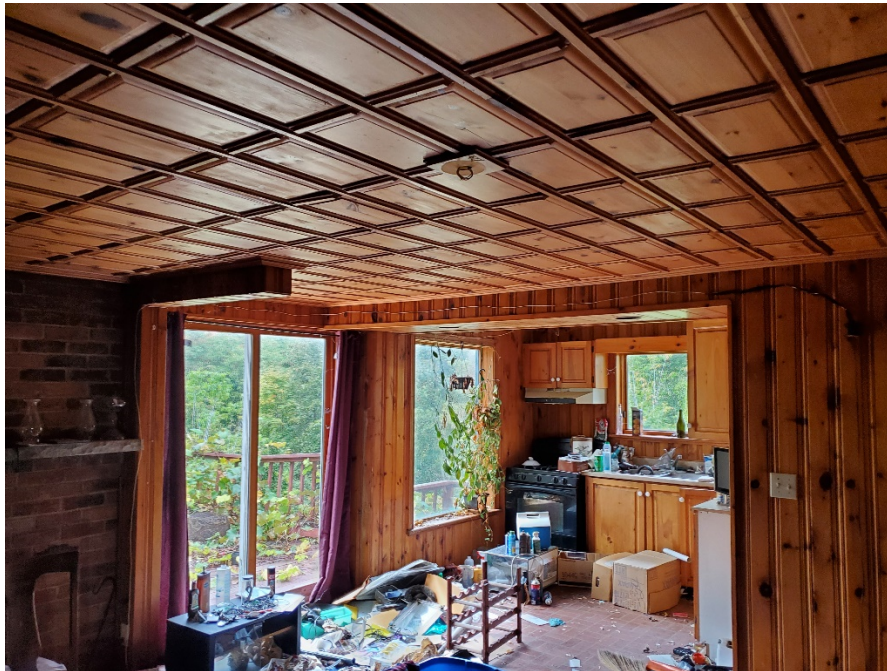
Photo No 02: North Kitchen Wall below Photo No:01
