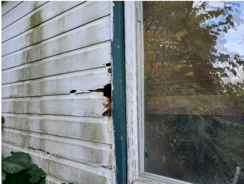
Photo No 06: Rotted Siding
