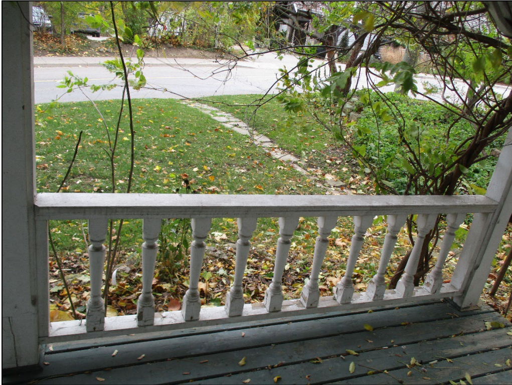
Figure 21: View of turned railings on front porch
