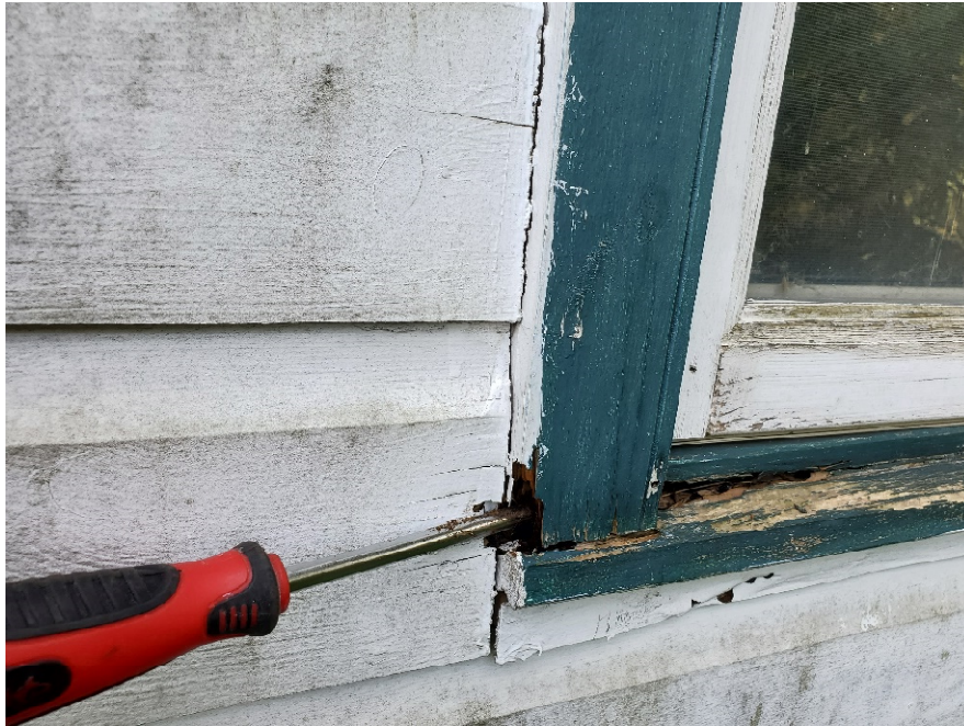
Photo No 07: Rotted Sill
