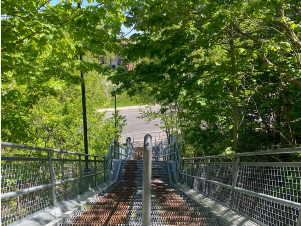
Overhanging trees should be cleared as well as vegetation growing through the grates, through the sides, and over the handrails.
