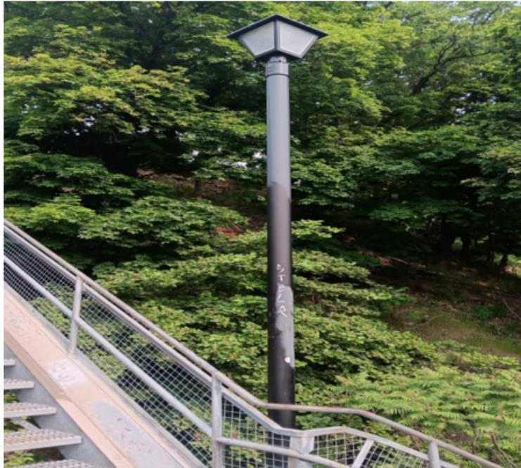
Many lights along these stairs are being impeded by vegetation (below), blocking the beam and darkening the area. Vegetation should be aggressively removed from light standards and fixtures.
