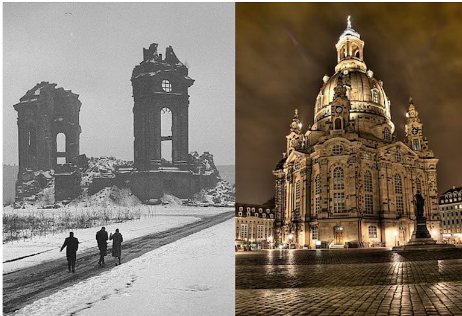
Frauenkirk Dresden, before and after
