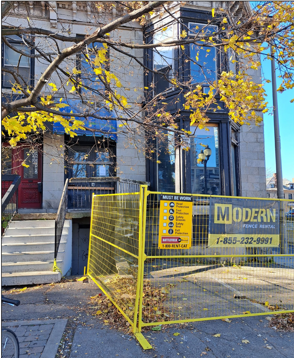
Front (east) elevation of 54 Hess Street South showing the safety fencing in place
