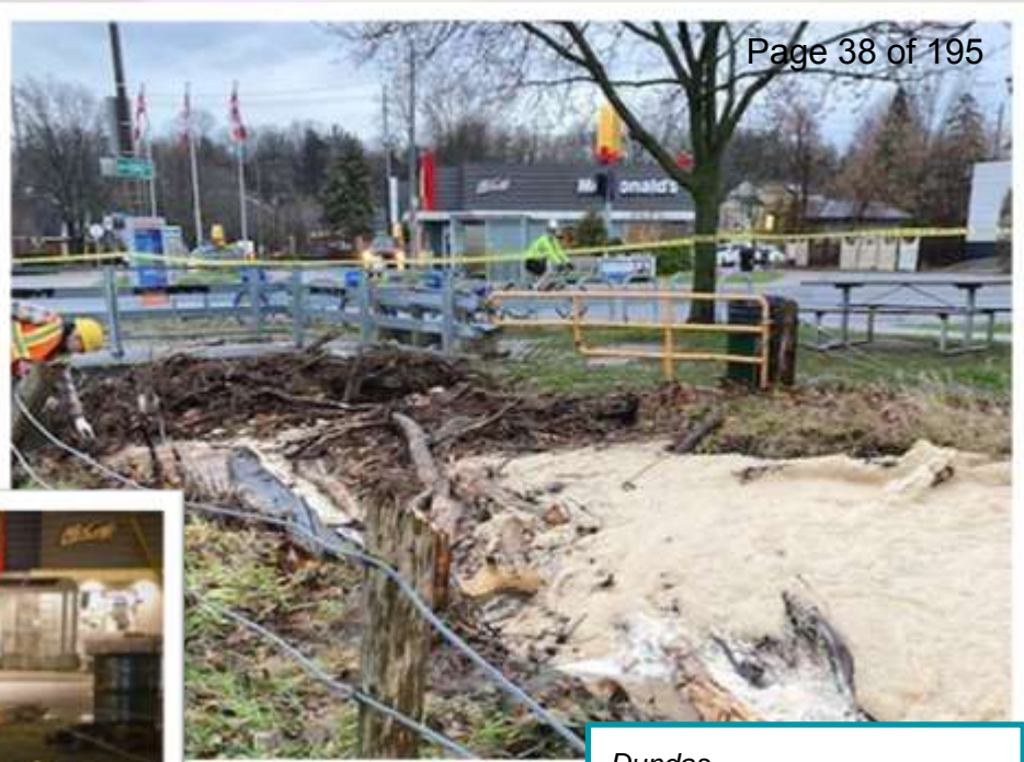
Dundas Box Culvert plugged - Sydenham Creek 2021 Dundas Star
