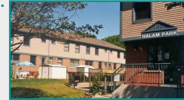
Halam Park Co-op 85 Halam Ave. 102 units
