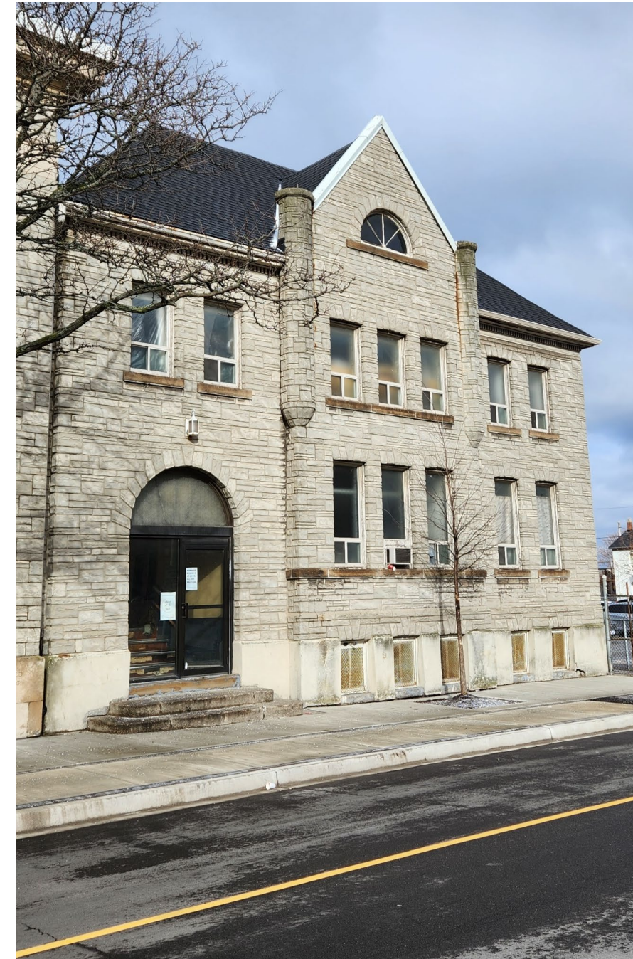
1901 façade covered with cement-based mortar
