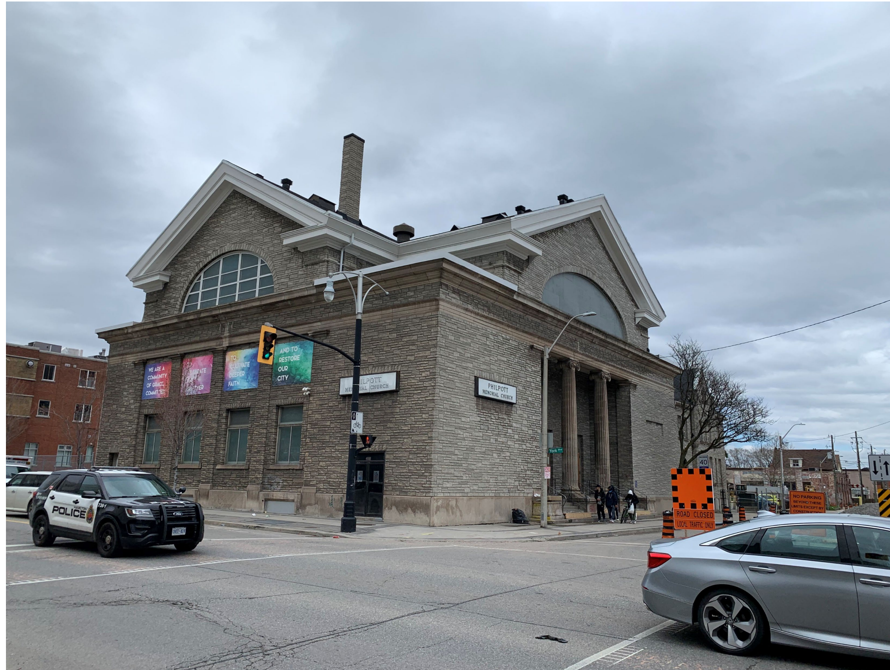
1906 façades covered with cement-based mortar
