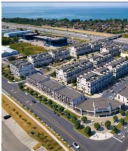
1290 South Service and Vince Mazza Way
