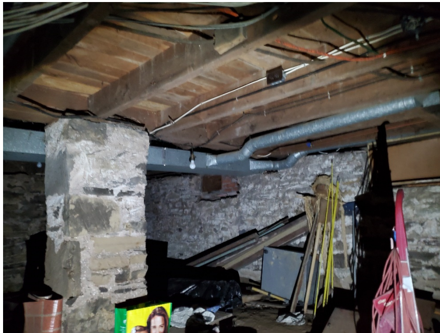
Photo No 03: Main Floor Framing (Original House)
