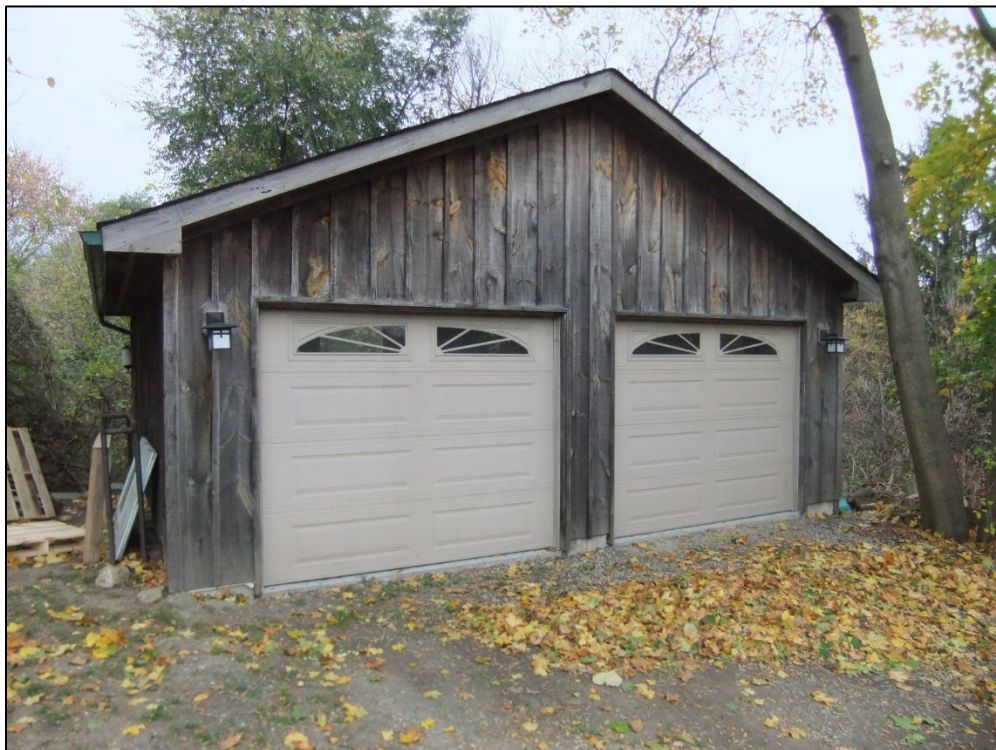
Figure 4: View of existing contemporary side garage
