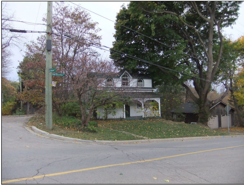
Figure 1: View of Front (East) Elevation facing Old Dundas Road
