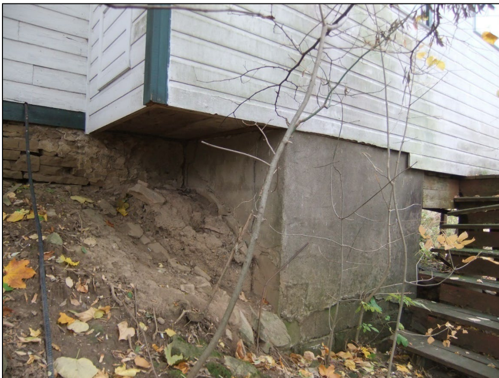
Figure 12: View of contemporary side addition and foundation
