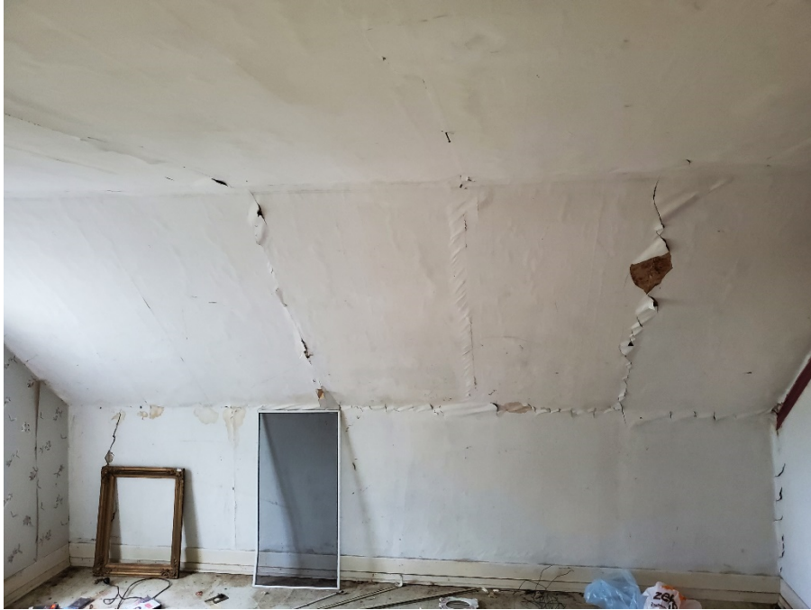
Photo No 01: 2 nd Floor North Wall above Kitchen
