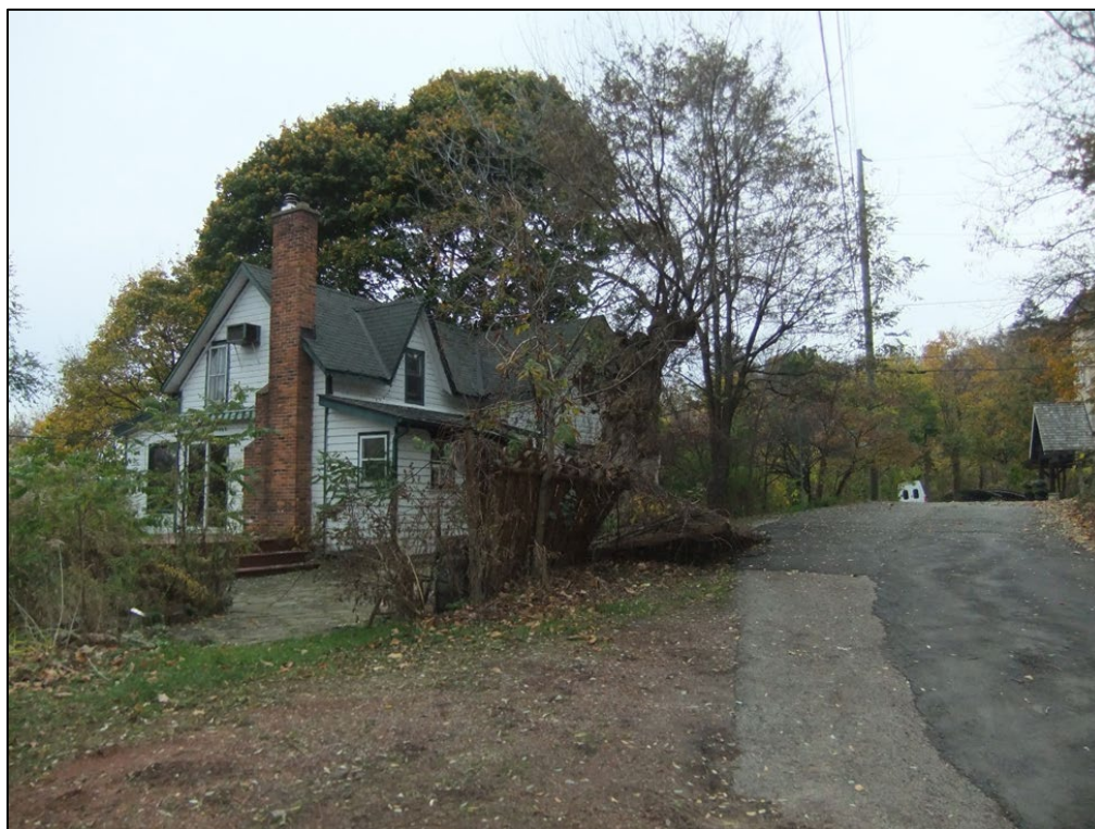
Figure 2: View of South Elevation along Ontario Road
