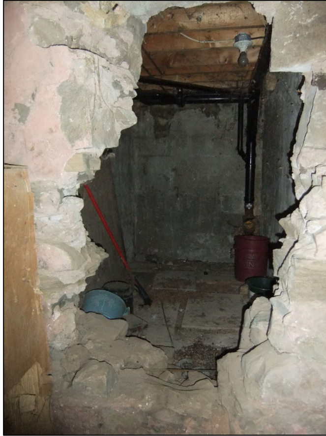
Figure 15: View of foundation wall in basement, looking into side addition
