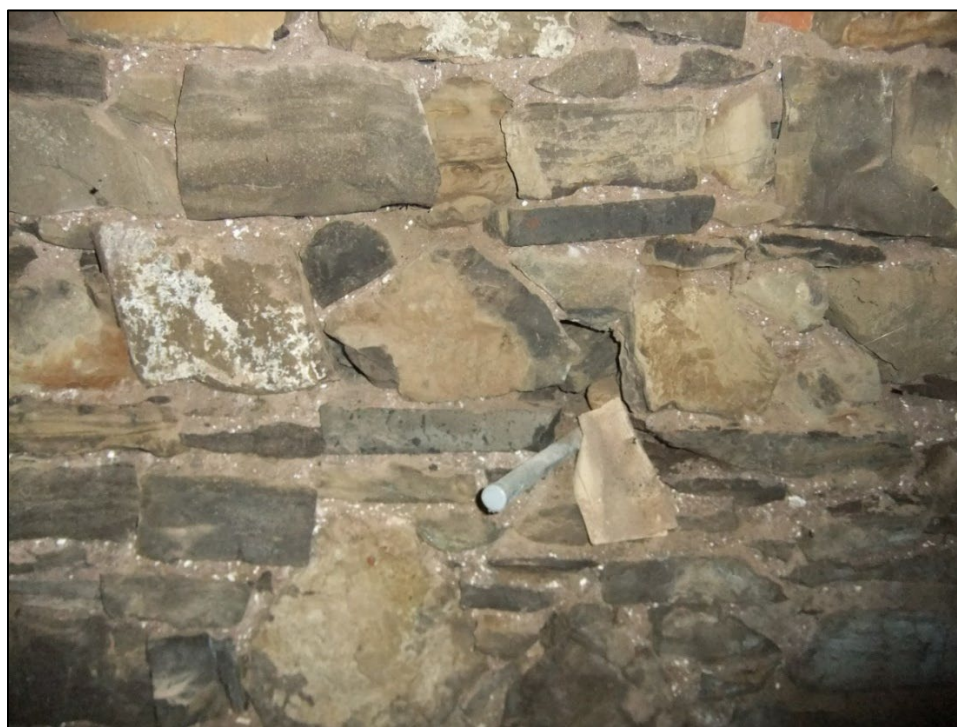
Figure 14: View of stone foundation wall in basement
