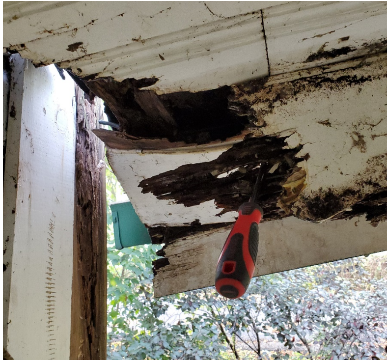
Photo No 05: Rotten Wood
