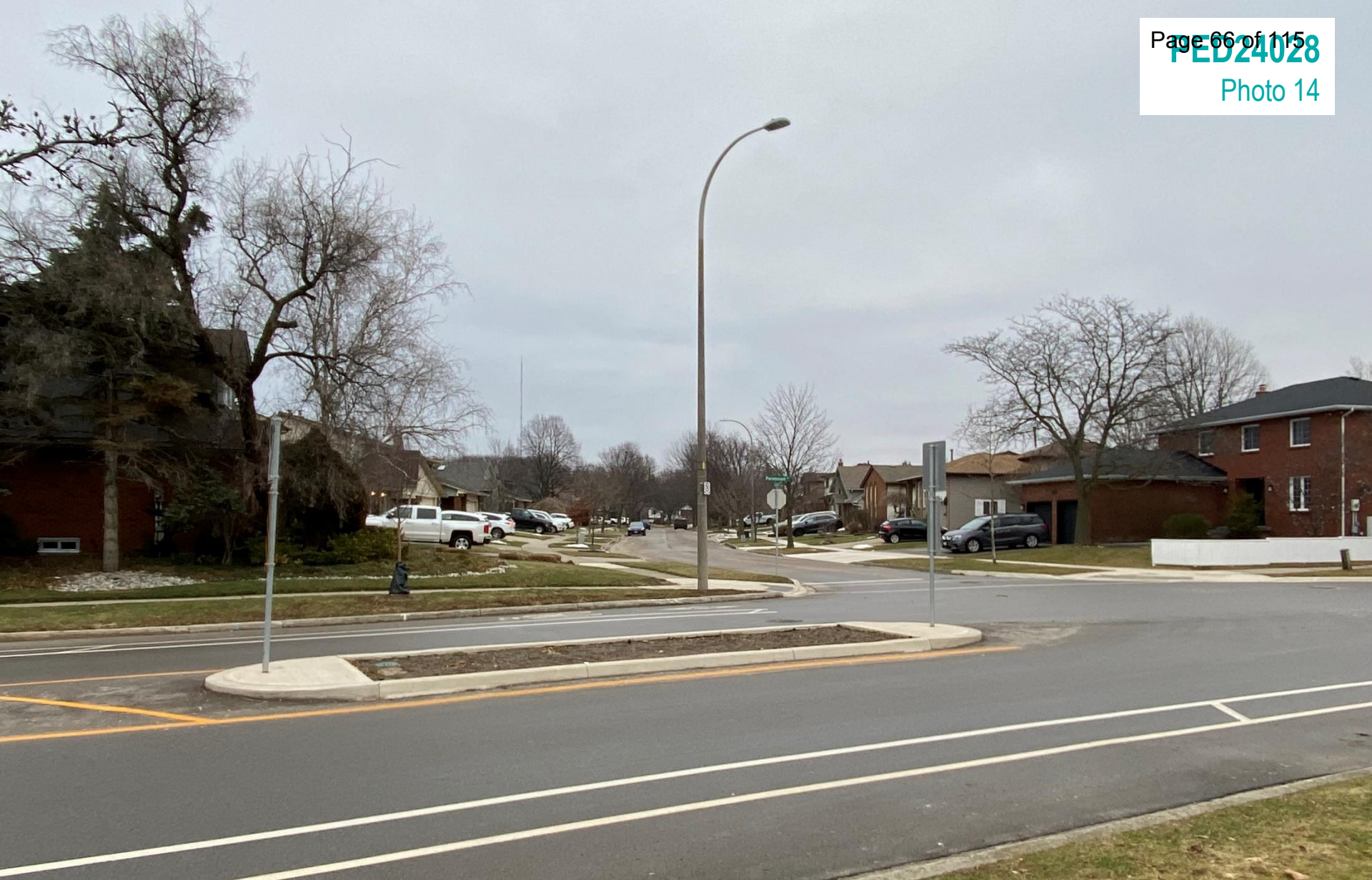
Looking east towards Ackland Street
