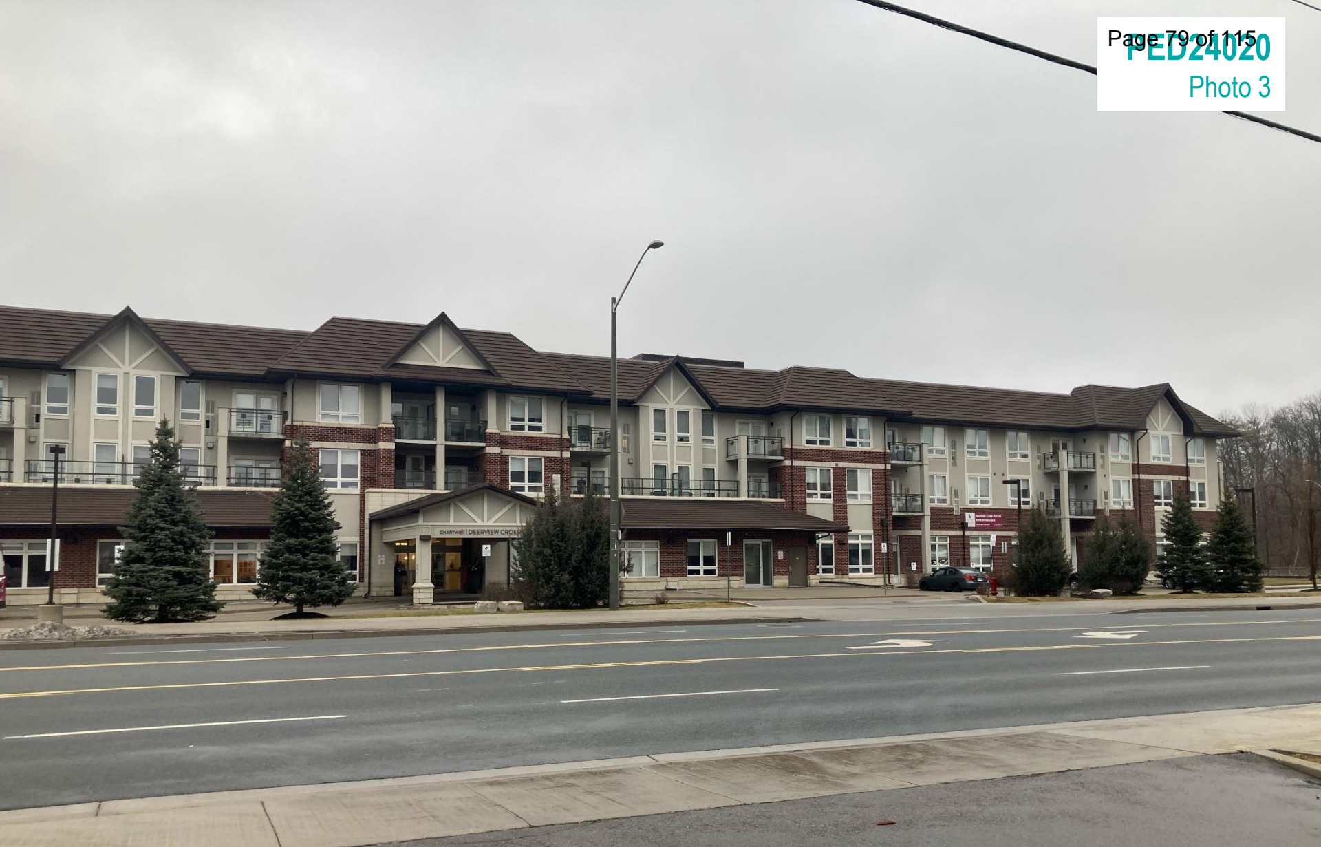
North side of Rymal Road West
