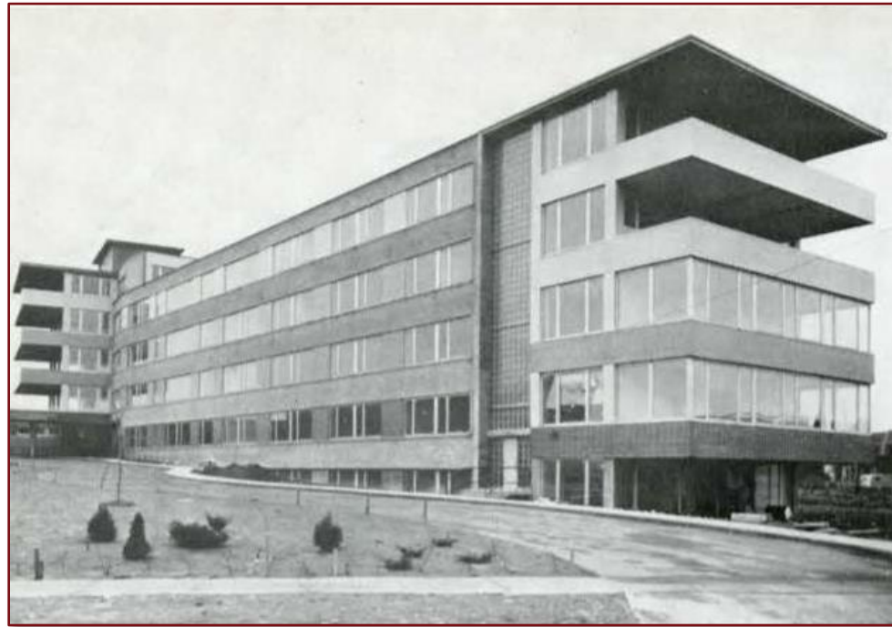
Image 15: Main Entrance to the Convalescent Hospital
