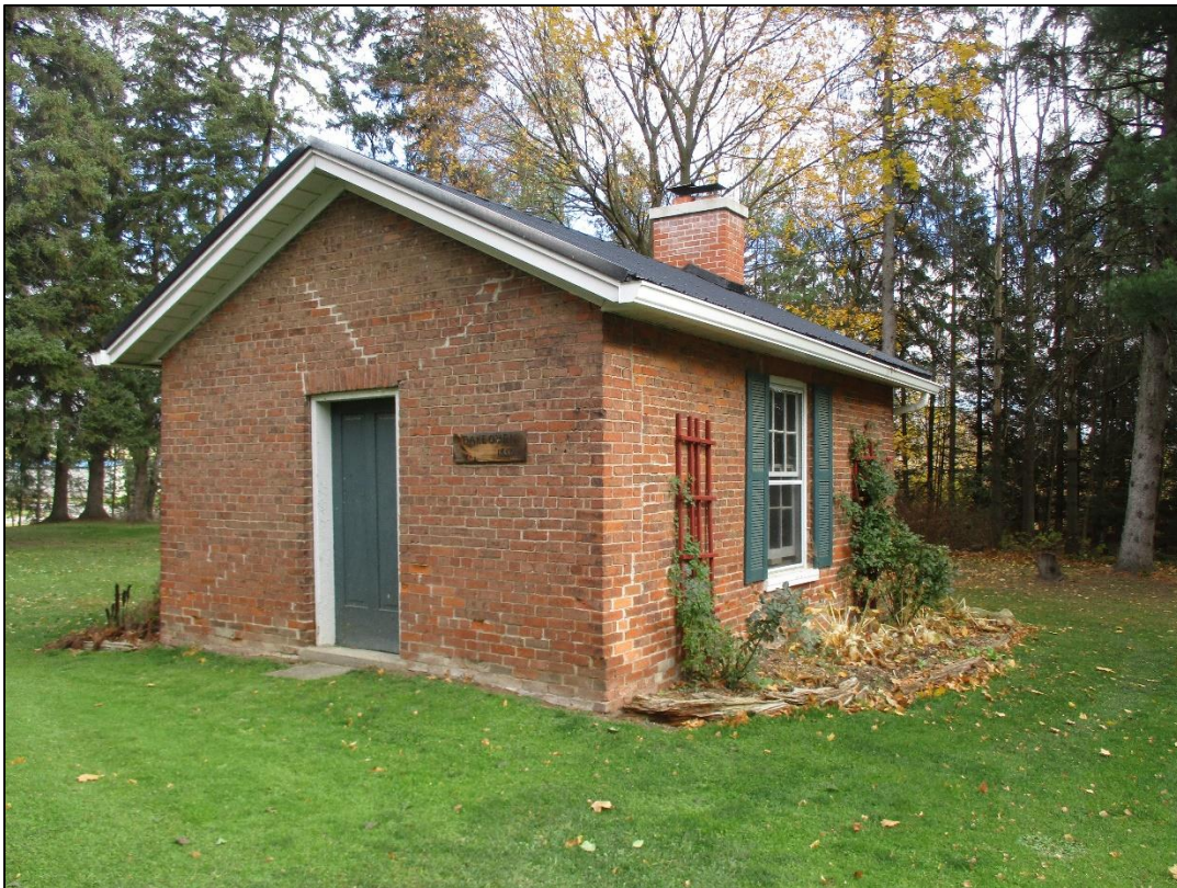
Figure 20: View of c.1856 bakehouse
