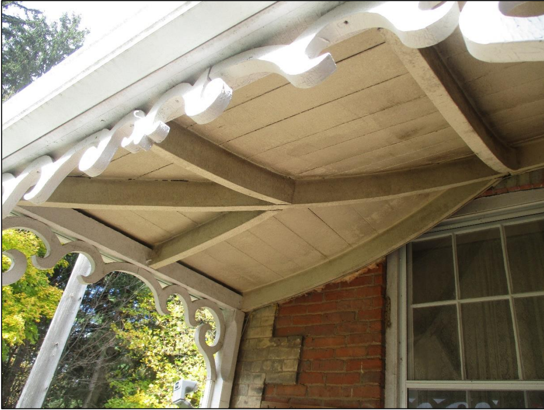
Figure 13: Detail of west side farmhouse porch
