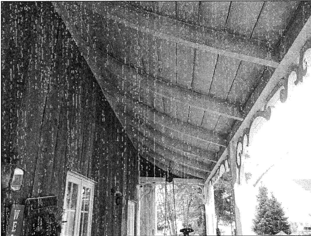
Figure 14: Detail of west side farmhouse porch
