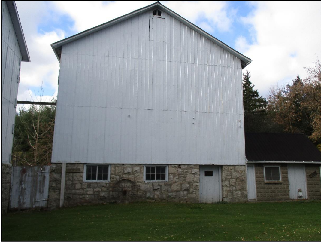
Figure 29: East Elevation of Dairy Barn
