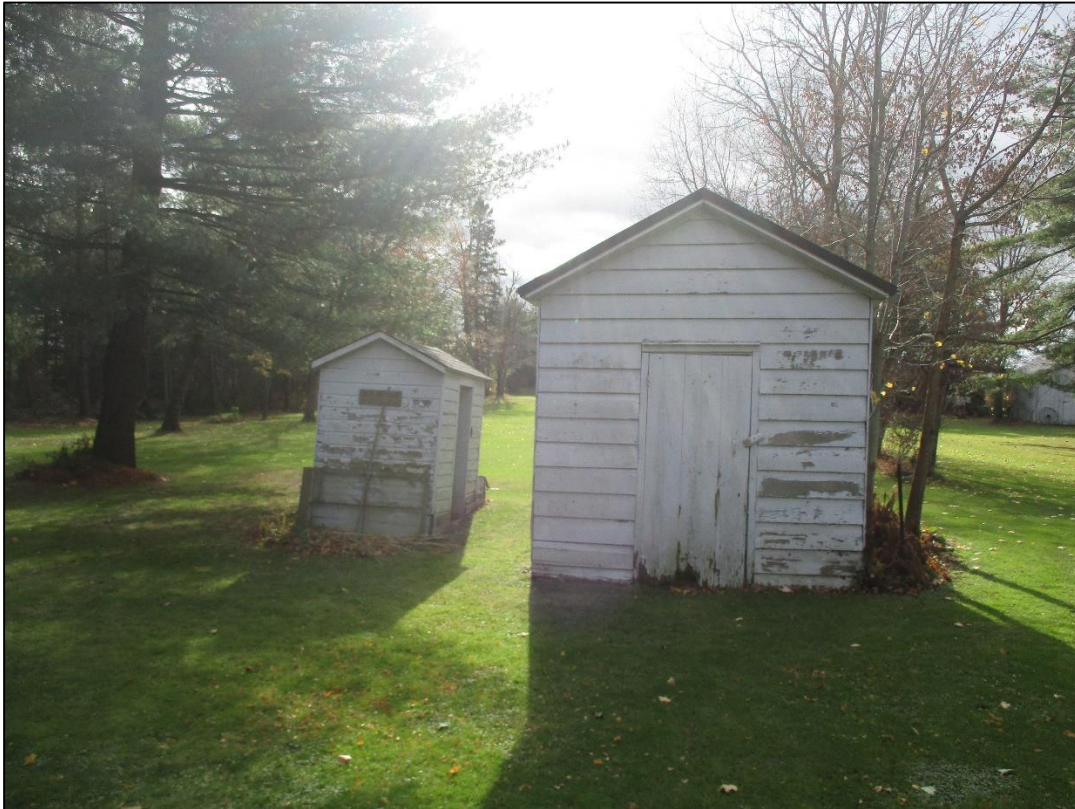
Figure 24: North Elevations of outhouse (right) and smokehouse (left)
