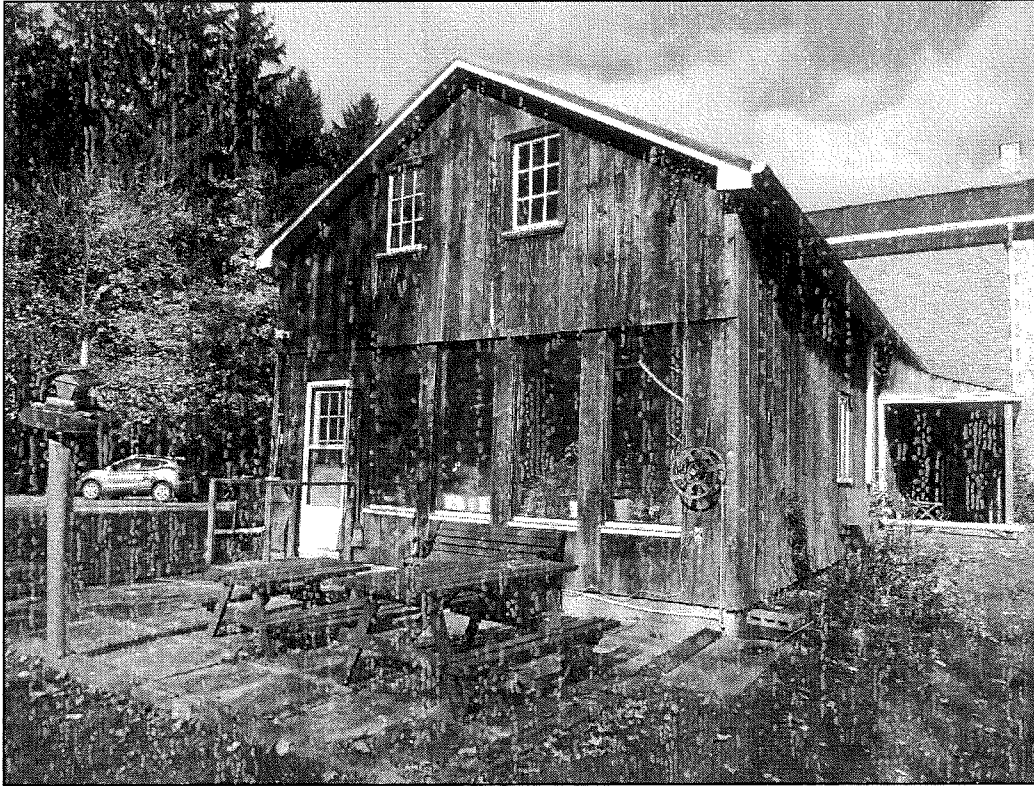
Figure 5: Rear (South) Elevation of Farmhouse
