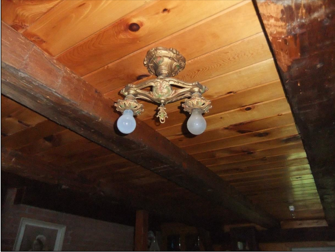
Figure 35: Interior View of farmhouse showing hand hewn beams
