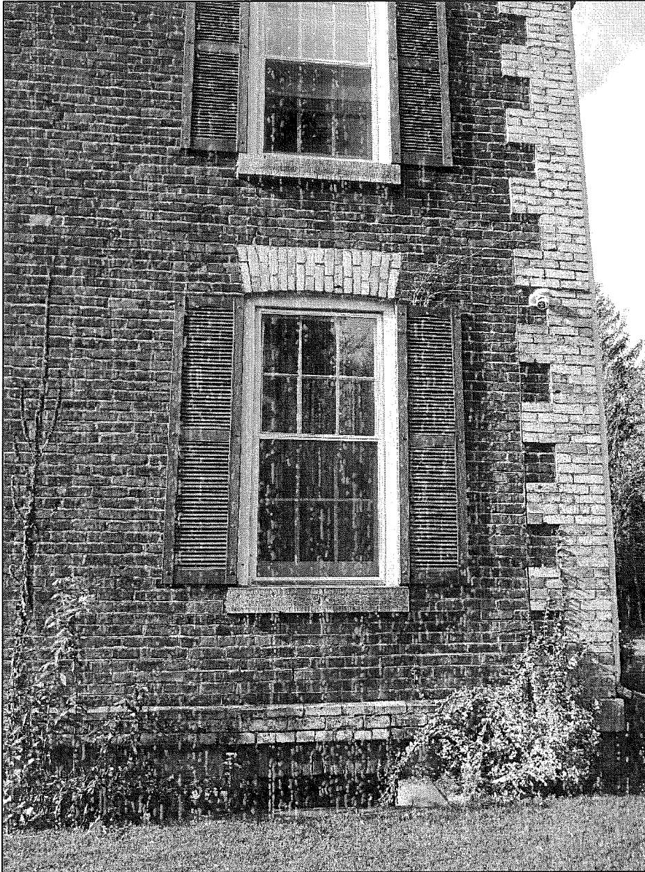
Figure 9: Detail view of windows, stone foundation, and projecting quoins
