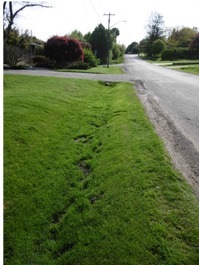
PHOTOGRAPH 6: EXAMPLE TYPE 'D' DRAINAGE FEATURE
