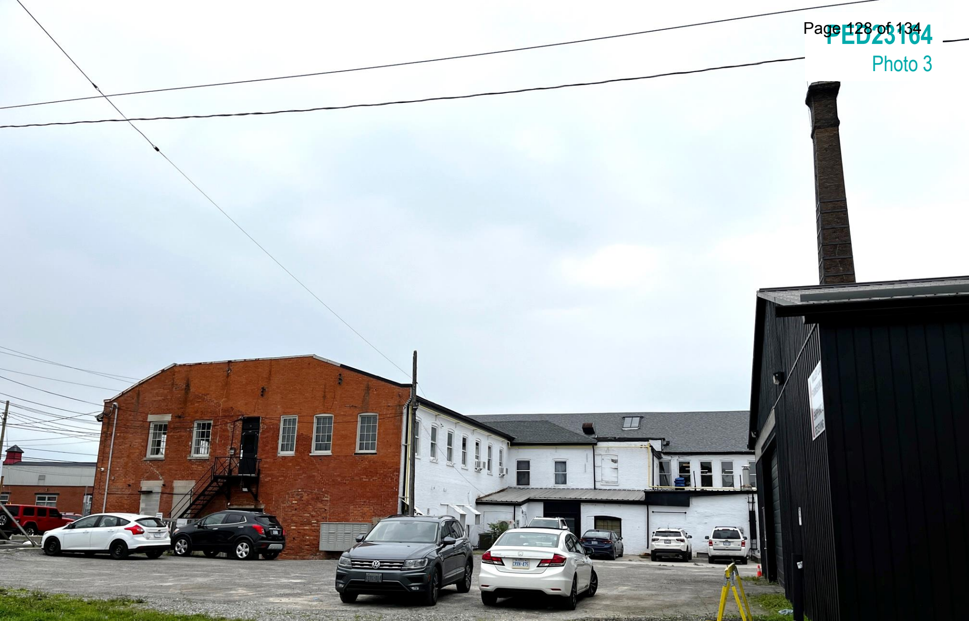
Looking West at the subject property, from McMurray St
