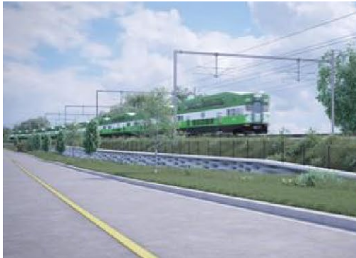
GO Expansion On-Corridor Works
