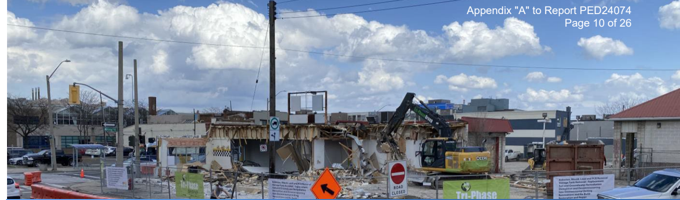
Demolition at King and Wentworth Streets
