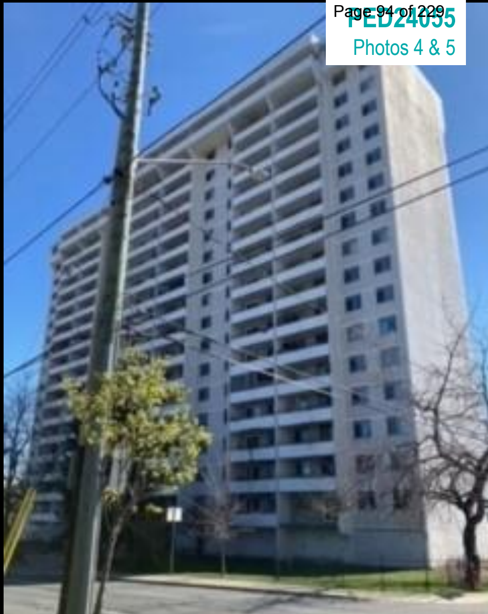
View From the Site Looking at the West Side of Queen Street South 2
