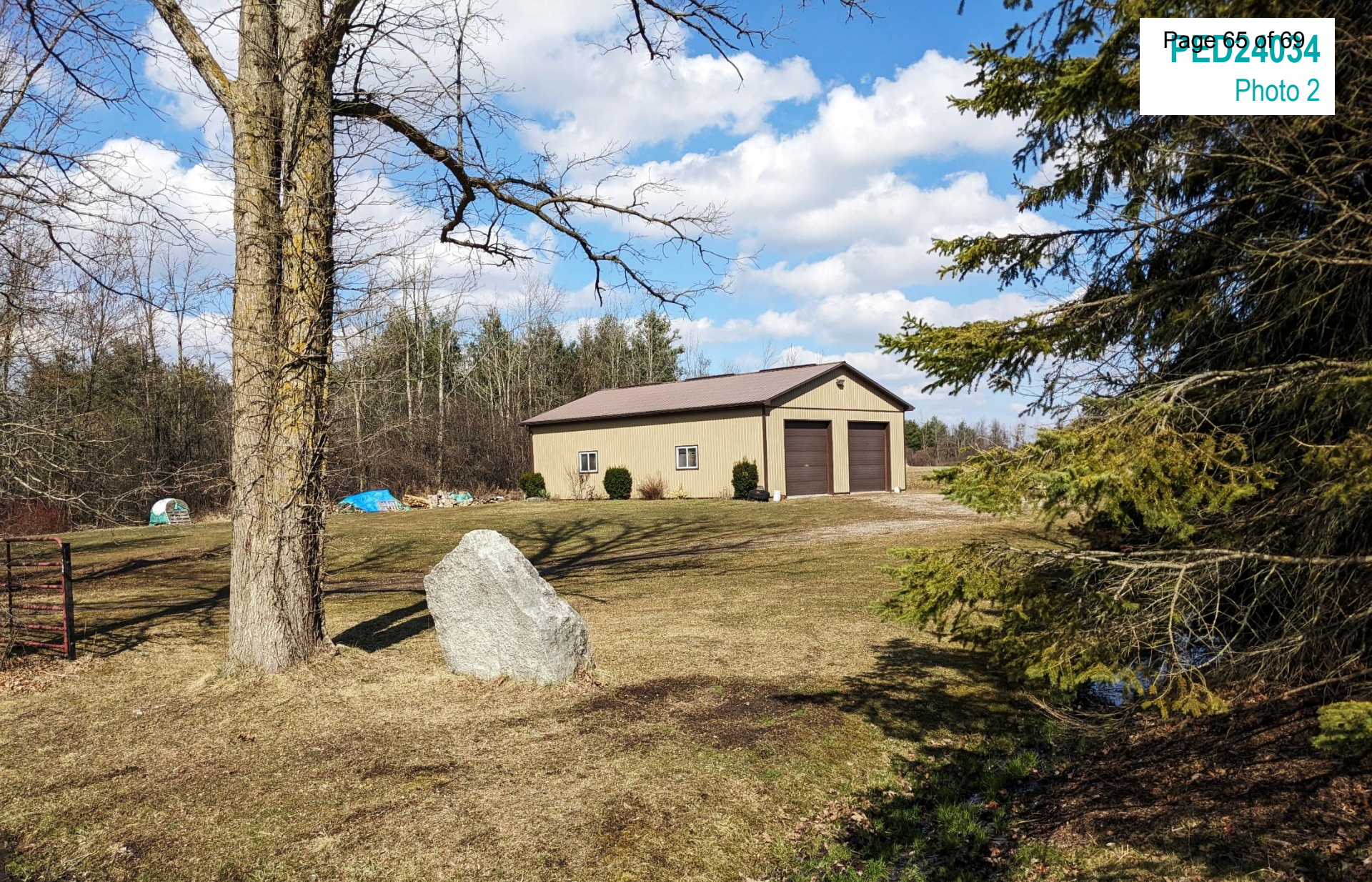
Existing accessory structure on farm parcel.
