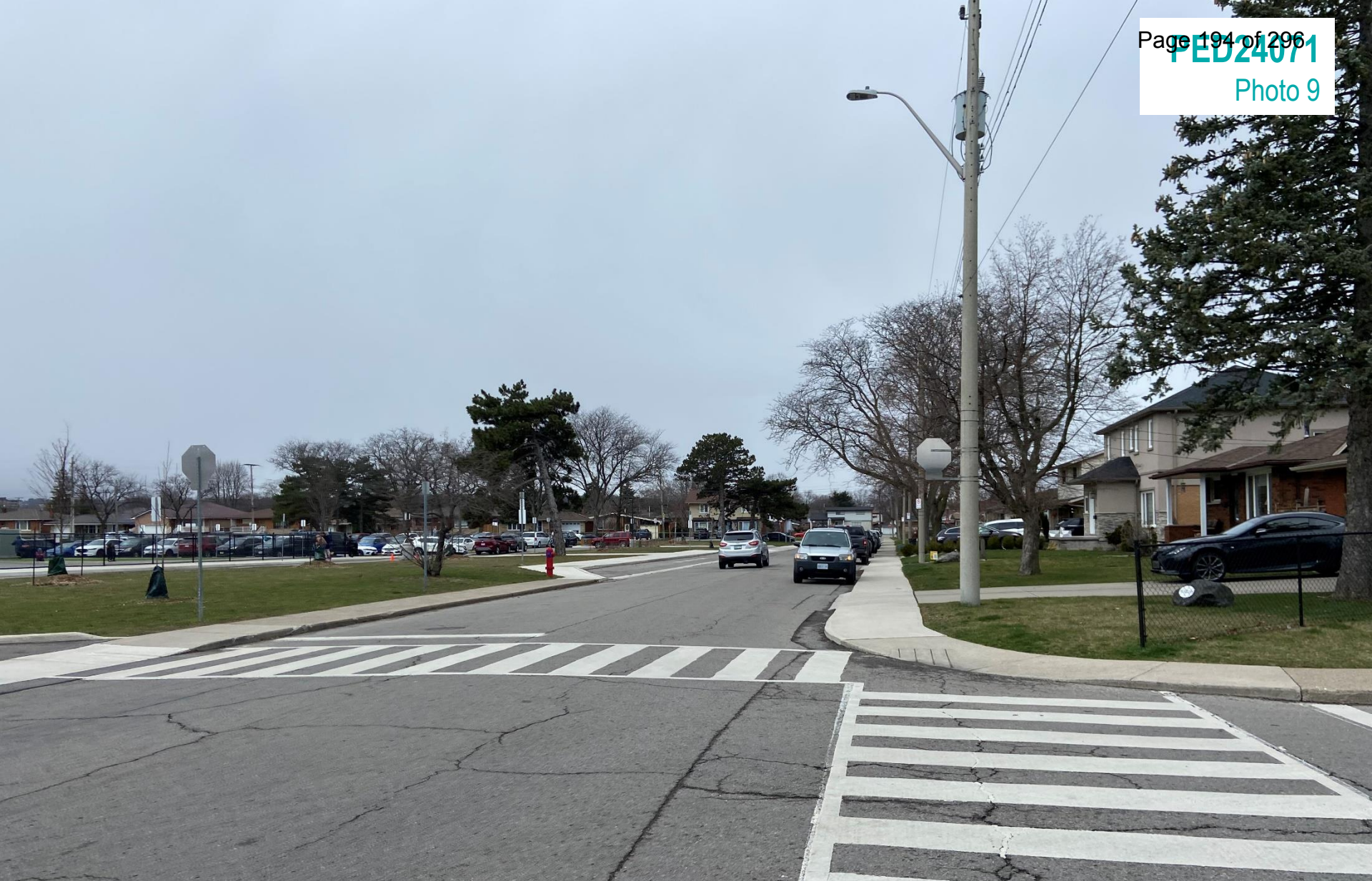
Second Drive looking west
