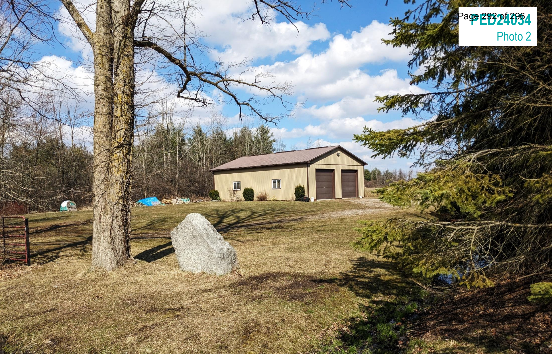
Existing accessory structure on farm parcel.
